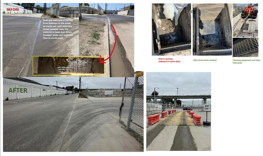
Sediment cleared, and sediment tracking controls installed at truck exit
