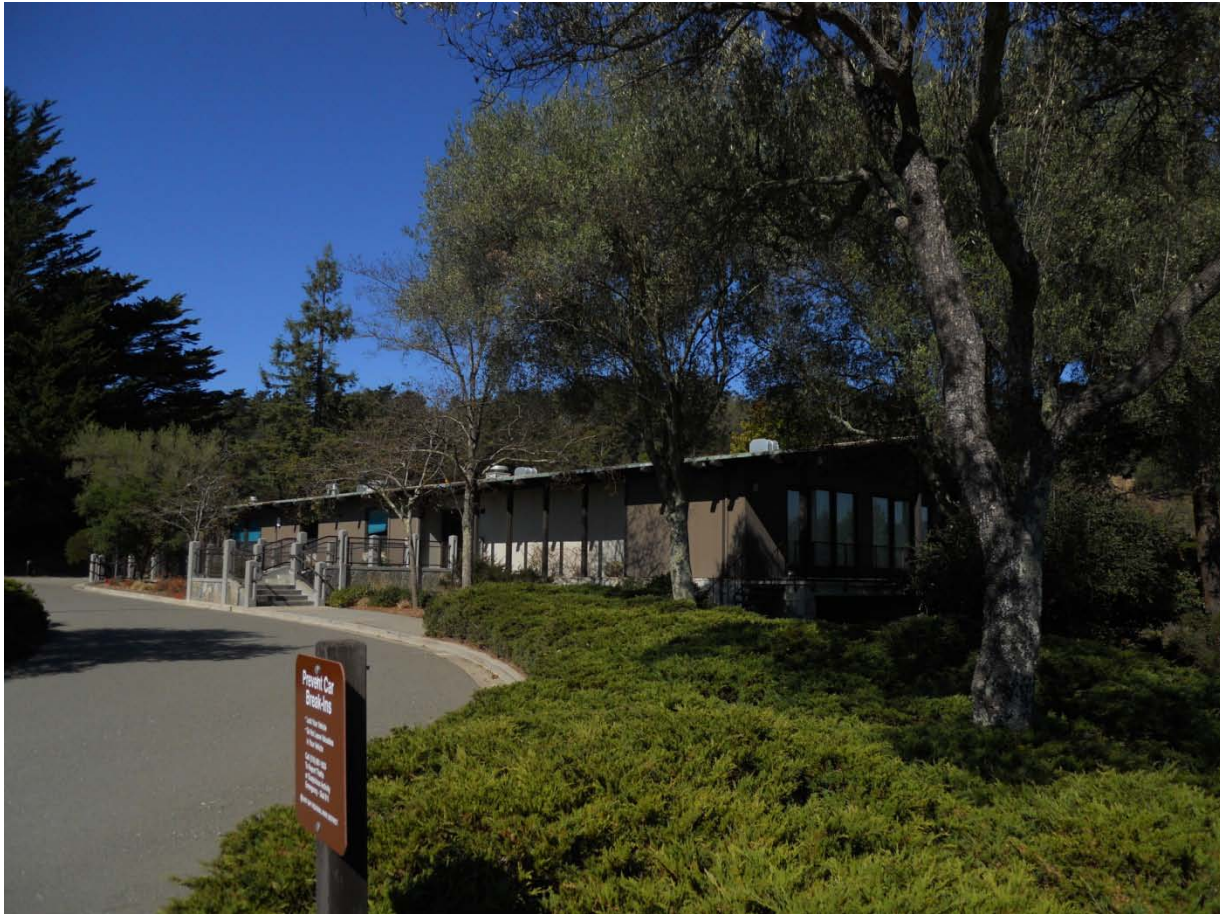
11500 Skyline Boulevard - Richard C. Trudeau Training Center Southwest Oblique
