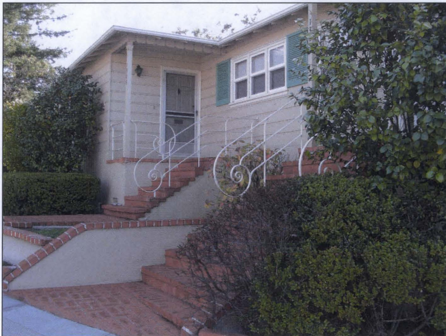
Photograph 3, detail of stairs and railing. Camera facing southeast. December 26, 2007.
