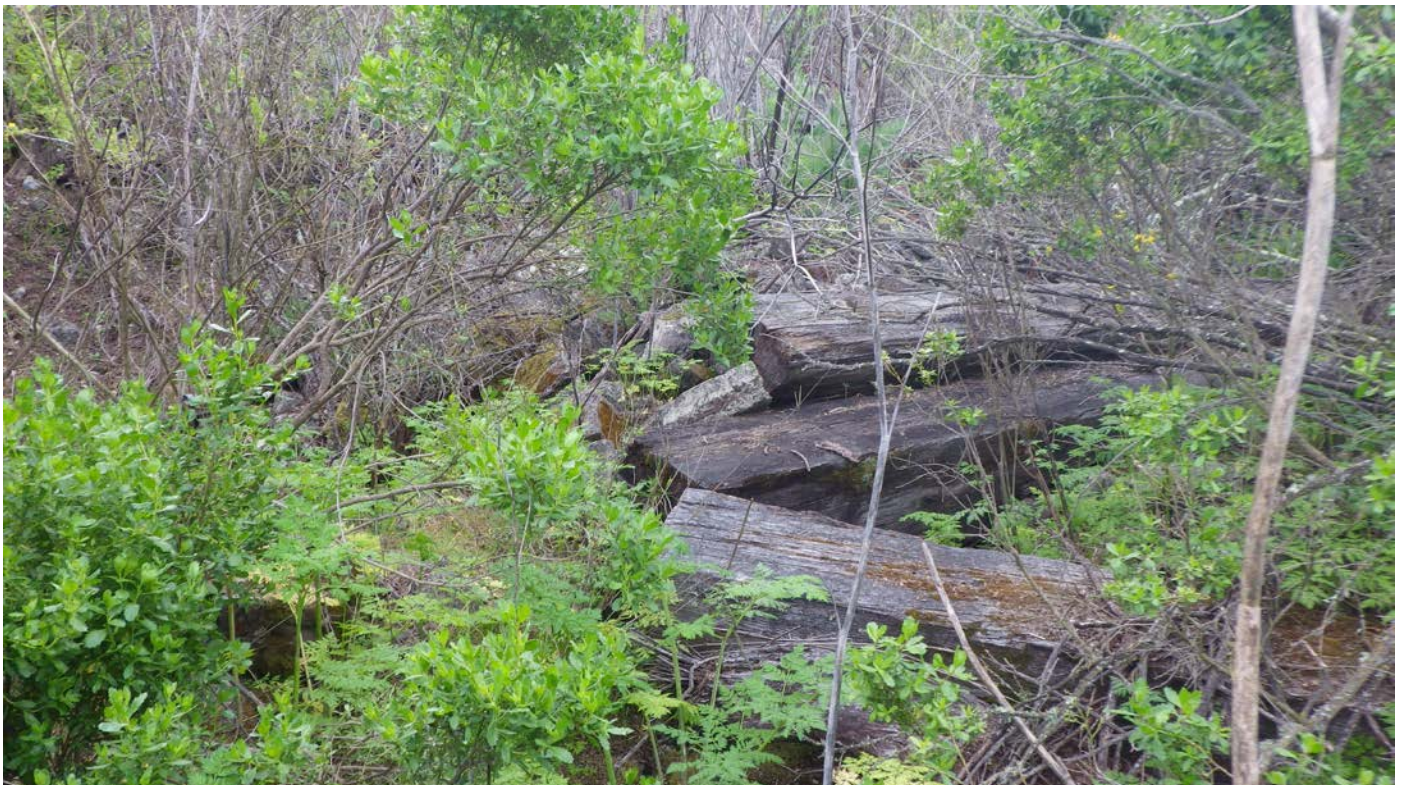
Site S6. Pile of large wooden beams 12x18 in. and concrete debris within the center of the mapped site. View to the south.
