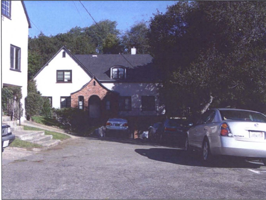
Photograph 2, north building. Camera facing north.
