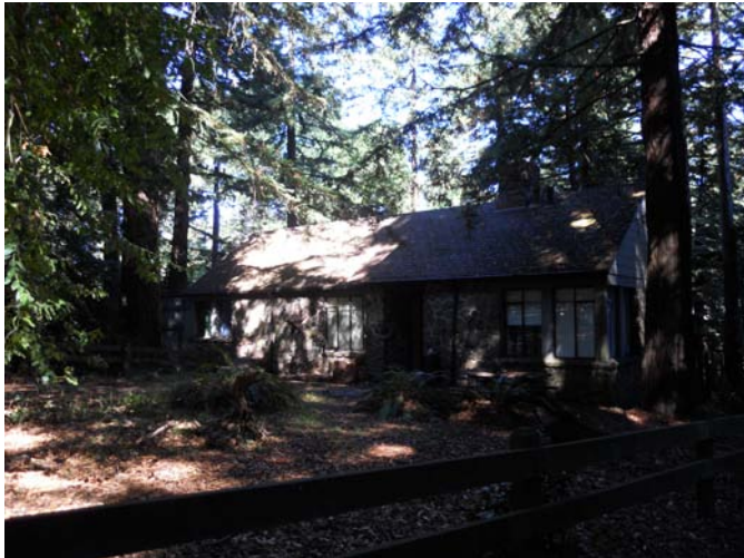
Residence in front of Redwood Bowmen Archery Range West Elevation
