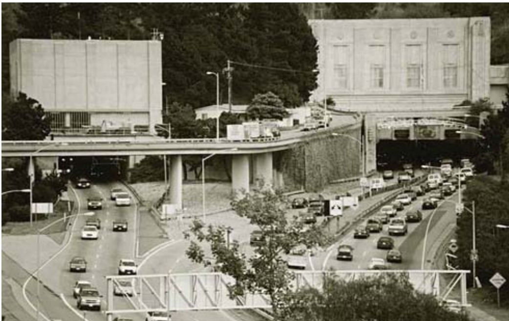
View of the western portals for Bore 1 (far right), Bore 2 (adjacent to Bore 1), and Bore 3 (left), from http://www.mtc.ca.gov/library/caldecott/ date unknown.
