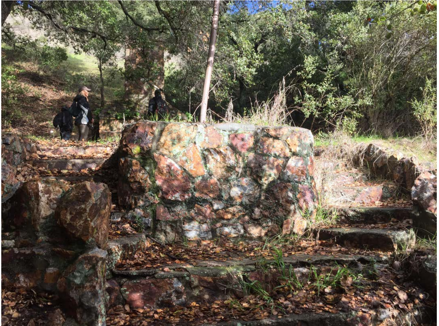
Site 7 (Feature F8 and F8a). Feature F8 is the steps and F8a is the flagpole and plinth. At the landing, the steps divide into two curvilinear sets of steps up to the meeting landing (Feature F4). The top, center rock is incised "1936," see next figure for detail.
