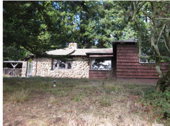
8500 Skyline Boulevard South Elevation
