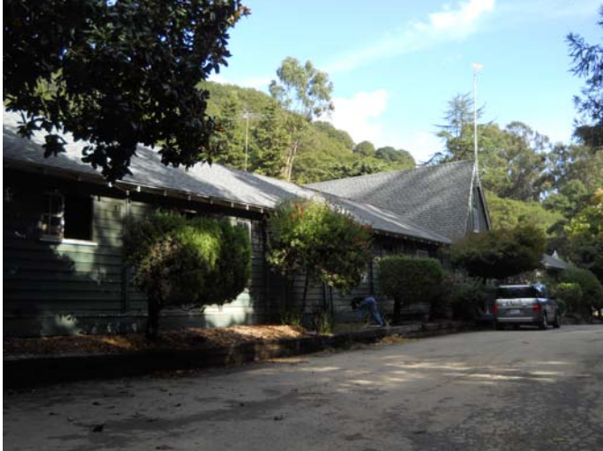
Piedmont Stables South Elevation (Front Façade)
