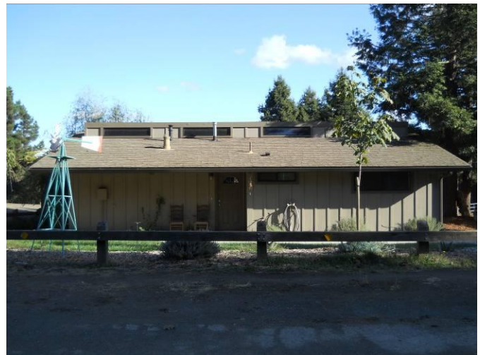
Chabot Equestrian Center Original Residence North Elevation
