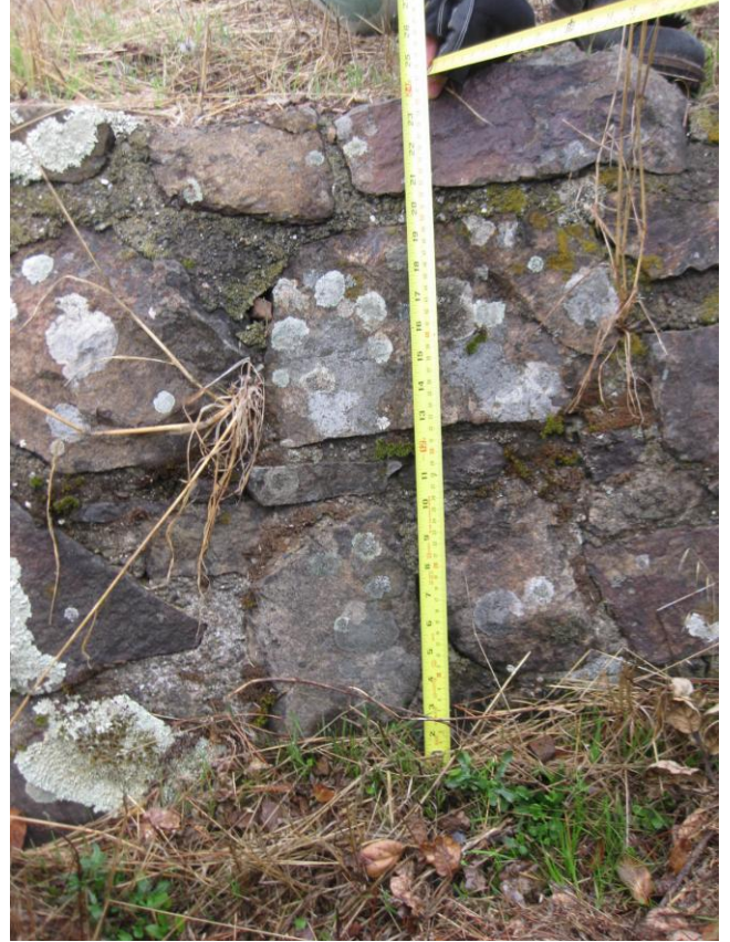
Photo #22 of cross section view to the north.
