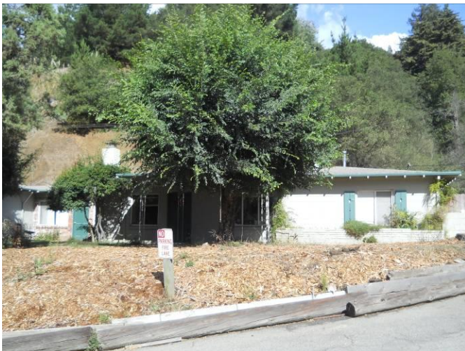
Skyline Ranch East Residence north elevation
