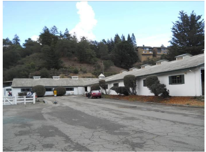
Skyline Ranch north elevation
