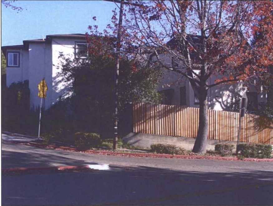
Photograph 4, west and south buildings. Camera facing northeast.
