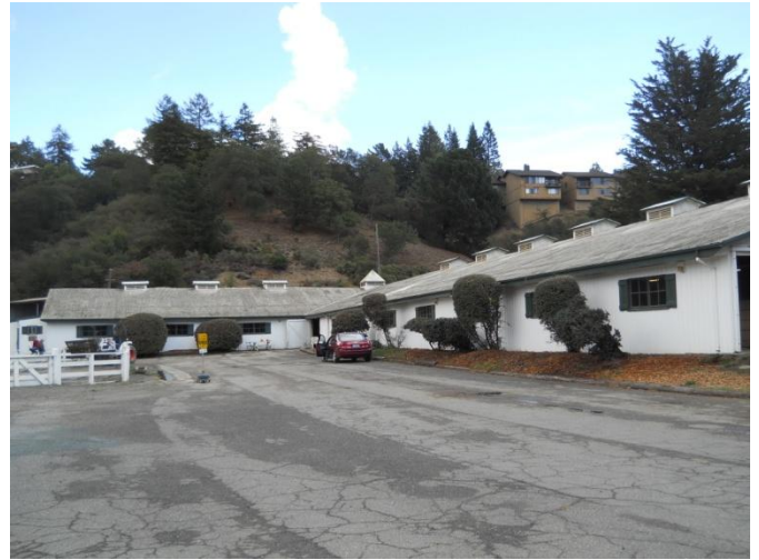
Skyline Ranch north elevation
