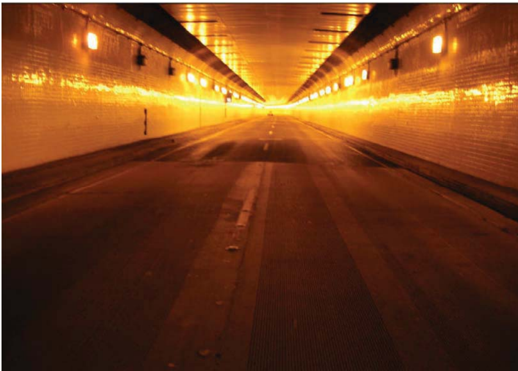
View looking east between Call Boxes 9 and 10, October 5, 2009.
