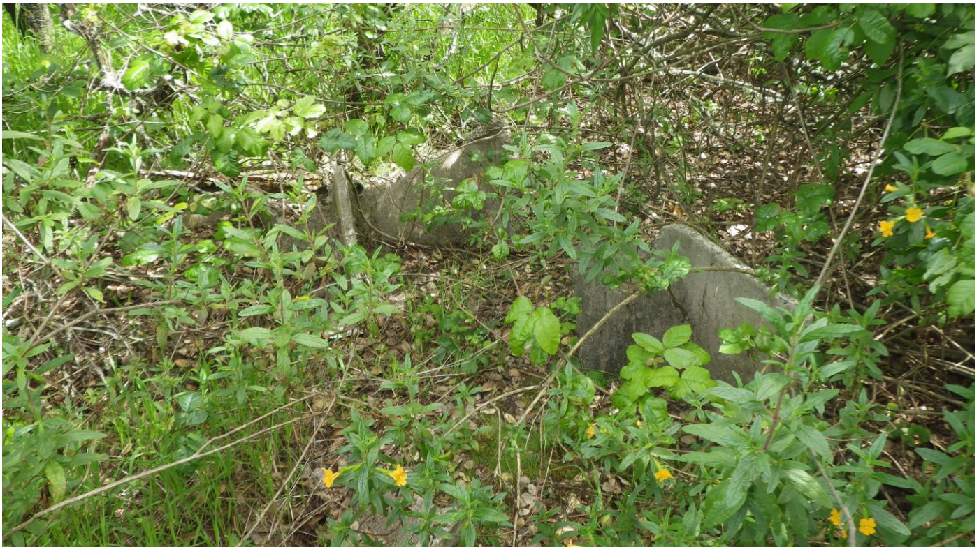
Site S1. Formed concrete and embedded hardware.
