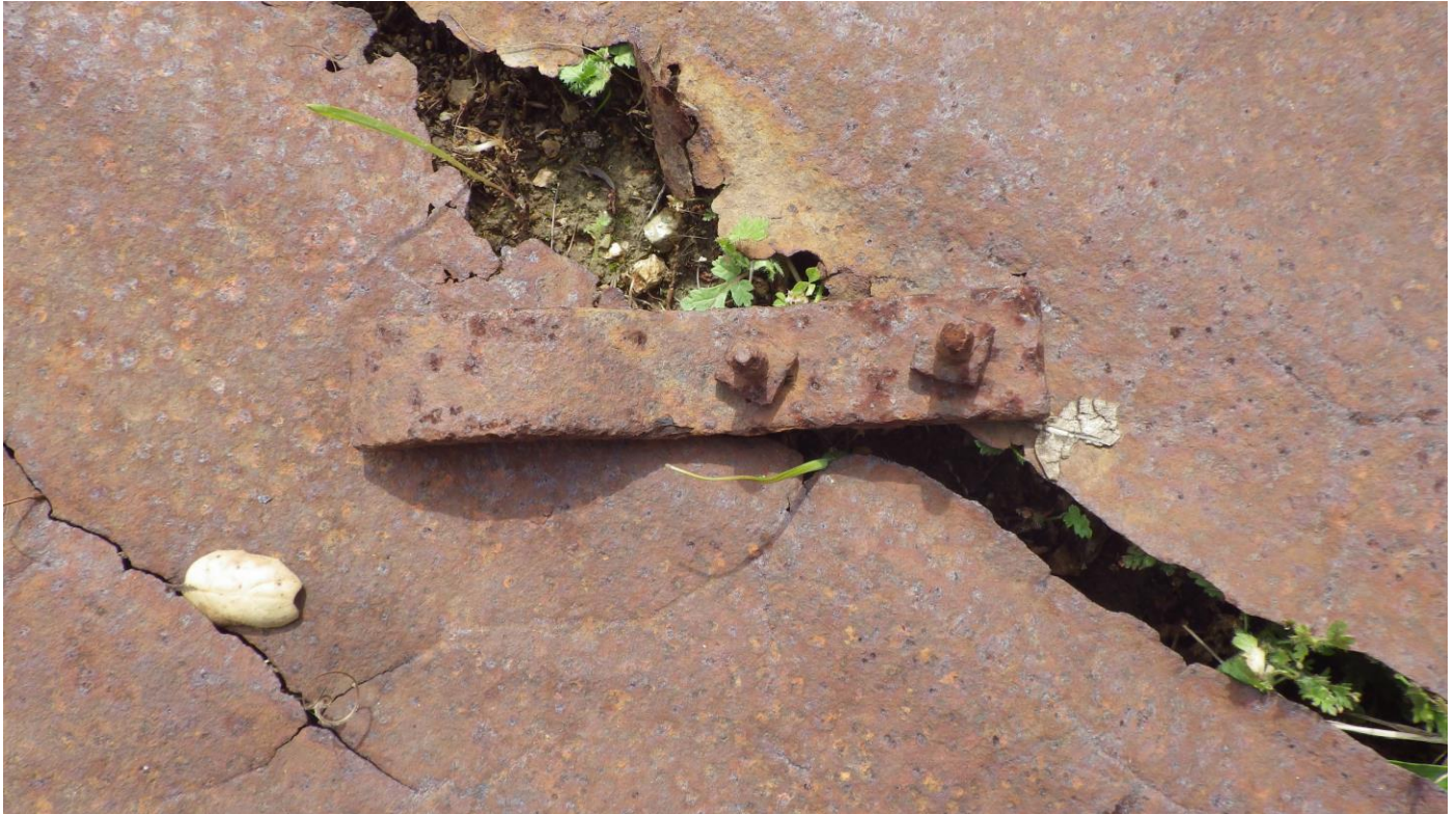
Site S1. Hardware attached to sheet metal (square bolts 7/16 in.).
