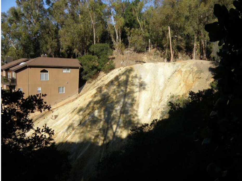
Lower tailings. View to Northwest.
