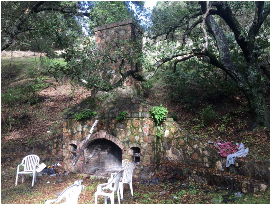
Site 7. Overview of WPA-constructed chimney with hearth, side grill niches, and bench/retaining wall wings. View to the north.
