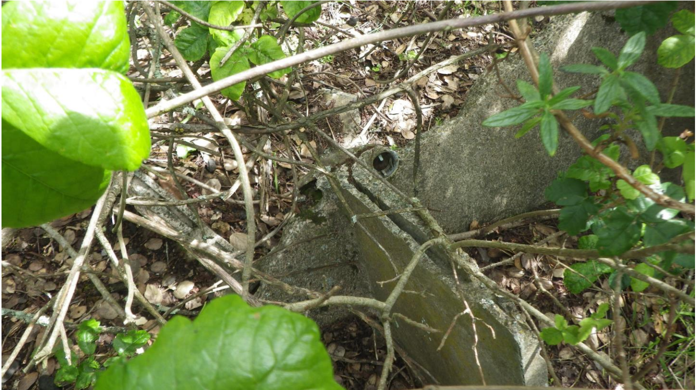
Site S1. Formed concrete and embedded hardware.
