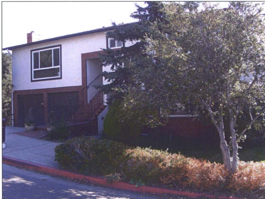
Photograph 3, west building. Camera facing east.
