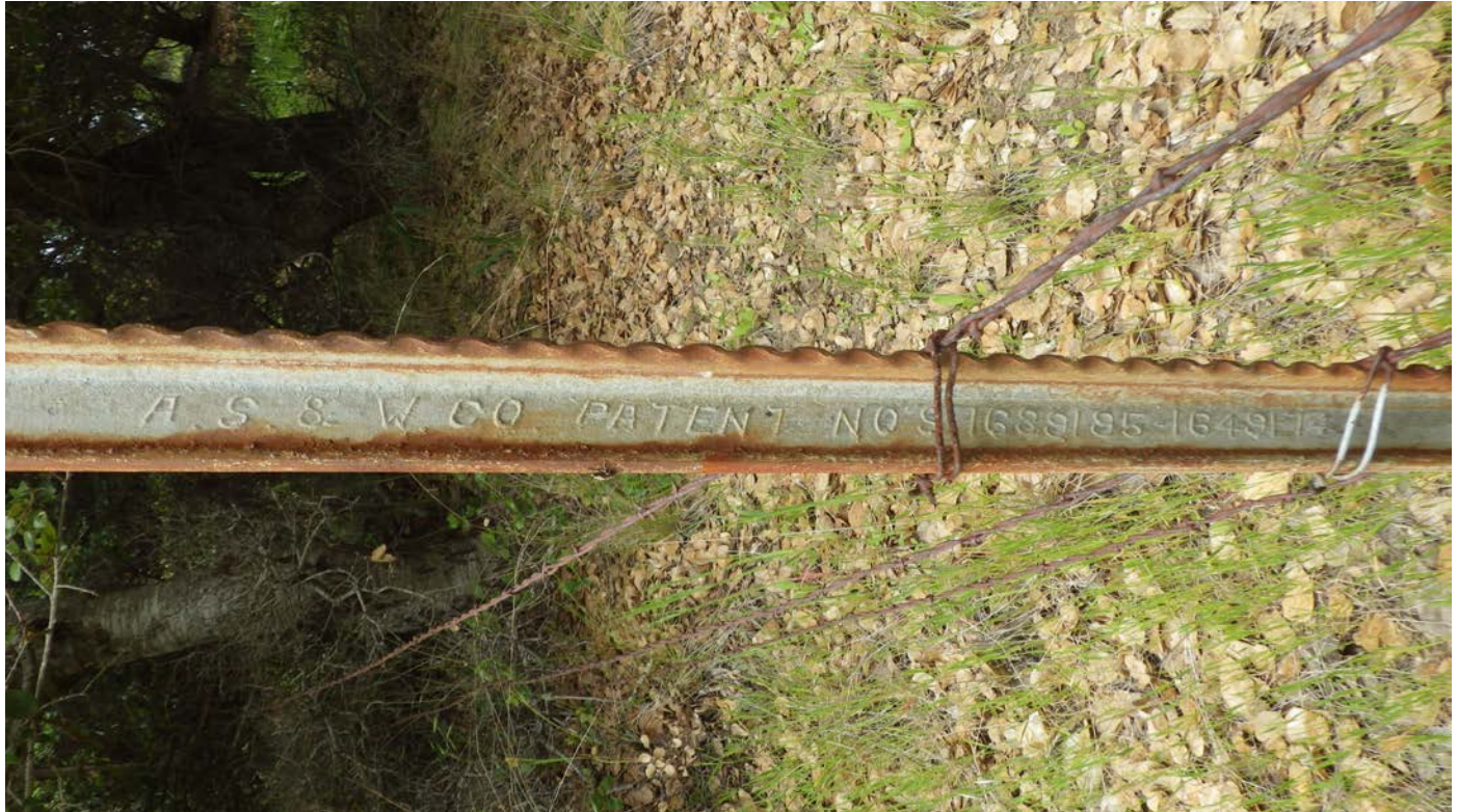
Resource S4. Detail of manufacture information on golf course boundary t-bar fence post (southern mapped section).
