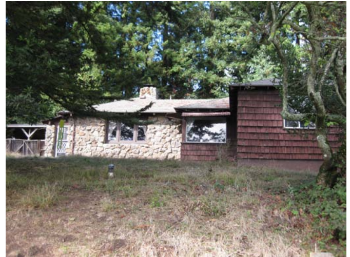
8500 Skyline Boulevard South Elevation
