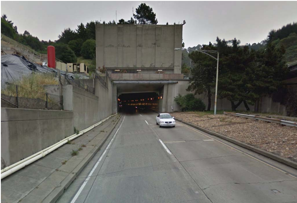
View of the western portal looking east, May 2011.
