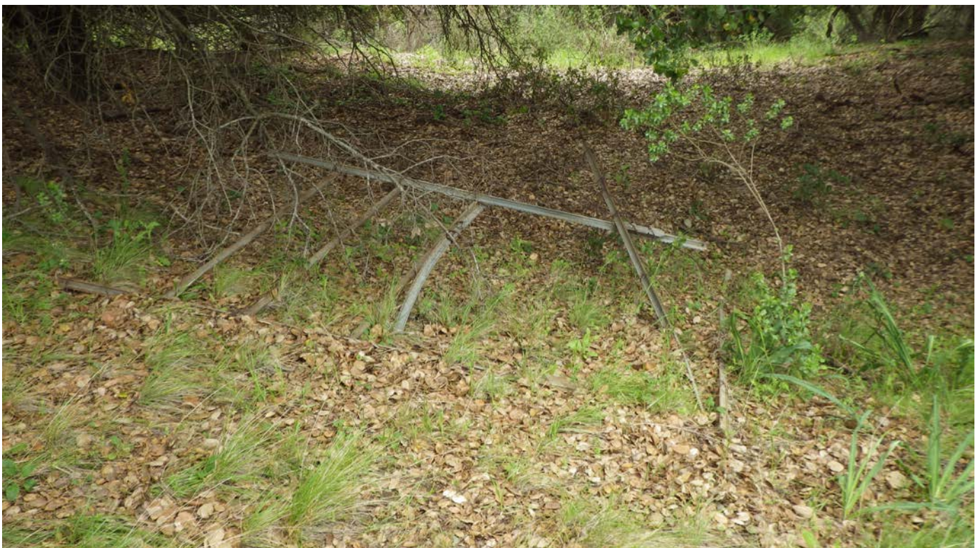
Resource S4. Downed gate near corner post made from t-bar posts (southern mapped section).
