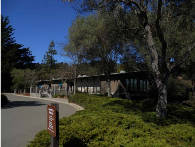
Richard C. Trudeau Training Center Southwest Oblique
