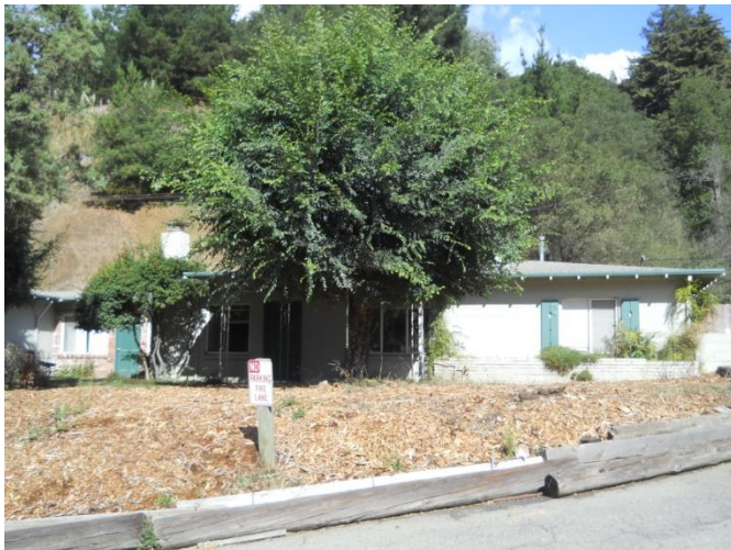
Skyline Ranch East Residence north elevation
