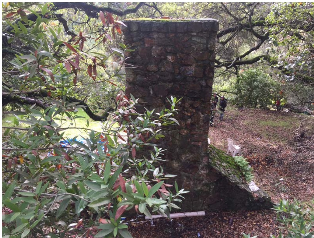
Site 7. Rear view of the chimney, note the step gradient and use of the chimney and wings to form a retaining wall and create a flat platform for meeting in front of the chimney. View to the south.
