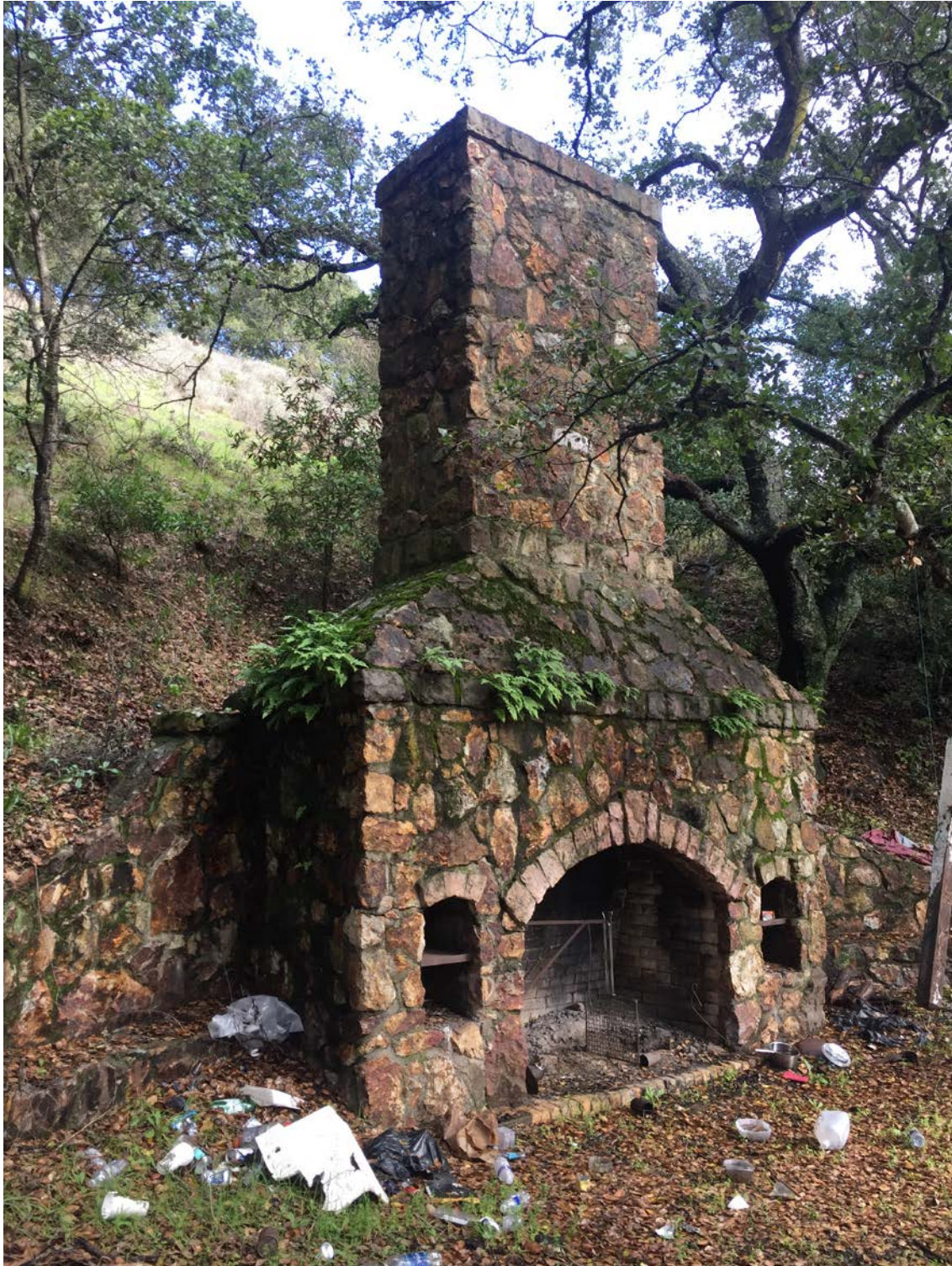
Site 7. The rock-and-mortar chimney includes architectural design features including voussoir-set stones with tripartite keystone over the hearth, square-set rock courses at the top of the hearth and base of chimney flue, and on chimney cap. View to the northeast.
