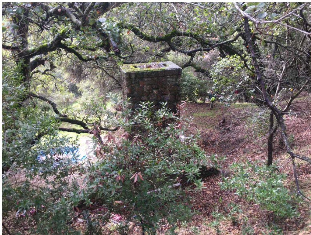
Site 7. Overview of chimney from uphill, rear, note three chimney flues for central hearth and two side grill niches. View to the south.
