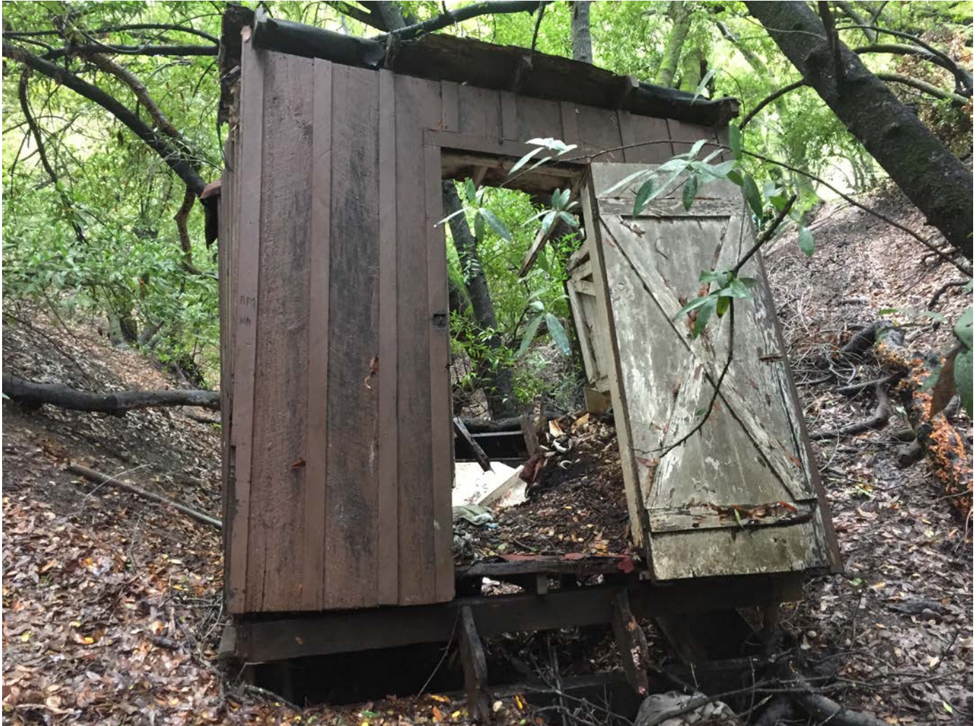
Site 7 (Feature F17a). The latrine walls are single-board thick. The door is made of vertical boards with styles and diagonal cross boards and set on the north façade above two steps, step rails remain (bottom center of photograph). Toilet, sink, toilet paper dispenser, and erosion debris are within the latrine. View to the south.
