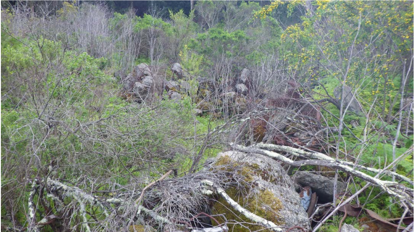
Site S6. Extensive piles debris including concrete, rebar, and galvanized pipe with chain (gate post) from the central portion of the mapped site. View to the south.
