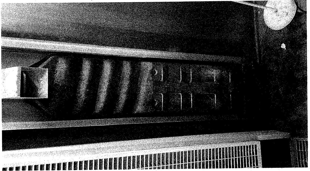
Exhibit 3, picture of heater taken 4/11/2018, removal of parts.
