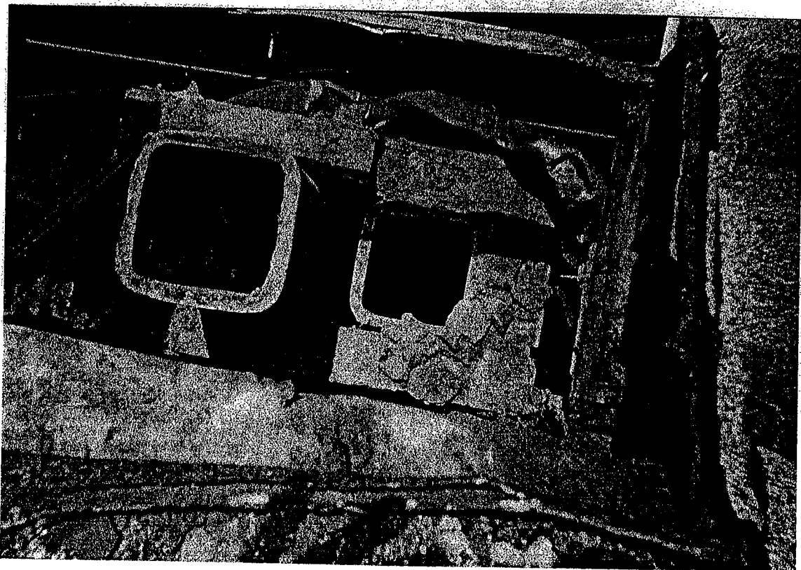
Photograph 8 depicts aerial view of chimney showing broken chimney at roof line.
