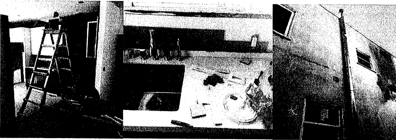
Gen. Contractor hanging new cabinets, new kitchen backsplash tiles, sink, faucet, countertop, new furnace exhaust.
