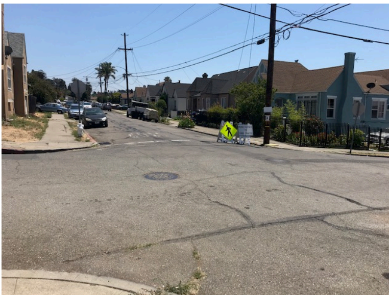
Figure 9: Northeast Corner at Ney Avenue and 76 th Avenue
