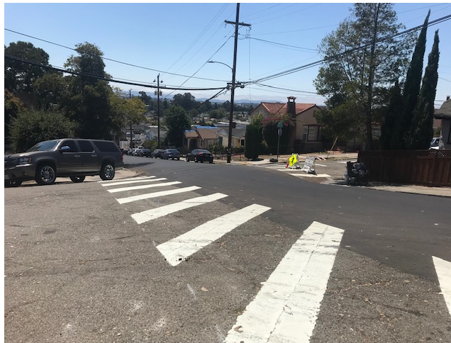
Figure 15: Continental Marked Crosswalk a Northwest Corner at Ney Avenue and Partridge Avenue
