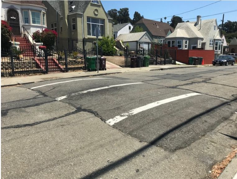
Figure 8: Speed Hump on Ney Avenue Between 75 th Avenue and 76 th Avenue
