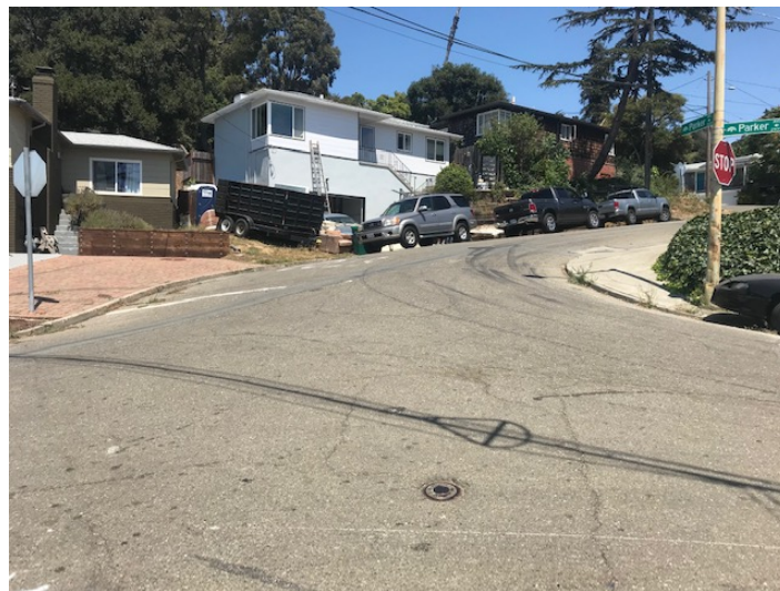
Figure 27: Northwest Corner at Parker Avenue and Outlook Avenue West
