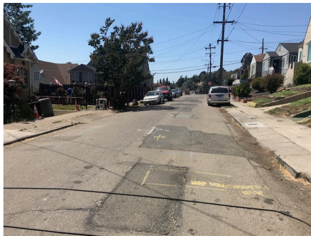
Figure 18: Outlook Avenue Between 75 th Avenue and 76 th Avenue Looking Northbound
