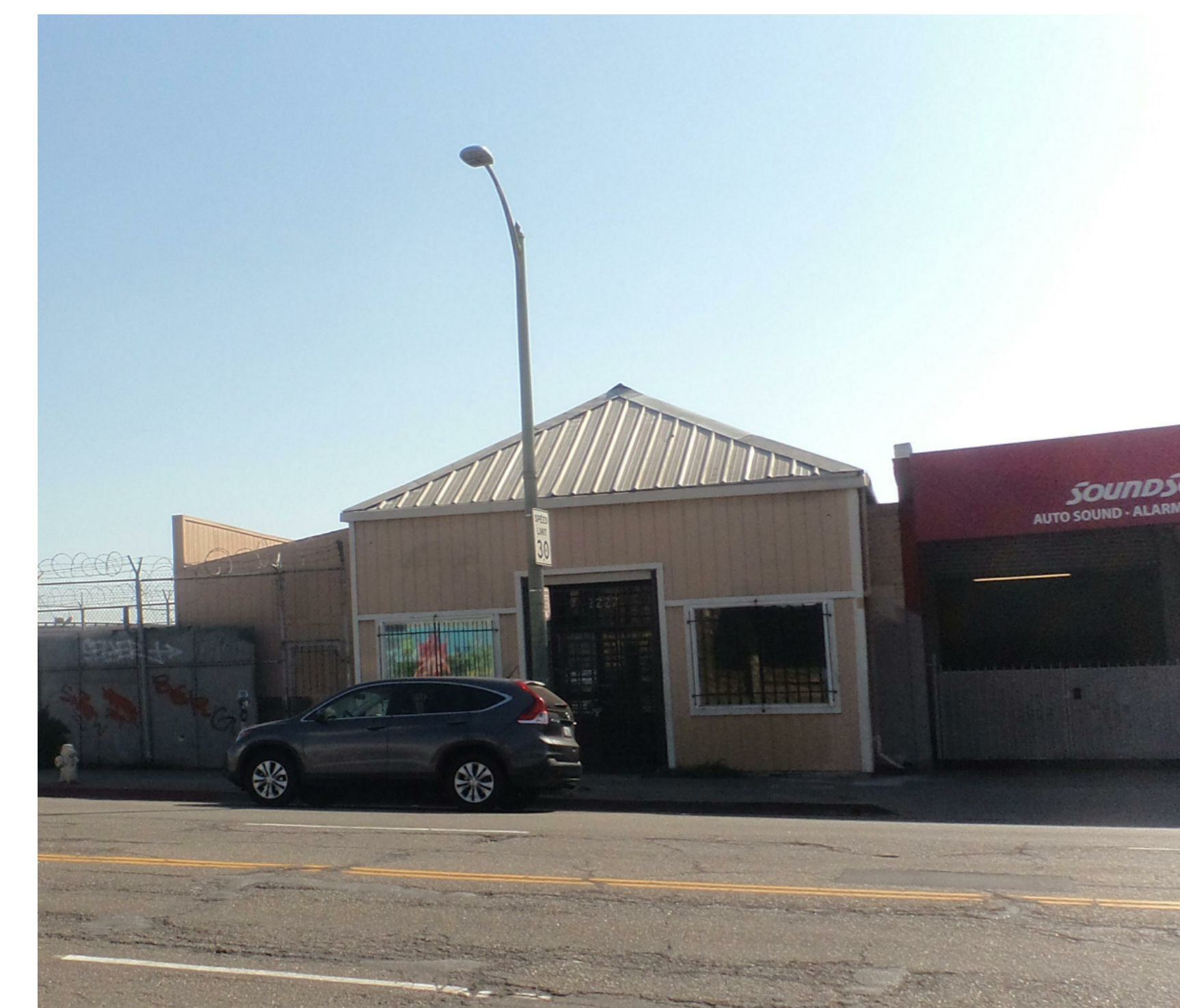
2227 INTERNATIONAL BOULEVARD (EXISTING SITE)
