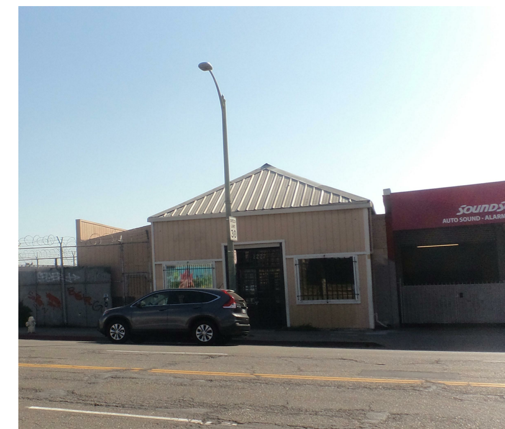
2227 INTERNATIONAL BOULEVARD (EXISTING SITE)
