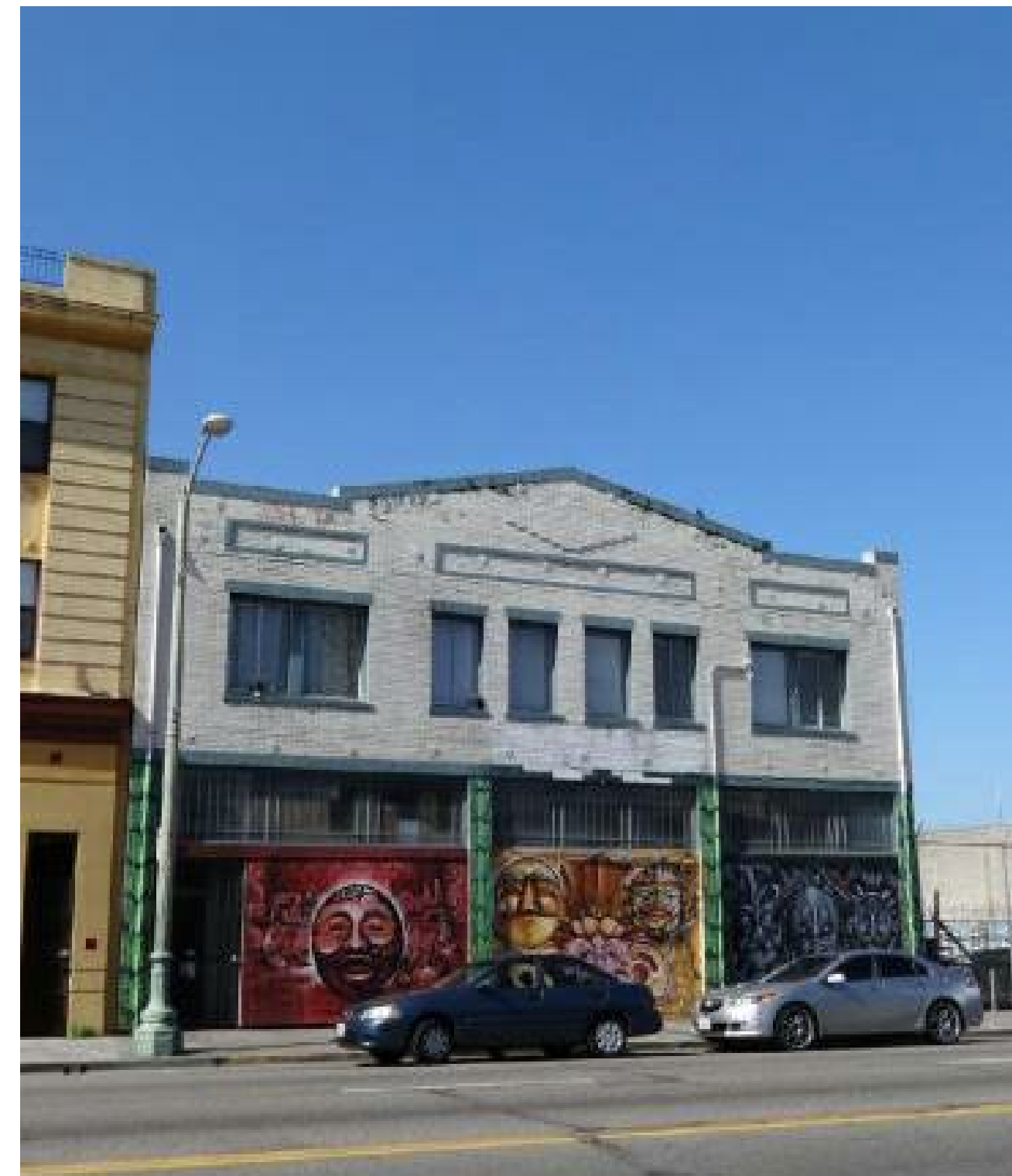
2257 INTERNATIONAL BOULEVARD (EXISTING SITE)
