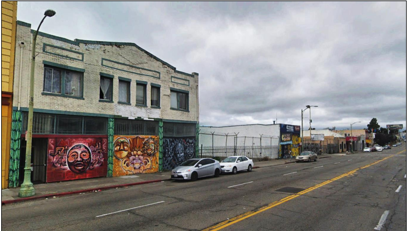
Figure 2 Project Site looking West; 2257 International Blvd. to be demolished
