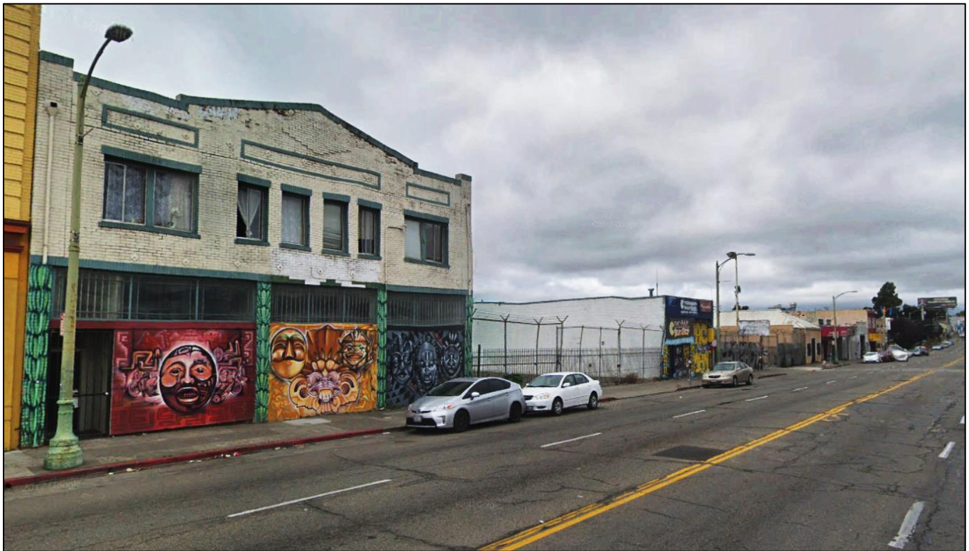
Figure 11 Project Site looking West; 2257 International Blvd. to be demolished
