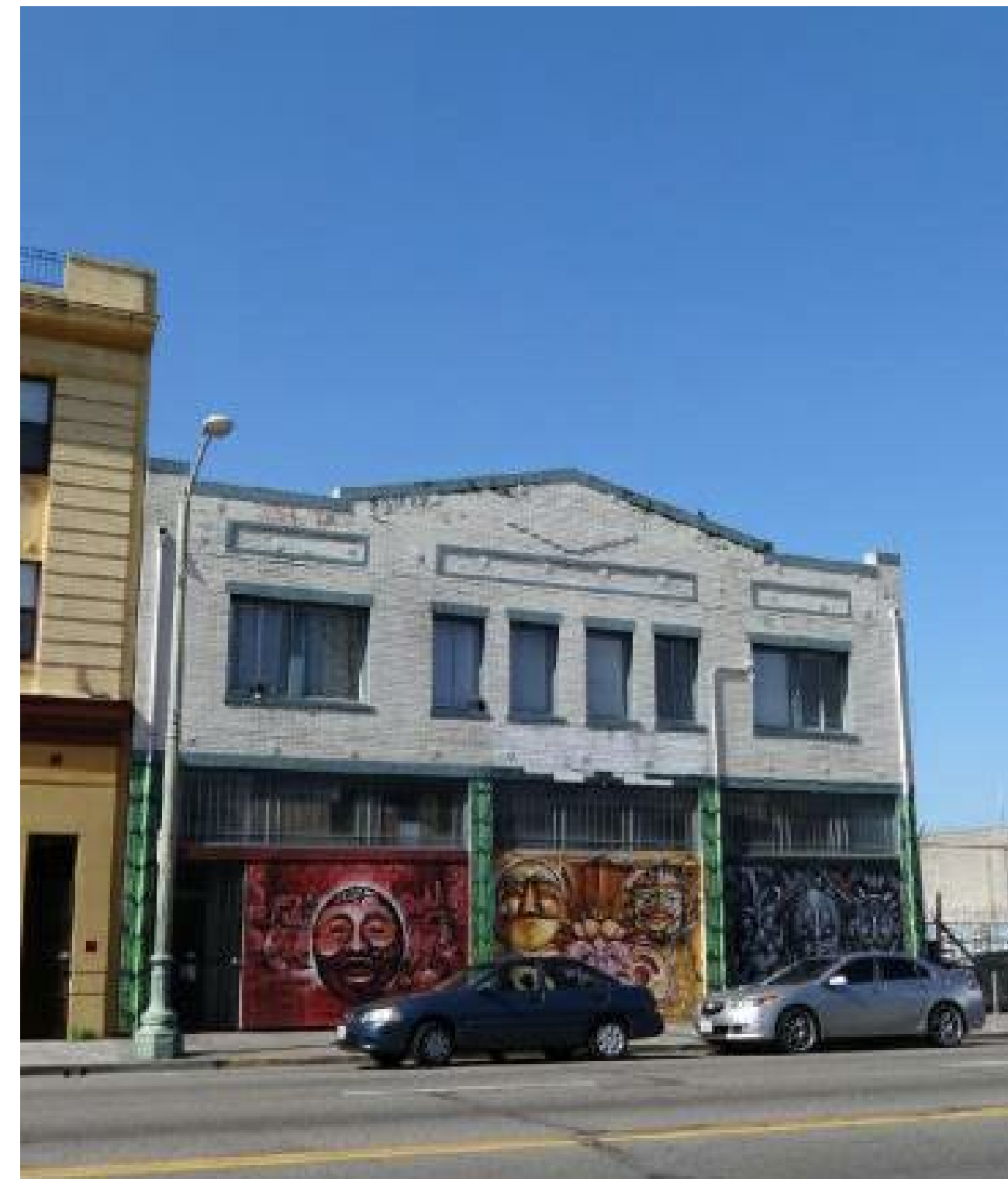
2257 INTERNATIONAL BOULEVARD (EXISTING SITE)
