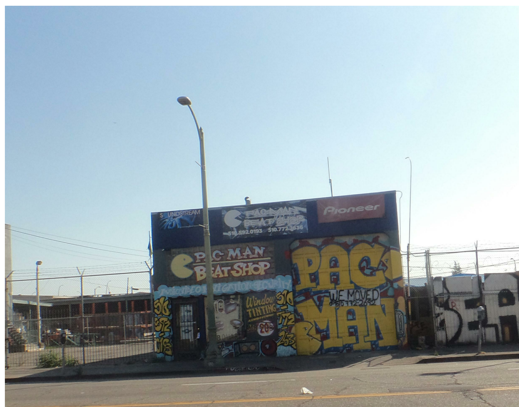
2245 INTERNATIONAL BOULEVARD (EXISTING SITE)
