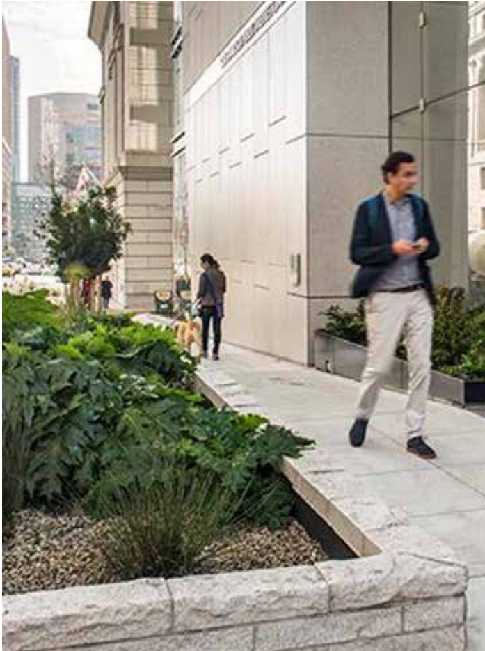
LIVING MACHINE BLACKWATER TREATMENT AT THE SAN FRANCISCO PUBLIC UTILITIES COMMISSION HEADQUARTERS, SAN FRANCISCO, CA.
