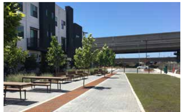
COMBINING MATERIALS TO CREATE STRIPES FRAMED BY CONCRETE BORDERS
