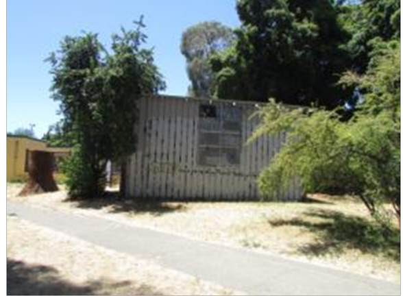
The Mosswood Park stage workshop. Knapp Architects photo, 2020
