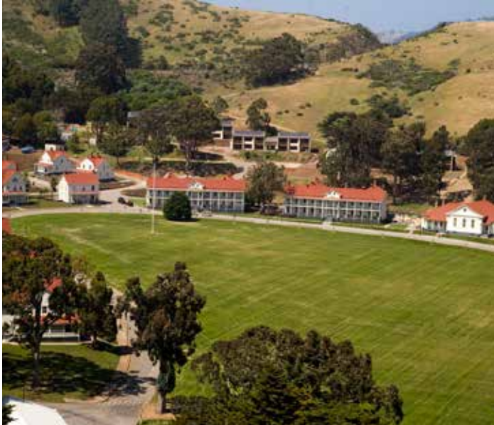
THE TRANSFORMATION OF FORT BAKER TO CAVALLO POINT LODGE IN SAUSALITO, CA POWERFULLY DEMONSTRATES THE INTER-RELATIONSHIP BETWEEN PRESERVATION AND SUSTAINABLE DESIGN.
