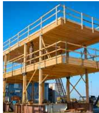
3 MASS TIMBER STRUCTURE
