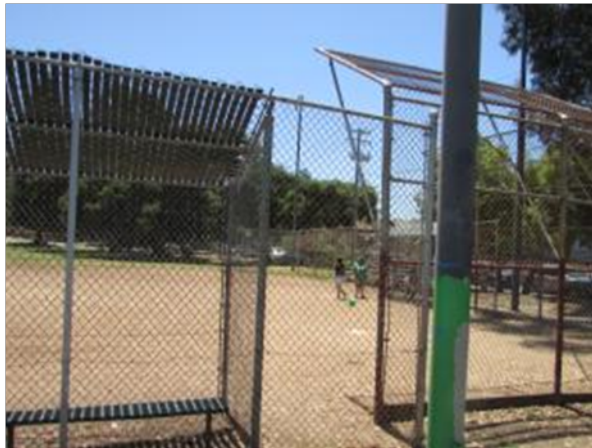
The Mosswood Park Baseball Field. Home Plate is in view. Knapp Architects photo, 2020
