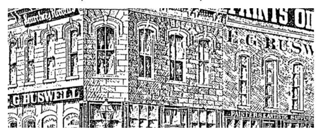
**9.Year:** 2022 **Cost:** \$5K **Improvement:** The *cornice brackets* portrayed in the historic illustrations will be fabricated and installed along both street sides. There were originally more than fifty of these brackets.
