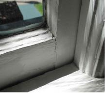
Samples of the many window frames whose wood is dried out, stained in places, with damaged paint.
