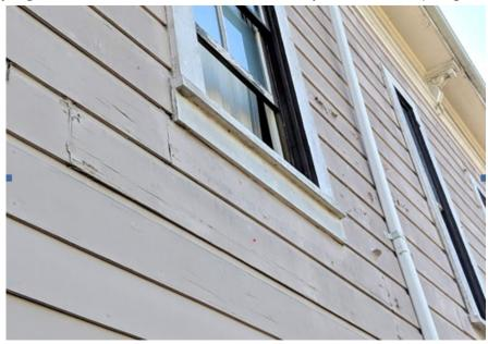
The paint is blistering and peeling, especially on the east (rear) and south (right) sides of the home.
