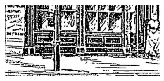
**5. Year:** 2021 **Cost:** \$5K **Improvement:** The original *cast iron columns* with floral detail revealed during careful demolition will be refurbished on the corner and along Broadway. The bases of these columns will be recreated with wood and stucco to match the historic design.
