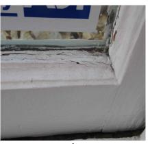
Some wood is dry-rotten but most damage is the result of aging putty, sun exposure and water seepage.
