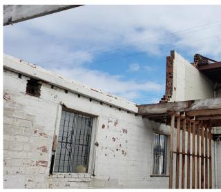
5.Add new metal coping at top of wall structure as well as liquid waterproofing over exterior and interior faces (open as a courtyard so both sides of the wall are fully open to the exterior elements) of terra-cotta walls in order to seal and waterproof all nooks and cranny's from the elements. (picture at top of parapet of 24th and 23rd prior to new construction.
