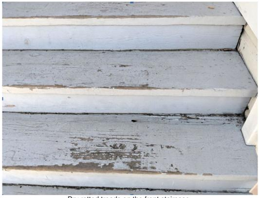
Dry rotted treads on the front staircase.
