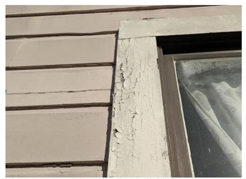
Many parts of the trim and some pieces of the hardwood siding also need to be replaced due to dry rot. Flat trim should be replaced with the historical molding.
