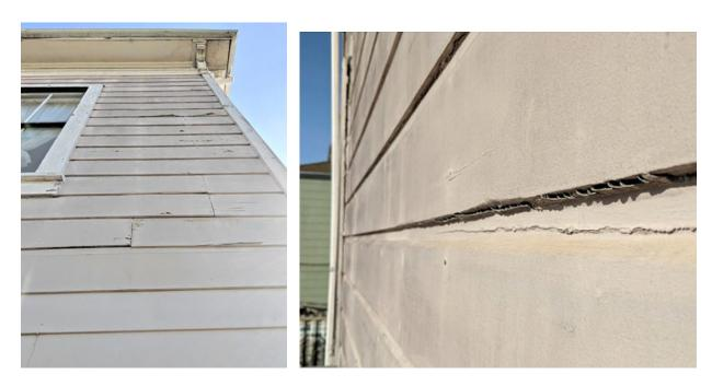
The finish nails are pushing out of the siding in many places and need to be reset (left). The caulking which was added to the bottom edges of all the siding boards needs to be scraped out as it is chipped and blistering, and should not have been placed there in the first place (right). The entire exterior of the house then needs to be re-primed and painted.
