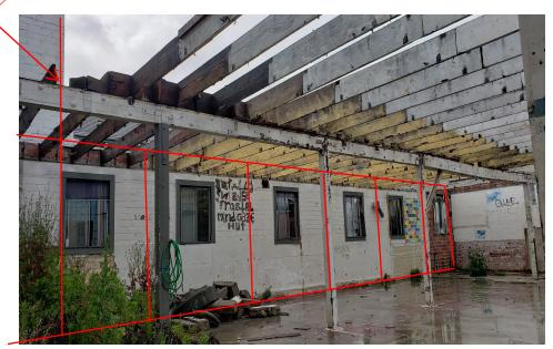
7.Repair damaged masonry work with masonry units to match original with cement Lime mortar to match existing. Provide chemical cleaning of masonry North and South Facades, with ProSoCO Sure Klean (or equivalent), then tuck pointing to take place after cleaning and repairing.
