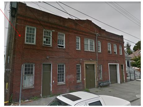
8.New coping and flashing over North and South Facades. Add flashing and waterproofing to integrate into the roof membrane at top of wall. Provide liquid waterproofing membrane over brick to seal and fill cracks and crannys at both the exterior and interior of the existing brick walls.
