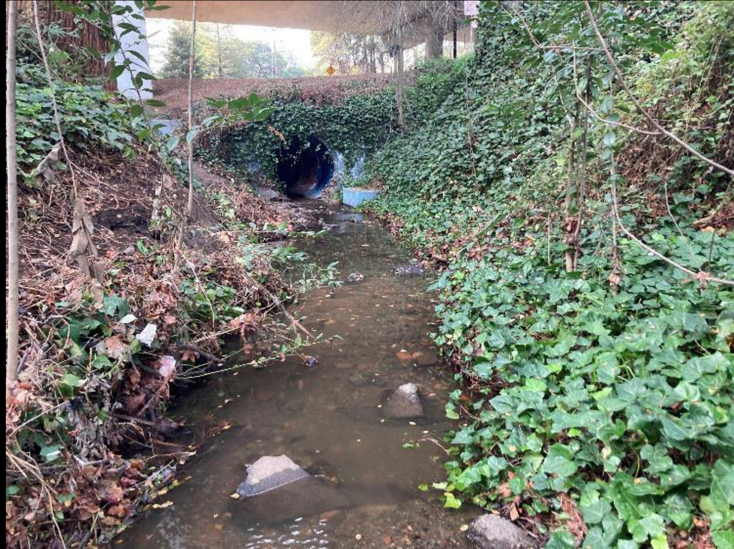
Pre-project conditions downstream of HWY 580. Natural channel with invasive ivy and native overstory vegetation.
