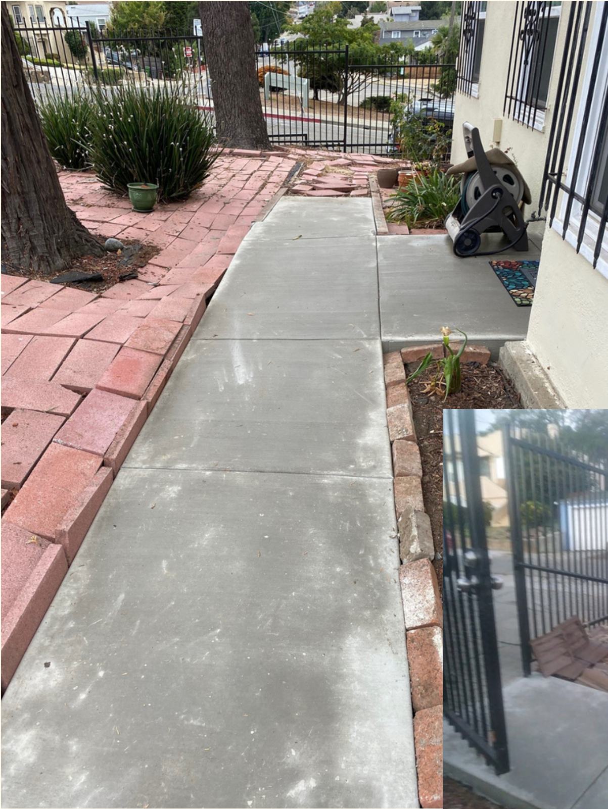
Access Improvement - AFTER
