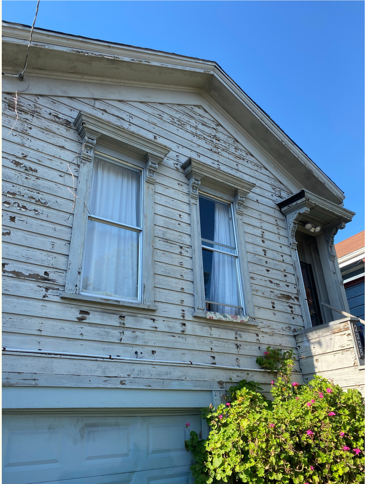
Lead Safe Homes project - BEFORE
