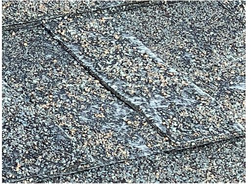
Closeup of shingle detail shows the material worn down to the fibers. Work Program Year 1(cont.): More evidence of fibers showing from beneath the missing asphalt granules.
