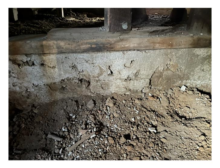
Work Program Year 4: Evidence of pest infestation in foundation framing and floor joists.
