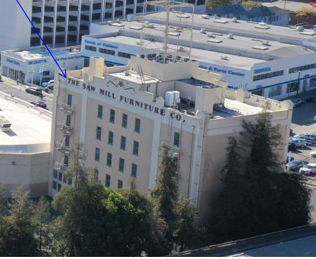
Year #7: Remove the existing metal coping cap (of the water proofing system) and install a new metal coping atop of the parapet walls, of North East South and West exterior walls, as well as liquid waterproofing over exterior. Add flashing & integrate into the new roof membrane at top of parapet.
