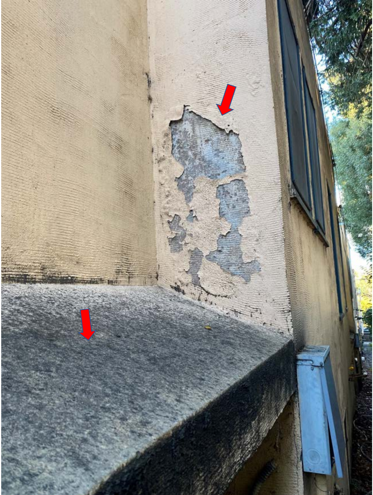
(Stucco repair on bungalow)
