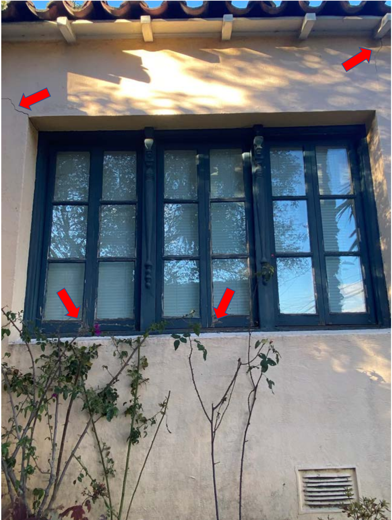
(Stucco cracking)
