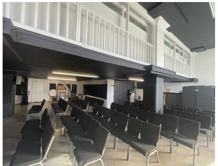
Ground floor space along the building's Broadway-frontage
