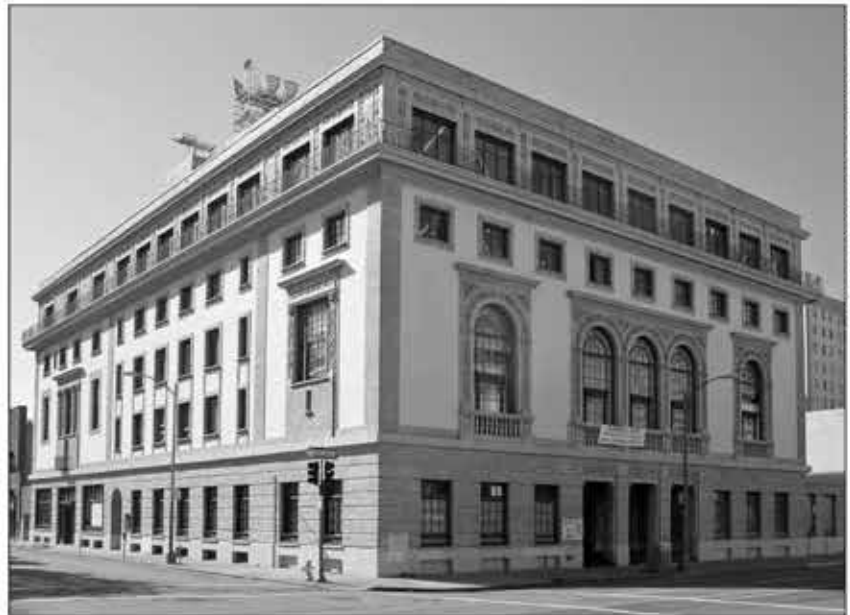
THE YWCA BUILDING , built by Julia Morgan, provides an early example of color used on a ceramic façade. It's also a good example of the use of a matte glaze finish.
