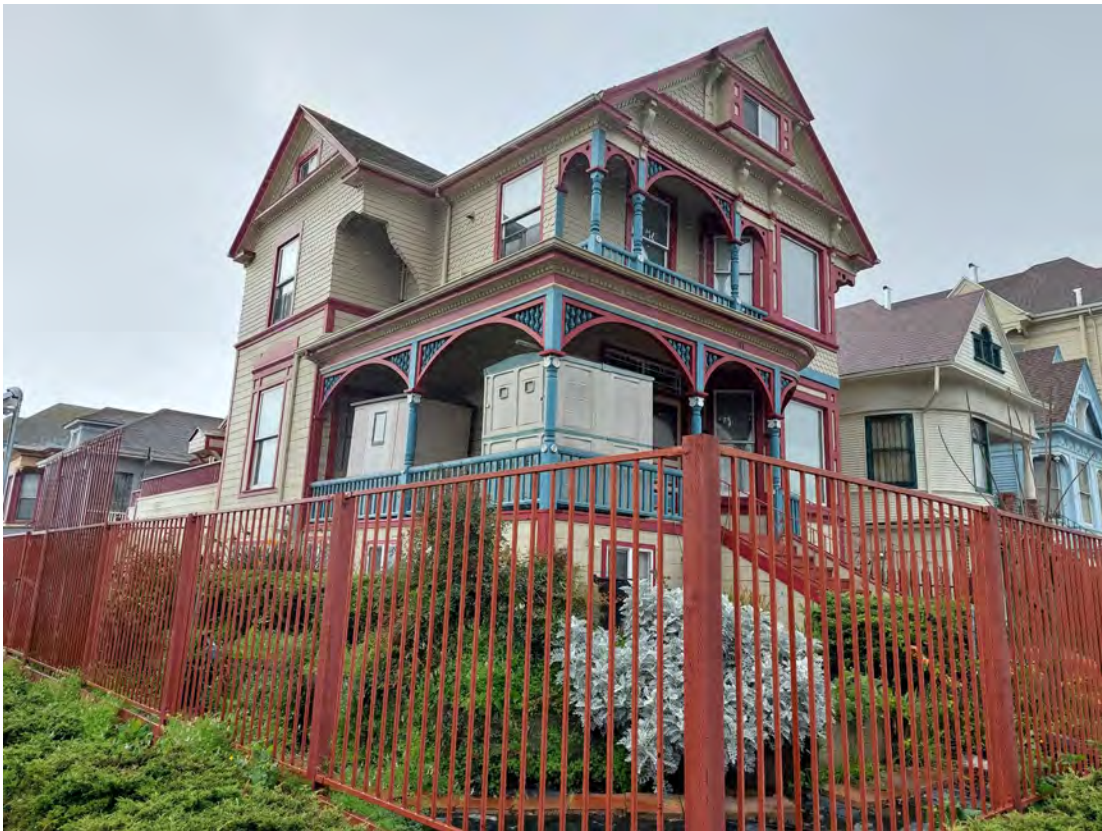
Photograph 4: Lougee-Baumgartner House at 51 8th Street (MR 05)
