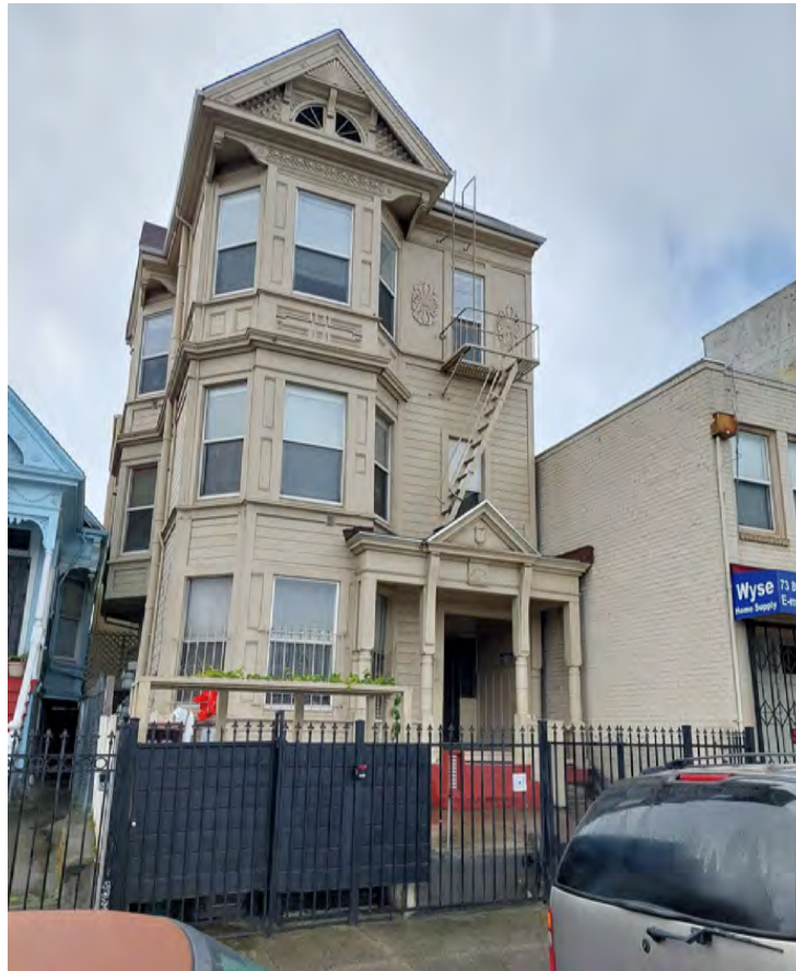
Photograph 7: Josephs House at 61 8th Street (MR 08)
