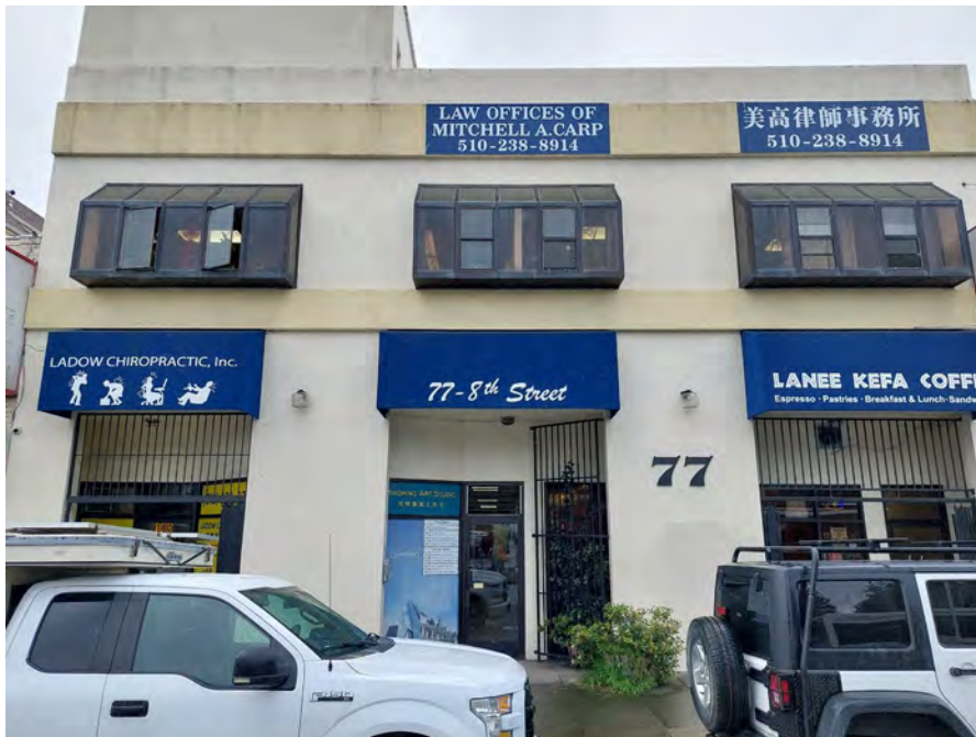
Photograph 2. 77 8 th Street, camera facing south, February 29, 2024.
