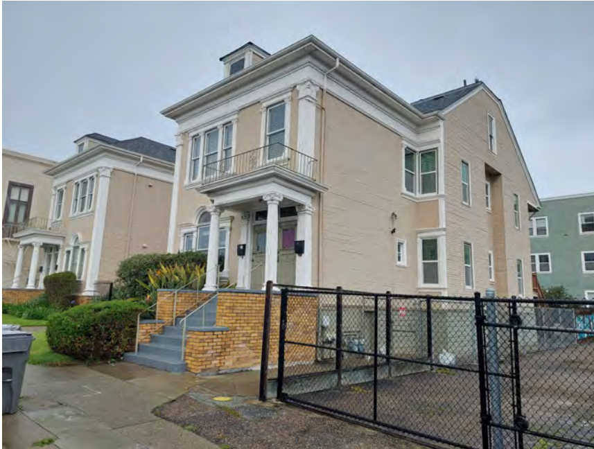
Photograph 2. View of the southern-facing facade and east sides; camera facing northwest, February 29, 2024.
