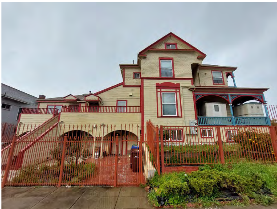
Photograph 3. East side of 51 8 th Street showing rear addition, camera facing west, February 29, 2024.
