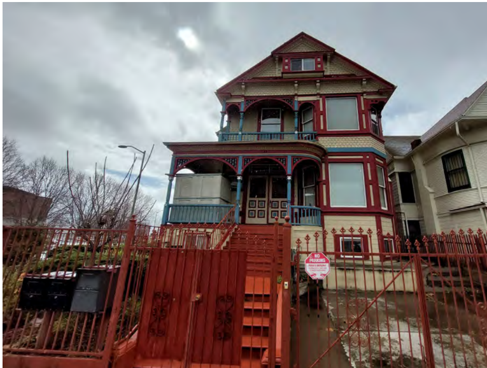
Photograph 2. Northern-facing facade of 51 8 th Street, camera facing south, February 29, 2024.
