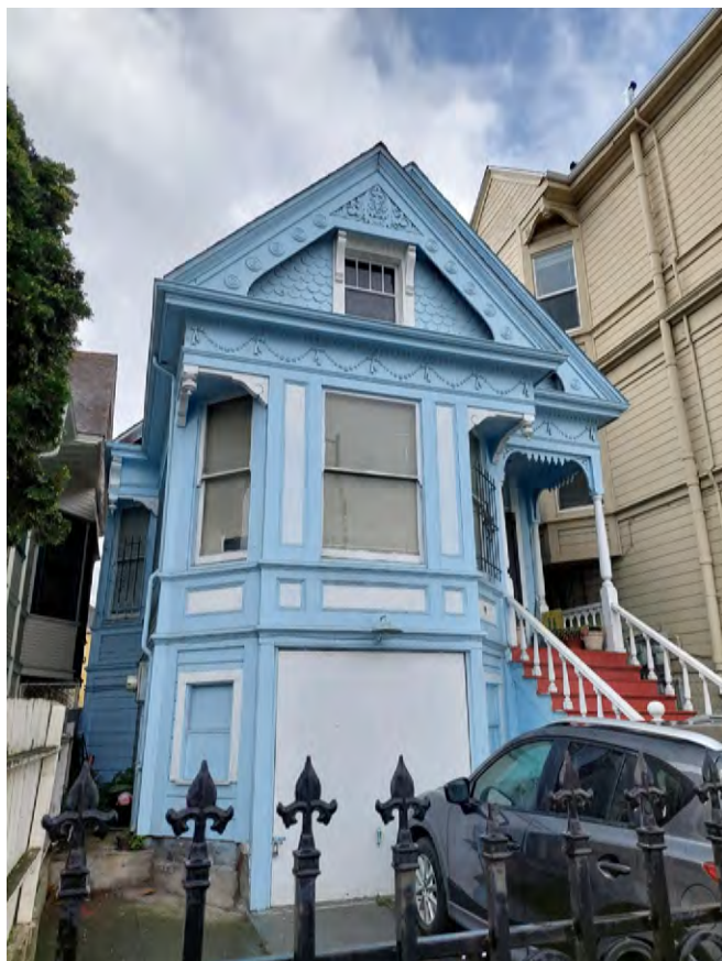
Photograph 2. 59 8th Street, camera facing southwest, February 29, 2024.
