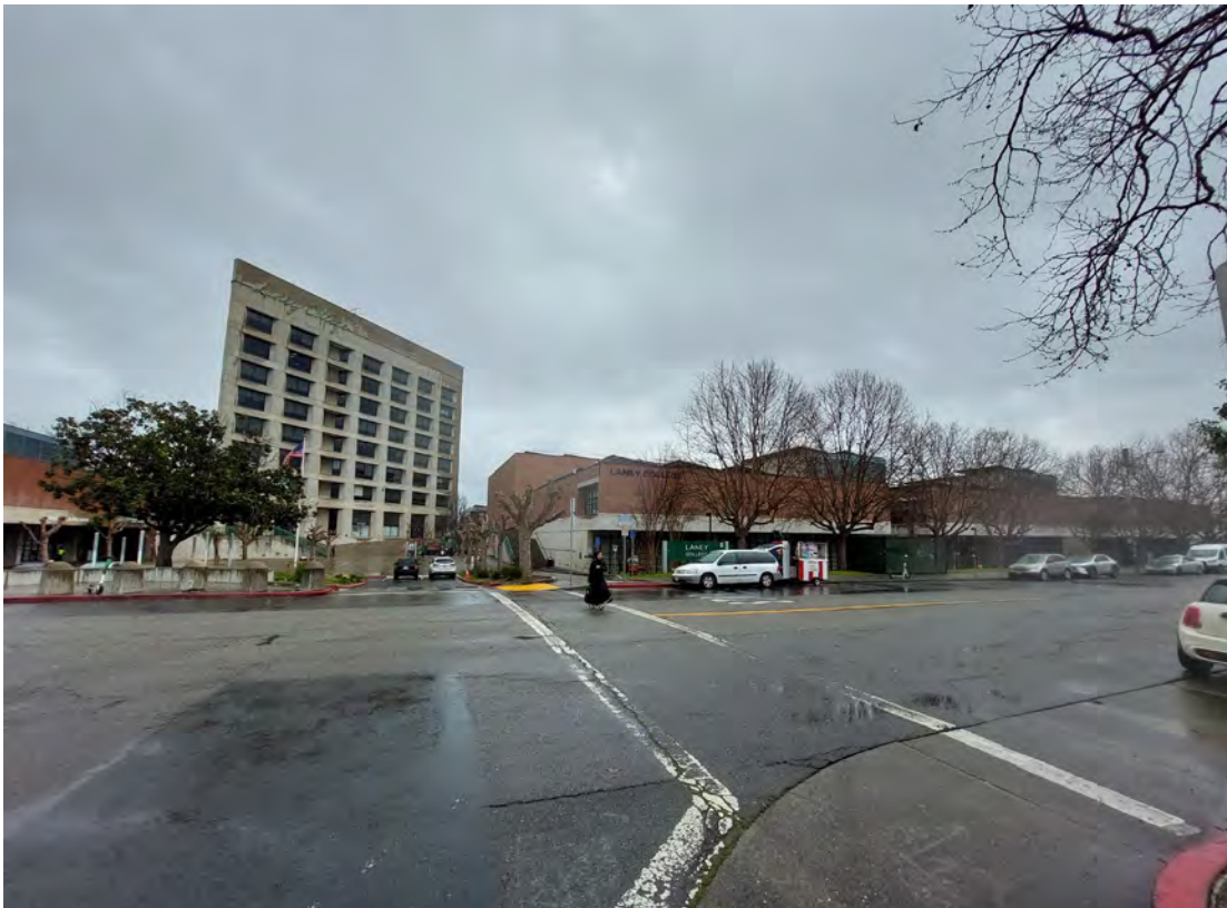
Photograph 3: Laney College at 900 Fallon Street, main public entry point (MR 04)
