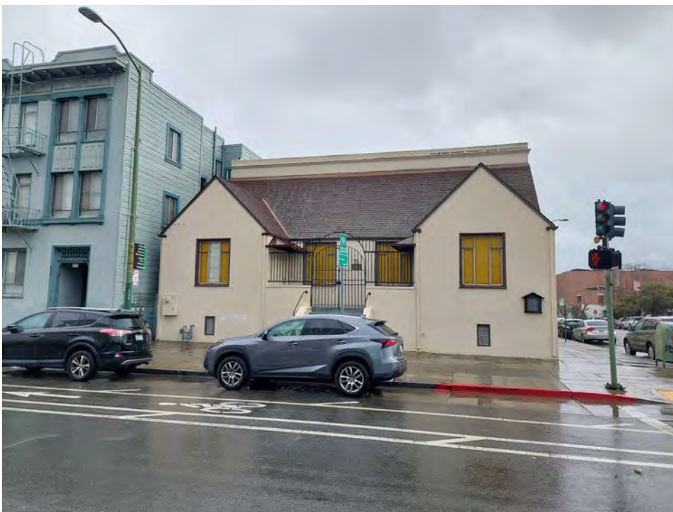
Photograph 3. Western-facing façade; camera facing east, February 29, 2024.
