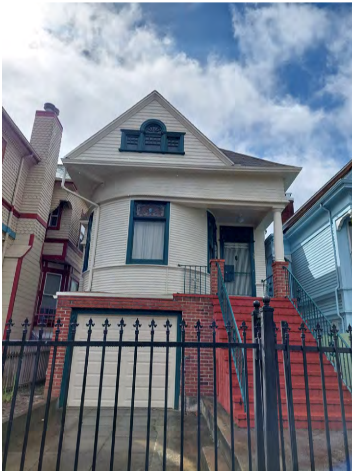
Photograph 2. Northern-facing facade of 5 8th Street, camera facing south, February 29, 2024.
