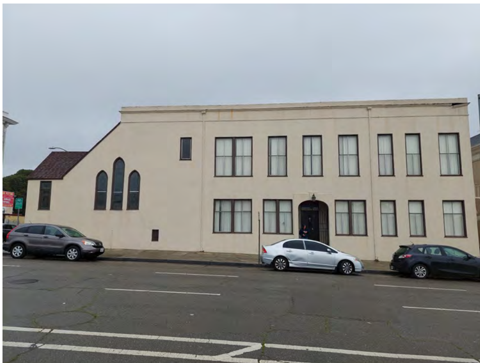
Photograph 5. South side of the building; camera facing north, February 29, 2024.
