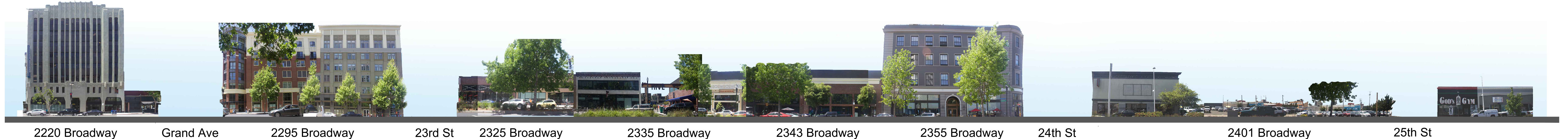
2220 Broadway Grand Ave 2295 Broadway 23rd St 2325 Broadway 2335 Broadway 2343 Broadway 2355 Broadway 24th St 2401 Broadway 25th St
