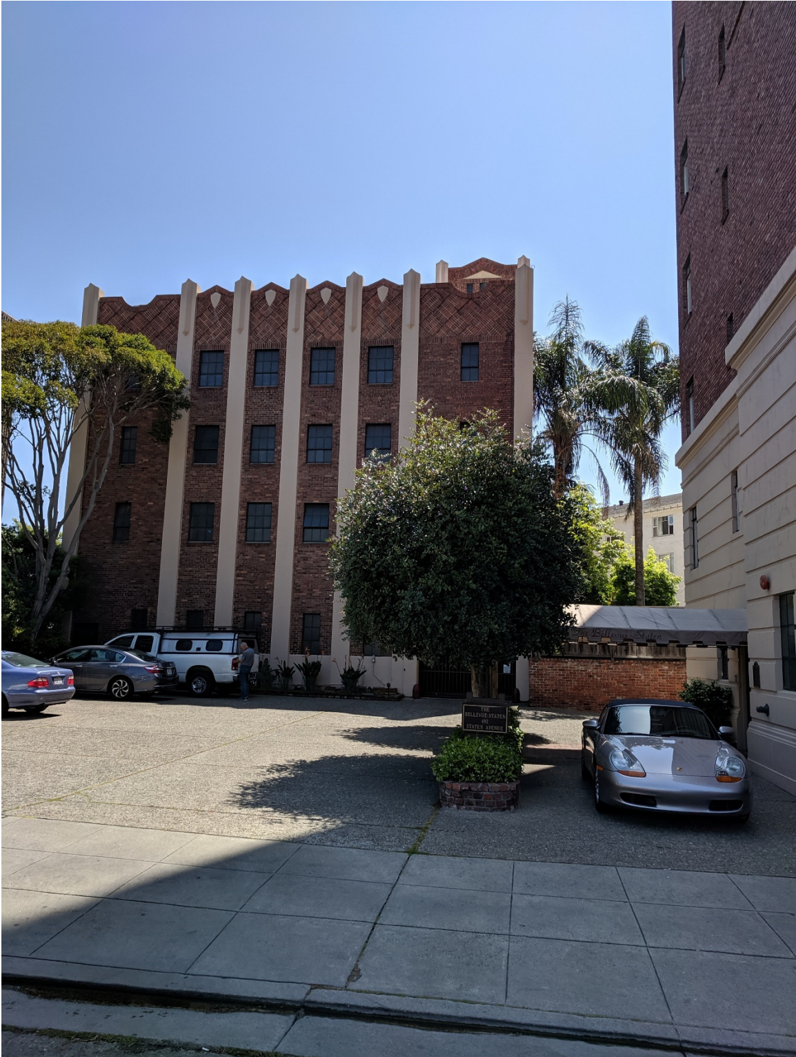
BVS parking lot, entry and original garage structure of brick and art deco design.
