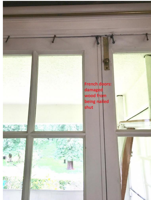
Work Program #5-6: Replace existing French doors to the veranda –deteriorated, missing hardware, nailed shut. This damage is consistent across all three French doors off of the front veranda
