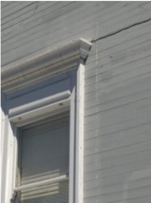
North side windows and siding
