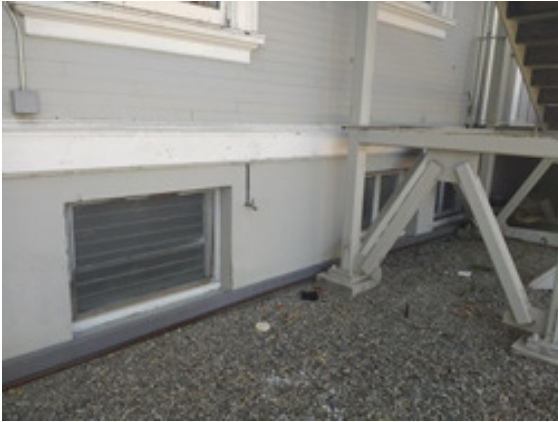
East side basement windows
