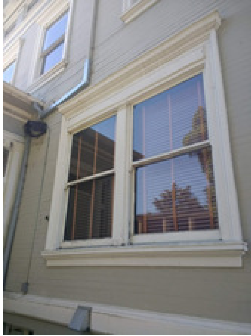
South side windows
