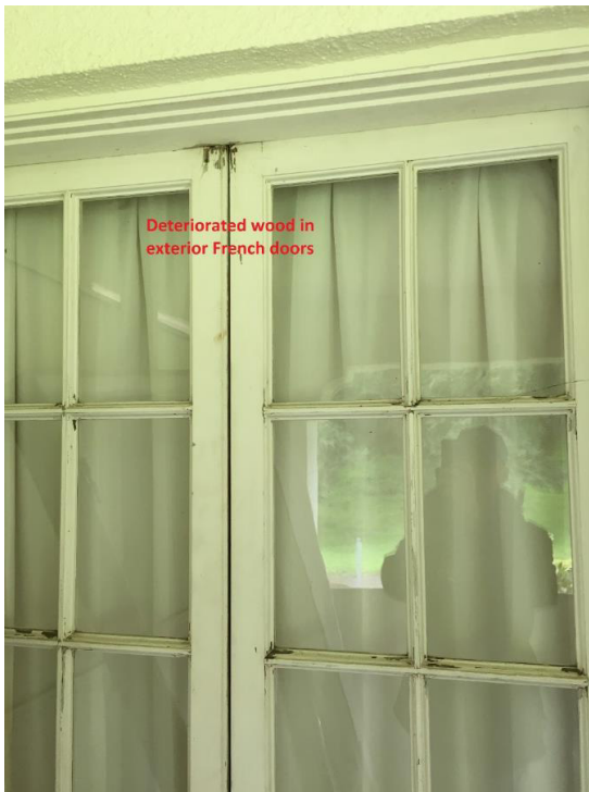
Work Program #7-10: Replace existing wood sashed windows –weathered, delaminated, broken, and or nailed shut Similar damage and weathering to windows throughout the house
