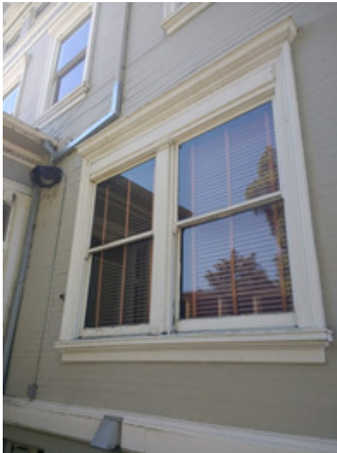
South side windows: former grand room
