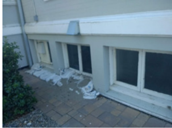
South side basement windows
