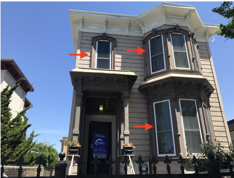
Windows at the property
