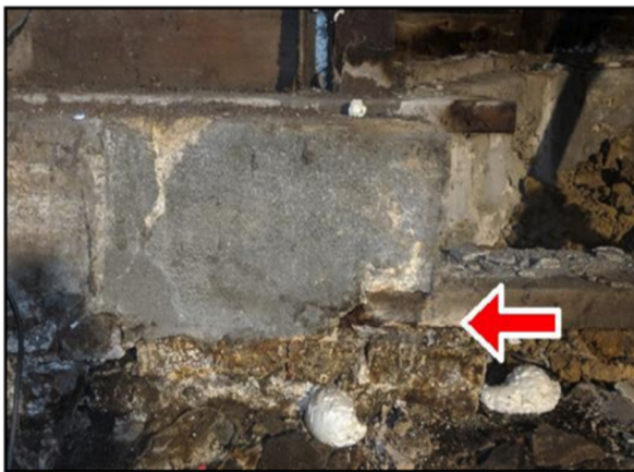
Cap over brick masonry
