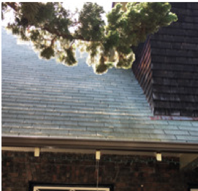
#10: repair or replace roof
