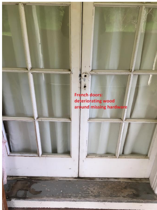
Work Program #7-10: Replace existing wood sashed windows –weathered, delaminated, broken, and or nailed shut Similar damage and weathering to windows throughout the house
