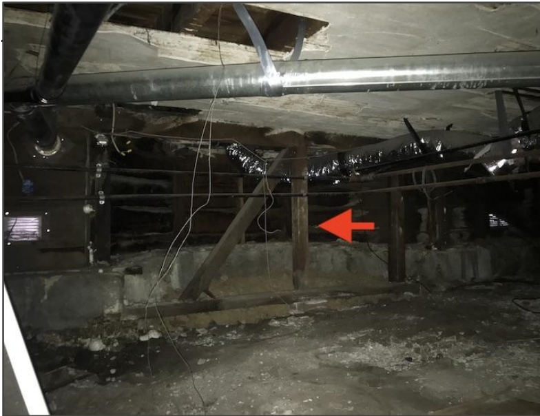
Wooden posts in the crawl space.
