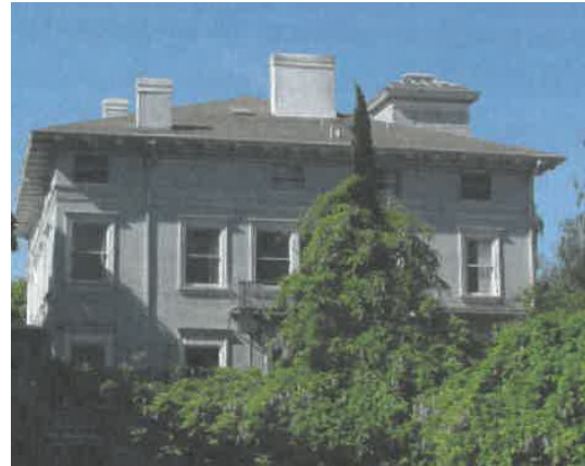
Chimney on the north side in 2007
