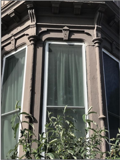
Close up of current window at the property.
