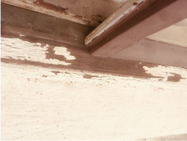
Above left: Condition of sill of casement window facing south in Master Bedroom.
