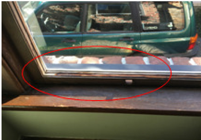
#1: repair windows at front & S side
