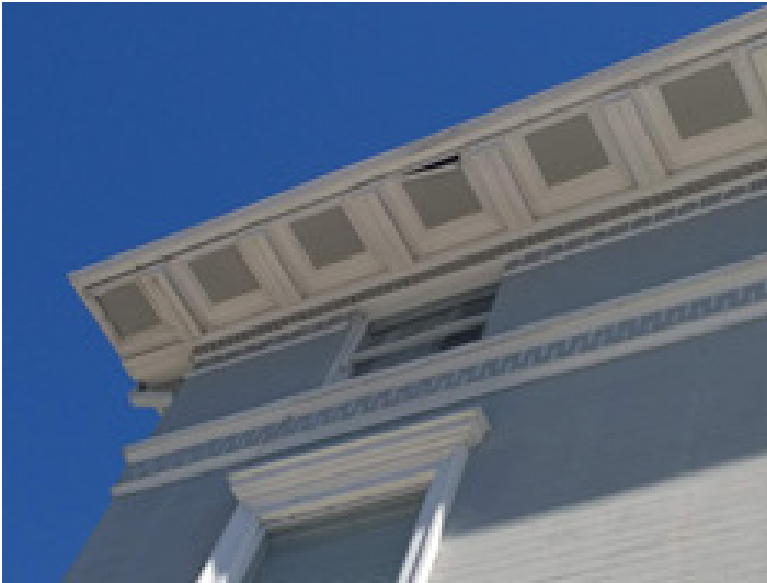
North side eaves
