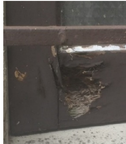
Above left: Condition of sill of casement window facing south in Master Bedroom.
