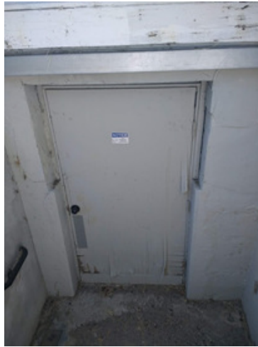
South side basement door
