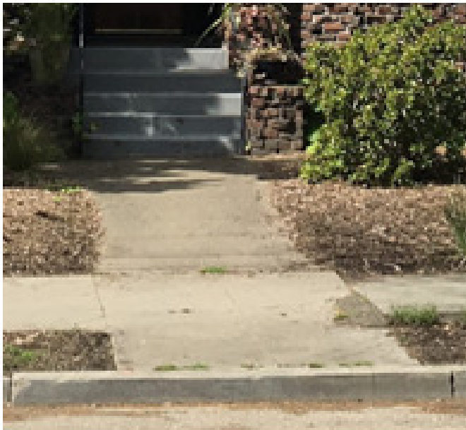
#8: replace concrete path
