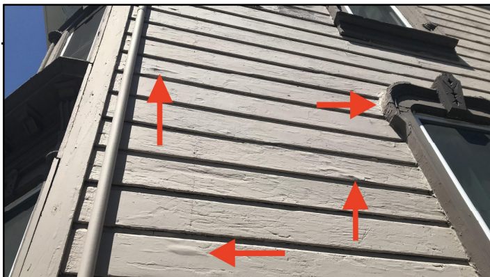
Damaged siding
