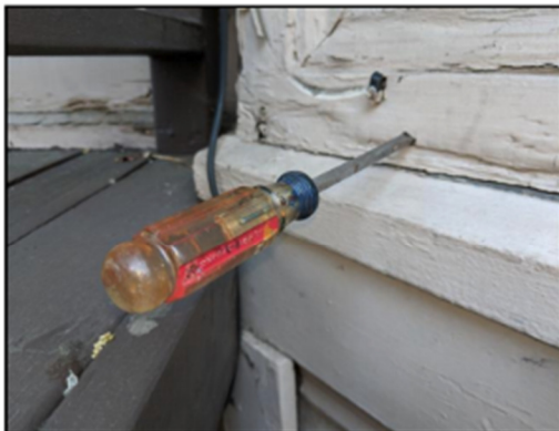
Damaged siding
