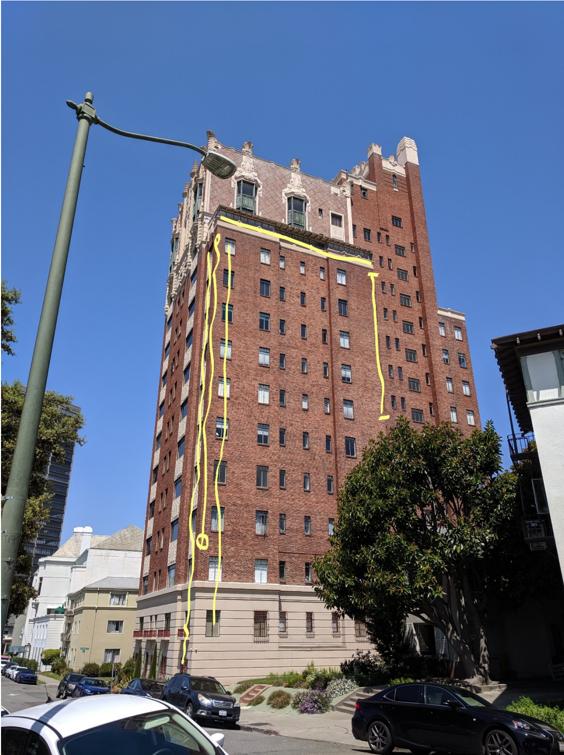
South East Side of BVS. Specific Work, lines left to right:
