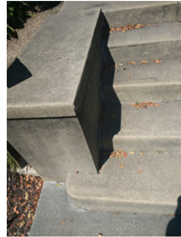
Wing wall on the west side
