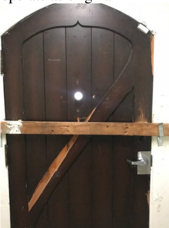
Repair original door at entrance stone at main entrance
