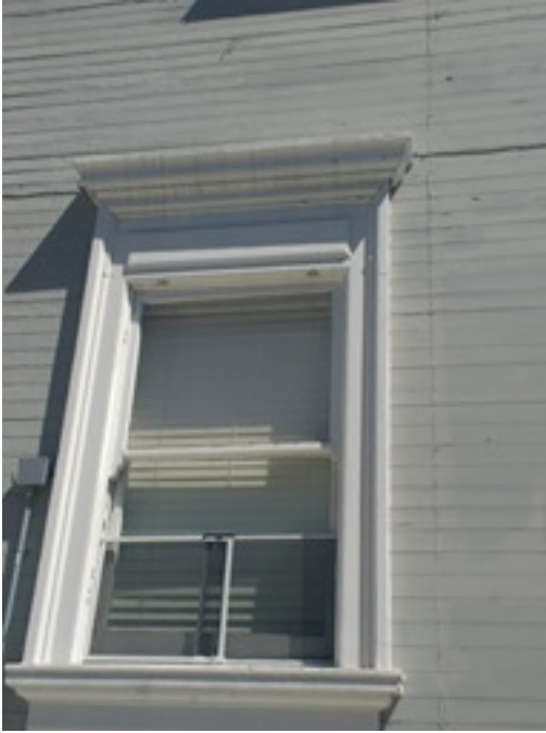
North side windows
