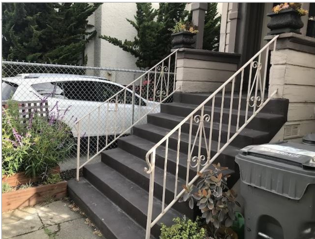
Current Stair railing at 678 18th Street
