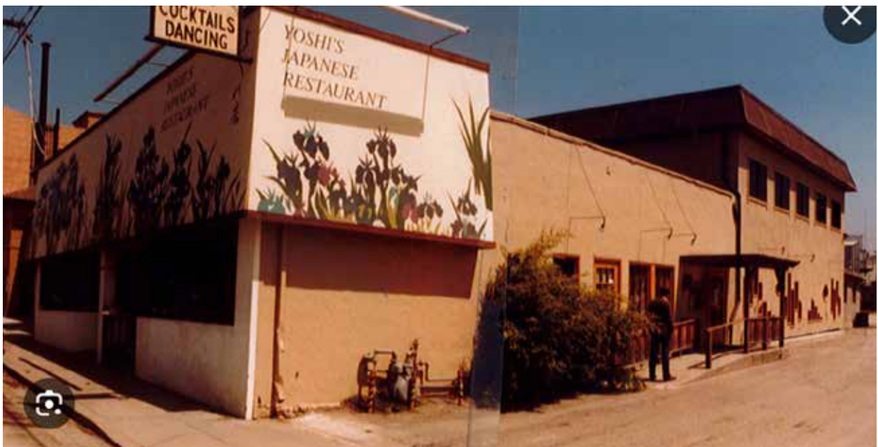
Fig.16 – 6028-30 Claremont Ave. – c1980
