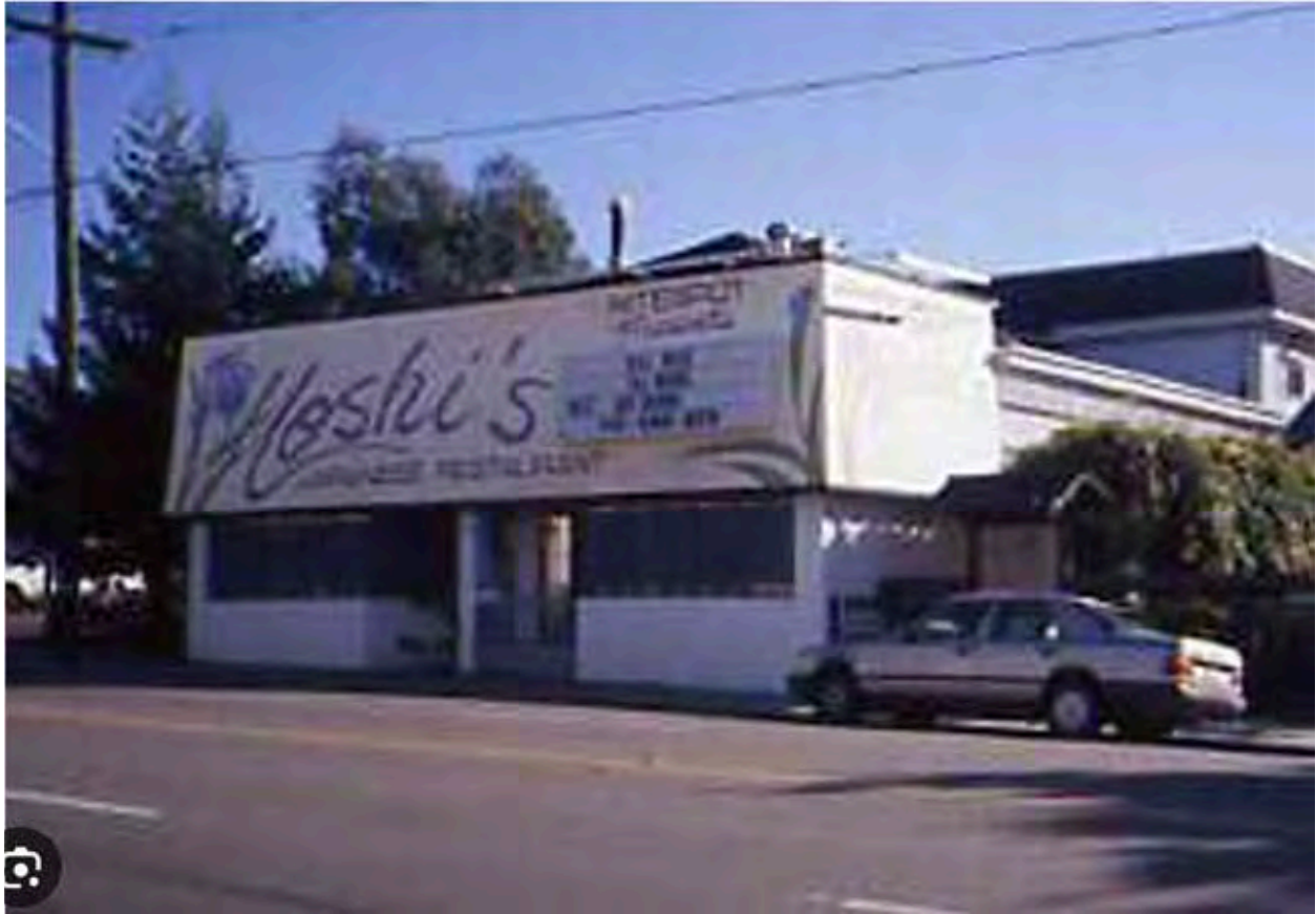
Fig.17 – 6028-30 Claremont Ave. – c1995
