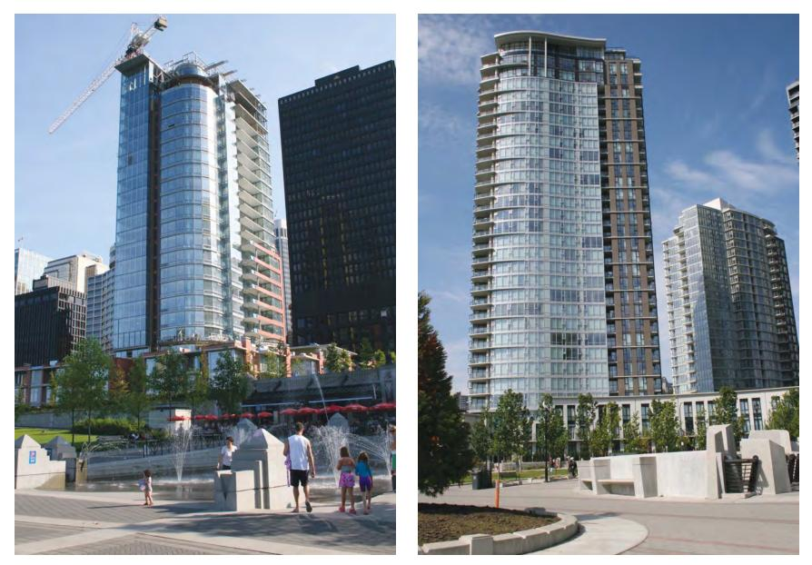
Special treatments (e.g. shaping, fenestration, materials, etc.) like these examples in Vancouver should be employed to accentuate the vertical proportion of towers.
