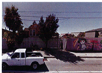
2 3209 & 3221 HOLLIS STREET, DOWN THE STREET FROM THE SITE
