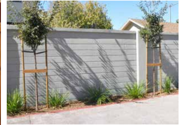
COMMUNITY FENCE, CONCRETE PANEL, 6' TALL
