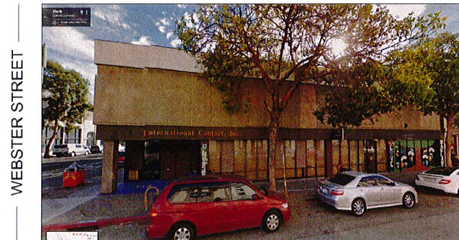
359 15TH STREET (PROJECT SITE)
