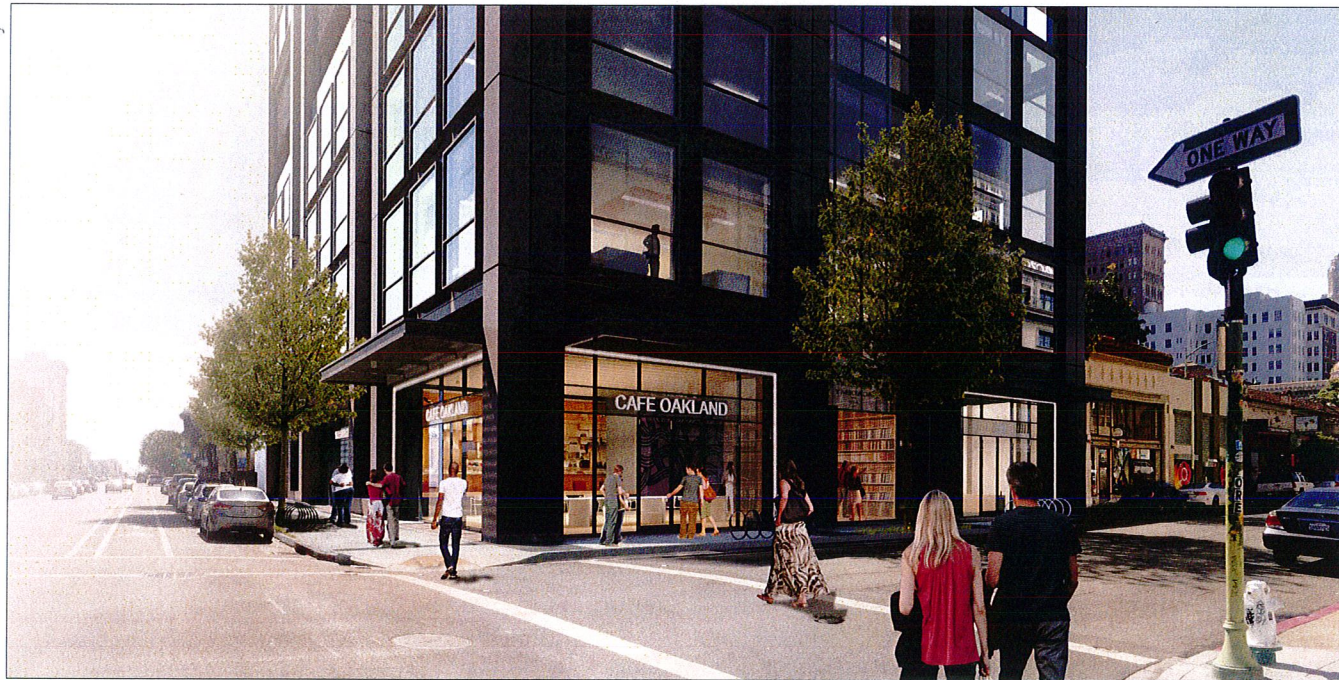
RETAIL AT THE CORNER OF WEBSTER AND 15TH STREET
