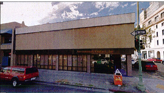
359 15TH STREET (PROJECT SITE)
