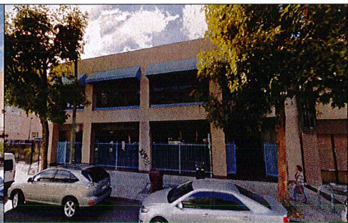
1433 WEBSTER STREET (PROJECT SITE)
