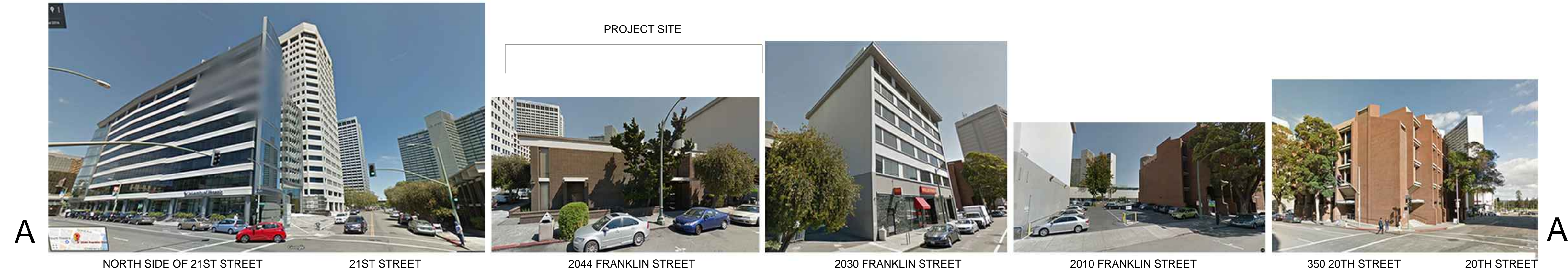
NORTH SIDE OF 21ST STREET 21ST STREET 2044 FRANKLIN STREET 2030 FRANKLIN STREET 2010 FRANKLIN STREET 350 20TH STREET 20TH STREET
