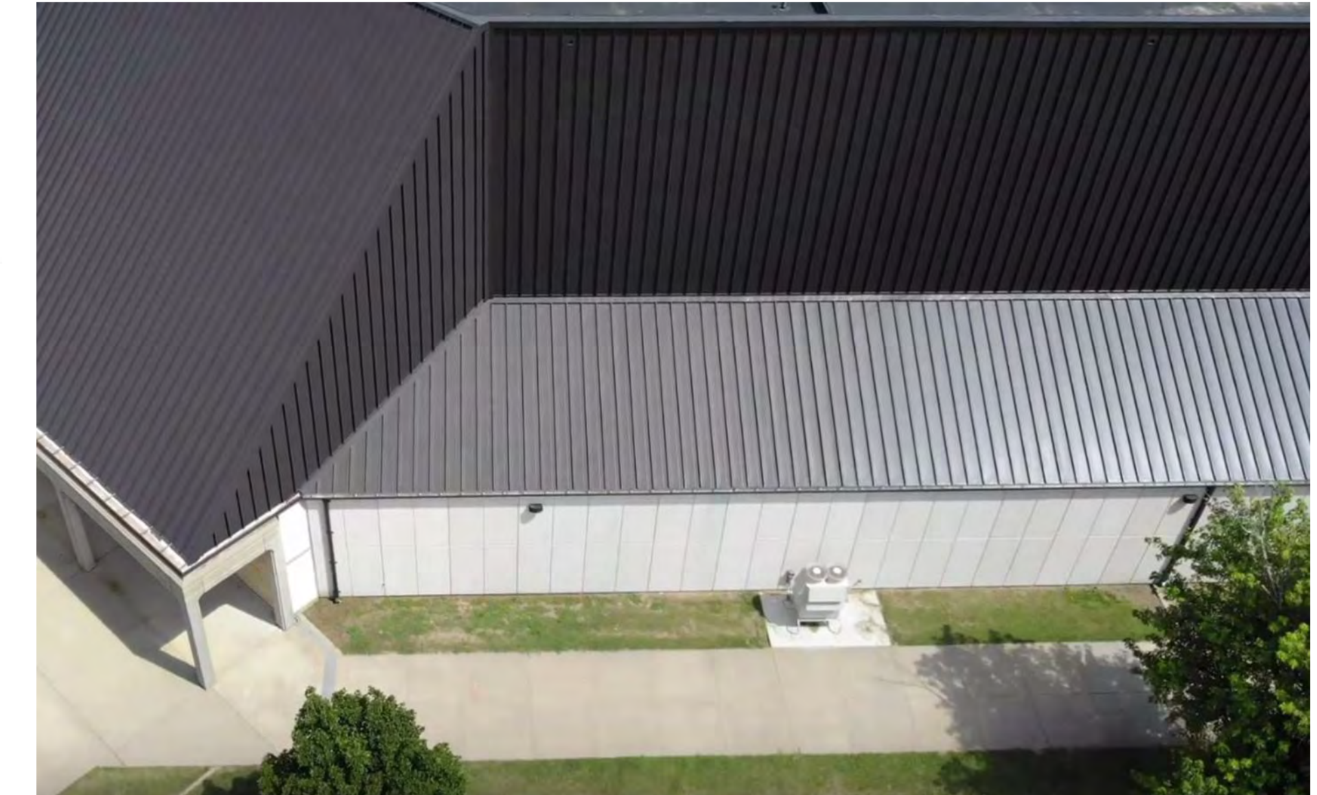
MCELROY METAL - STAND-IN SEAM PANEL 238T SYSTEM - 24" PLANK PREWEATHERED GALVALUMEMETALIC PVDF - METALLIC COLOR
