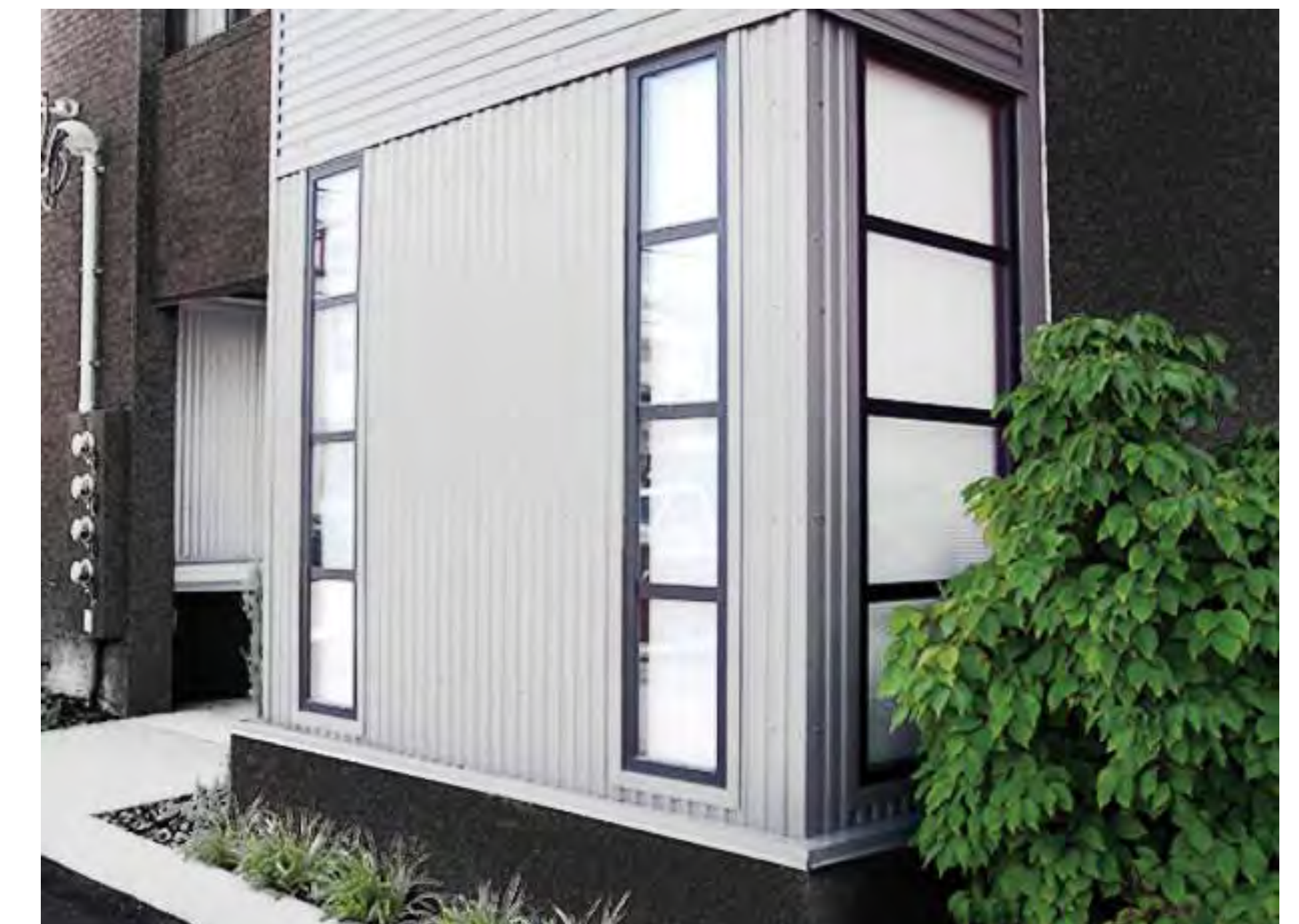
MCELROY METAL - MINI-RIB PANEL 3" VERTICAL RIBBED METAL PANELS REGAL WHITE PVDF - STANDARD COLOR
