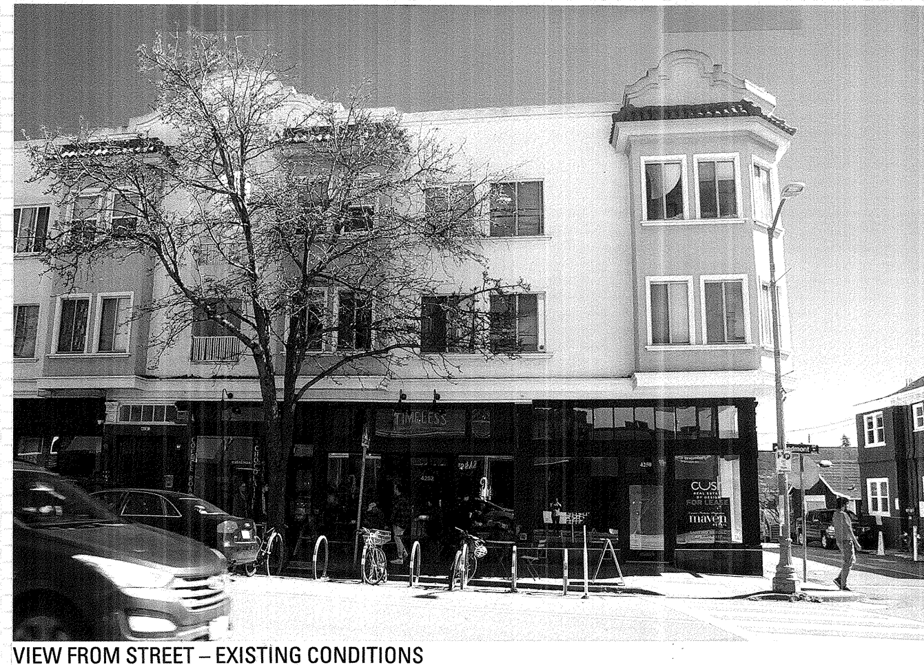
VIEW FROM STREET - EXISTING CONDITIONS
