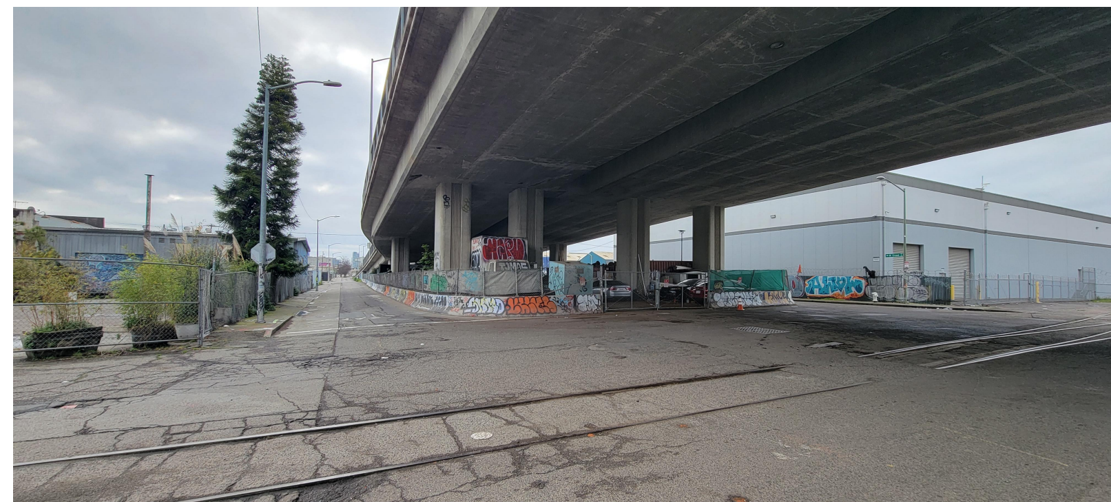
R1_W Grand Ave overpass and storage_at Wood St
