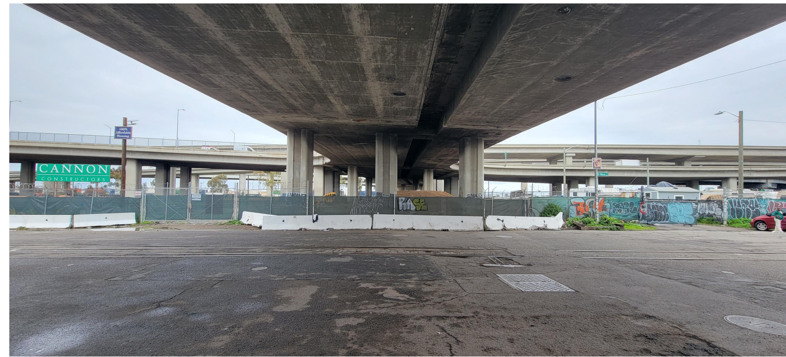
AC 5 W Grand Overpass facing NW
