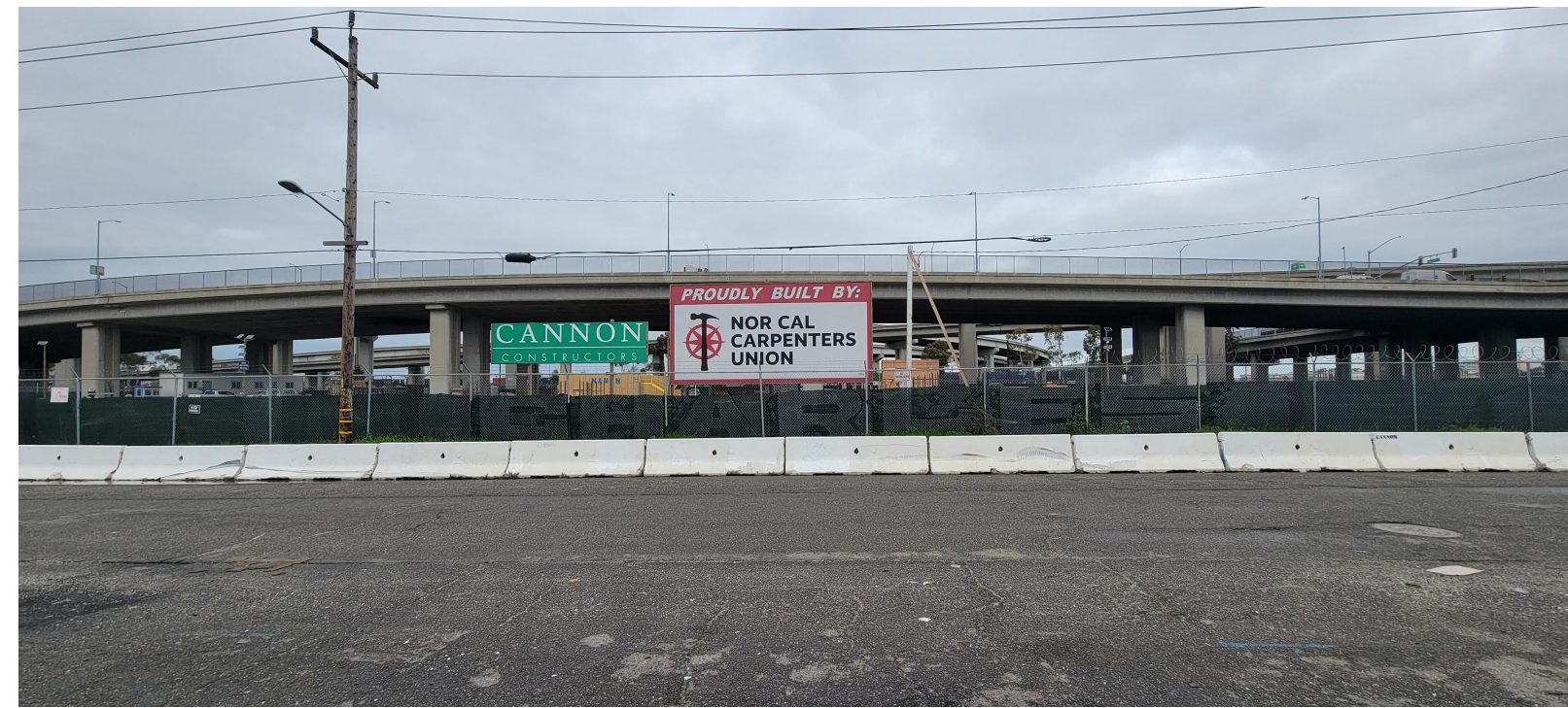
AC 4 7800 Frontage Rd_Viewed from Wood St_Cannon Construction Affordable Housing_2
