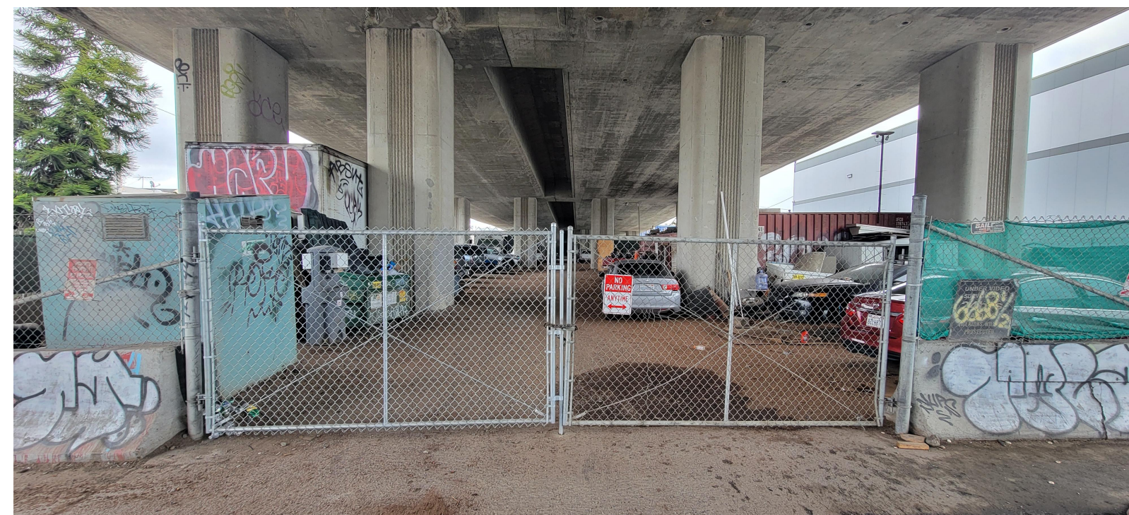
R1_W Grand Ave overpass and storage_at Wood St_2
