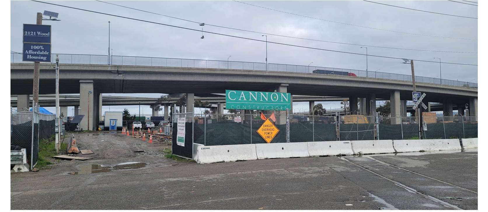
AC 3 2121 Wood St Cannon Construction Affordable Housing
