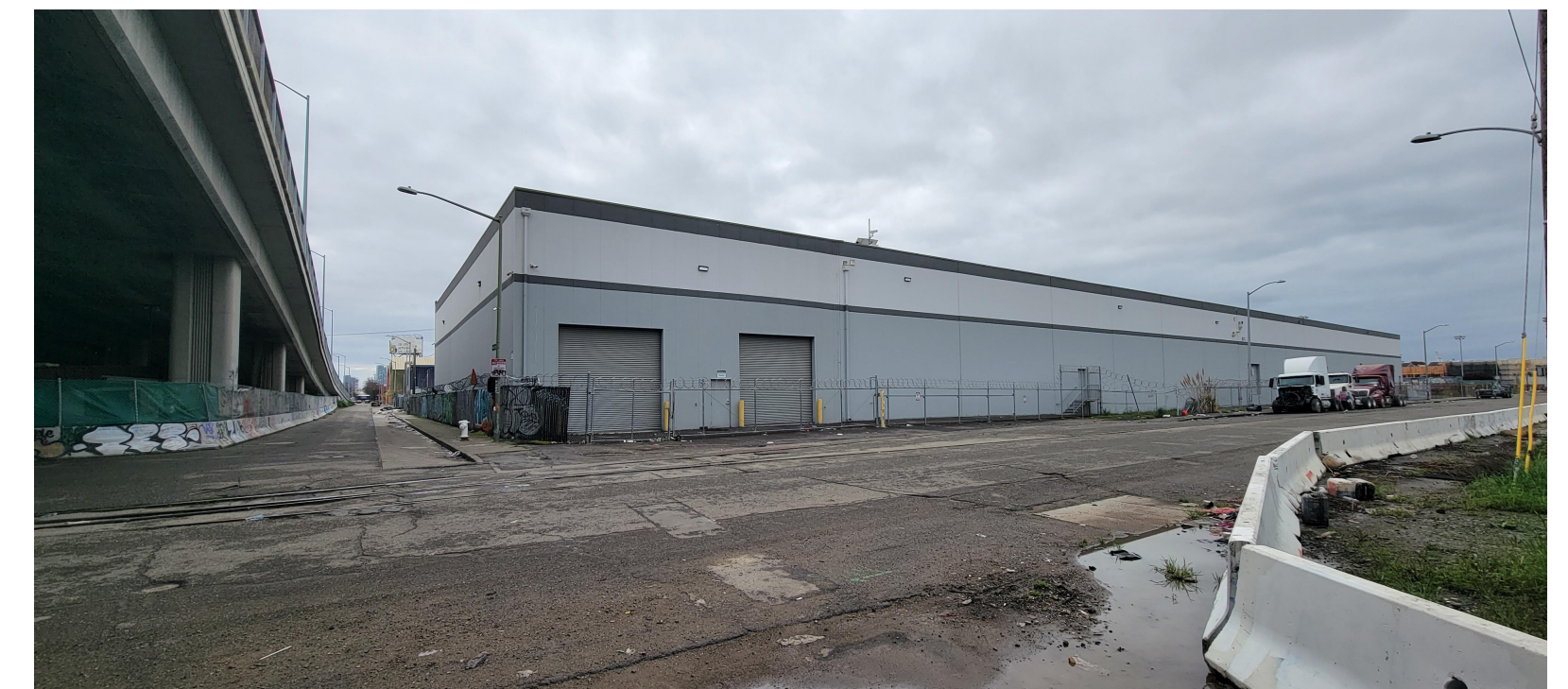
R2_1700 20th St_From Wood Street_MR Sandoval Construction
