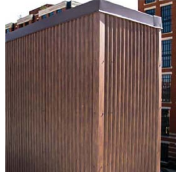
2 OXIDIZED CORRUGATED METAL SIDING
