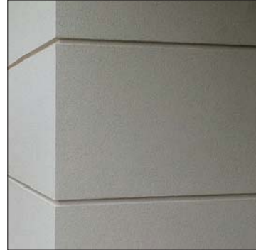
1 SAND FLOAT TEXTURE CEMENT PLASTER: CONTROL JOINT REVEALS SHERWIN WILLIAMS 'EIDER WHITE' - SW 7014 OR SIMILAR
