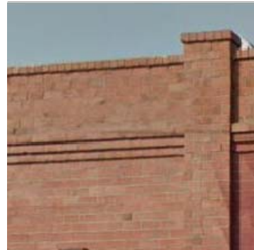
4 PRESERVED AND RESTORED BRICK FACADE
