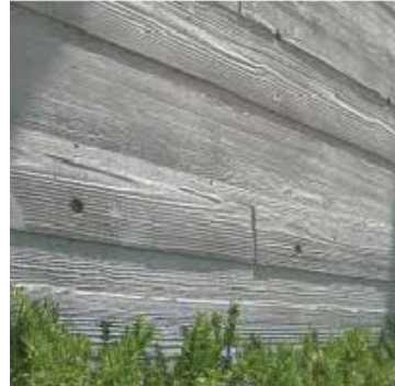
3 BOARD FORMED CONCRETE
