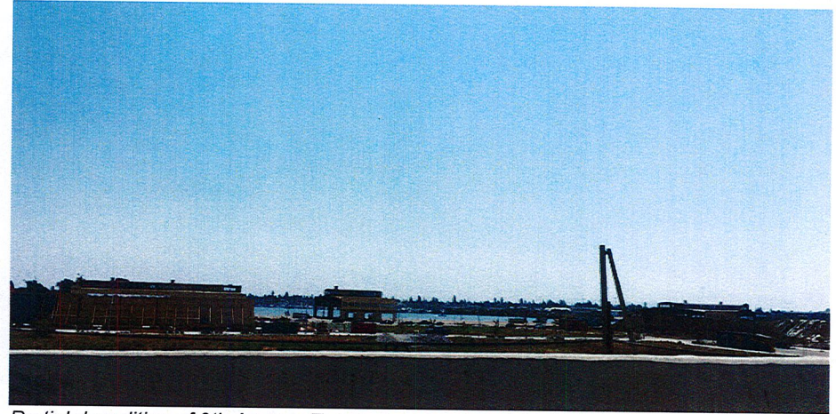
Partial demolition of 9th Avenue Terminal and new water view
