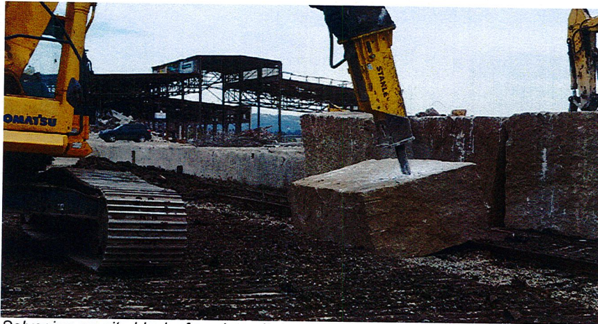
Salvaging granite blocks found on site
