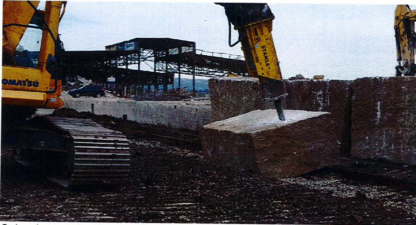
Salvaging granite blocks found on site.
