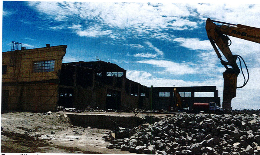
Demolition in progress
