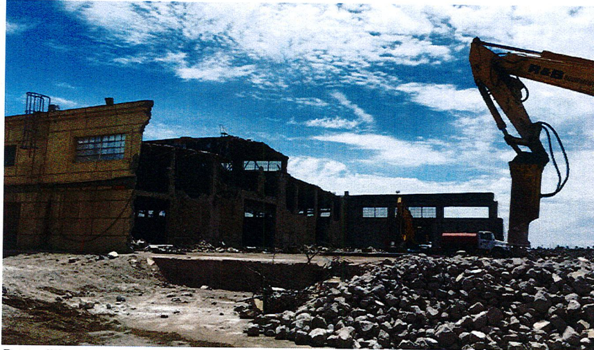
Demolition in progress
