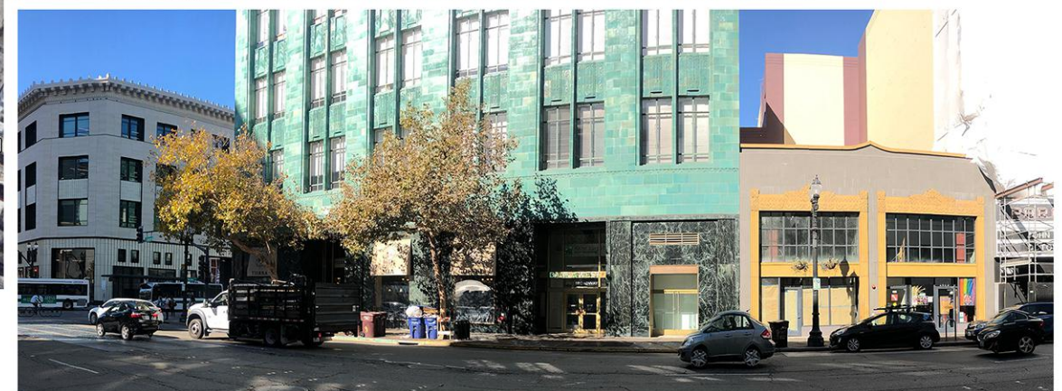
North / West View
