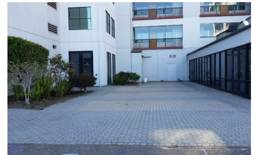
4: View of Parcel D looking west
