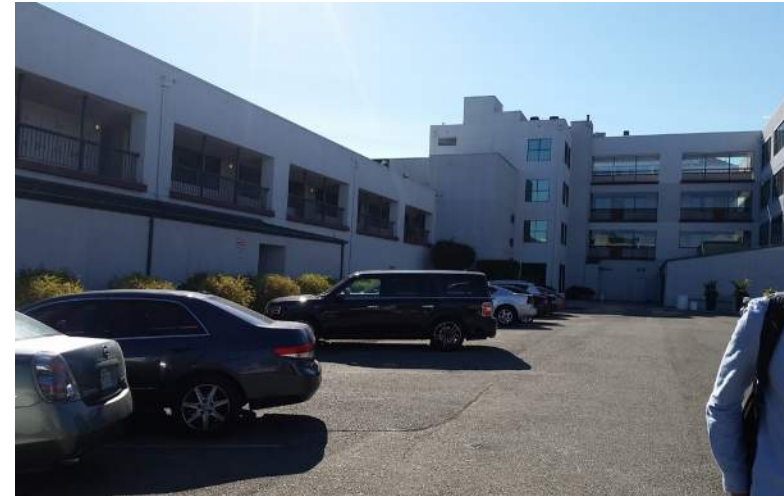
1: View of Parcel D looking west
