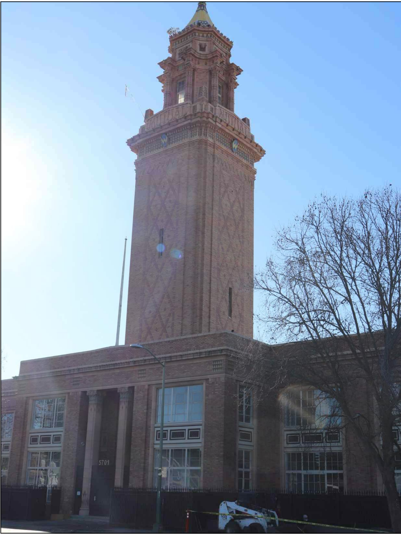
5701 International Blvd. looking West
