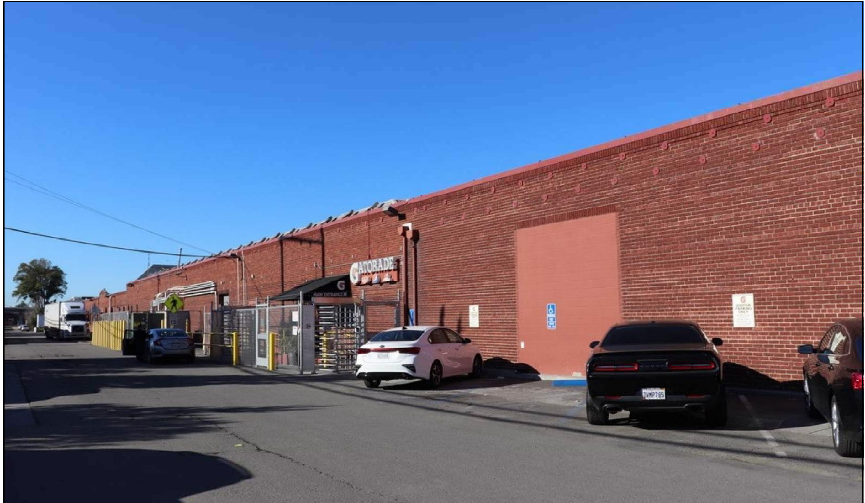
5625 International Blvd. Southern side of building along 57th St. looking Southwest from 57th St.
