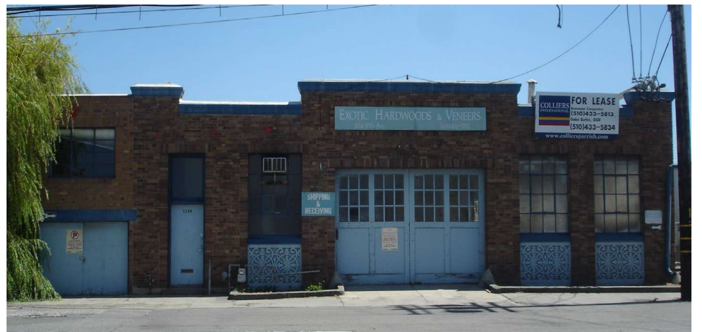
1154 57th AVENUE, NORTH FACADE
