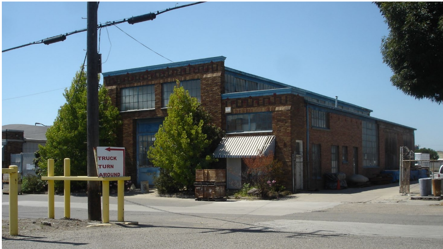
1135 57th AVENUE, SOUTH AND EAST FACADE
