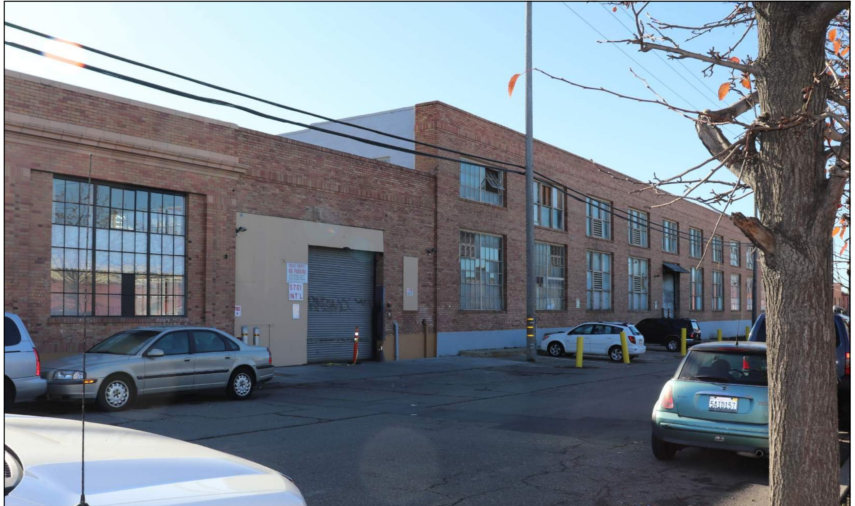
Rear portion of North side of 5701 International Blvd. looking Southwest from 57th St.
