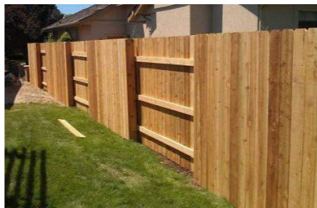
GOOD NEIGHBOR FENCE
