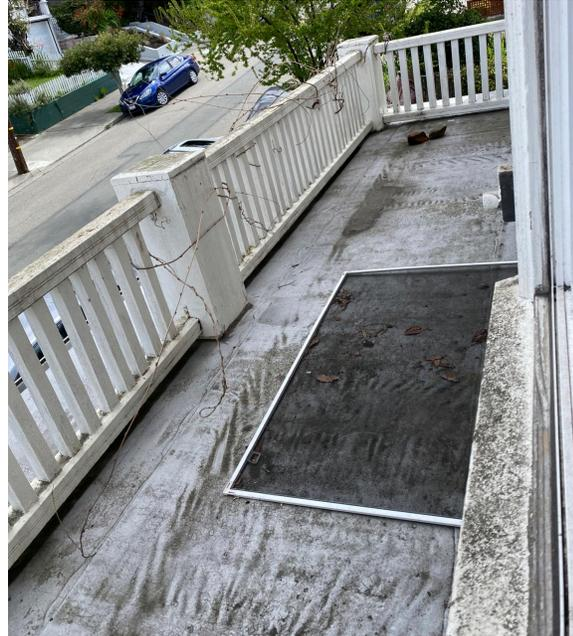
**Images 17 and 18** Show the balcony railing needs to be sanded, sealed, and repainted to maintain its integrity. If enough of these are found to be rotted beyond repair, they will need to be replaced. The flooring may also need to be replaced to prevent any leaking through the floor, down to the front porch.
