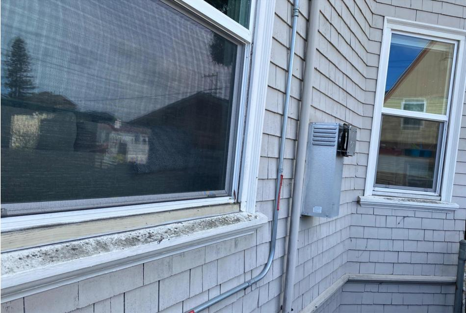
**Image 20** shows mildew on 2 window trims, many of the sills are in this condition and need to be sanded, sealed, and repainted or replaced if beyond repair . All trim would also be repainted at this time.
