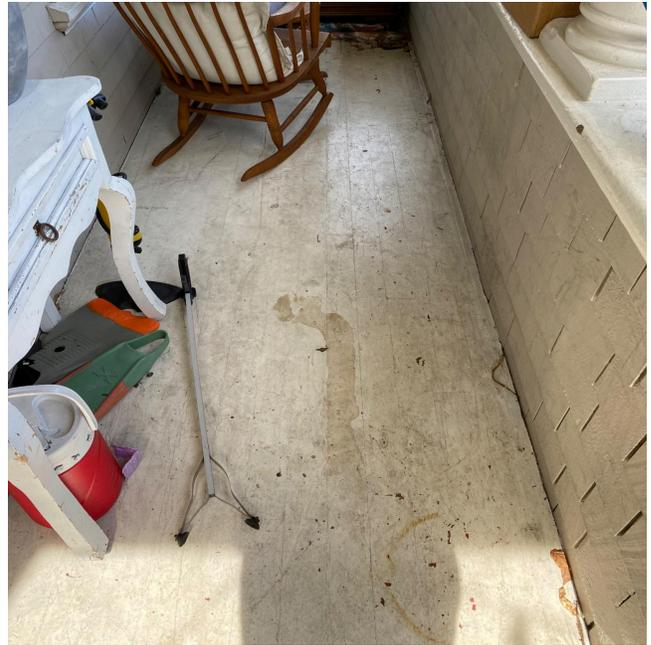
**Images 13 and 14** show the wood front porch that needs to be repaired, sanded and repainted. The concrete steps would also be replaced to match the wood style. Concrete in front of the steps would be sanded, cleaned, and repainted, or replaced with a historically appropriate brick or paver.
