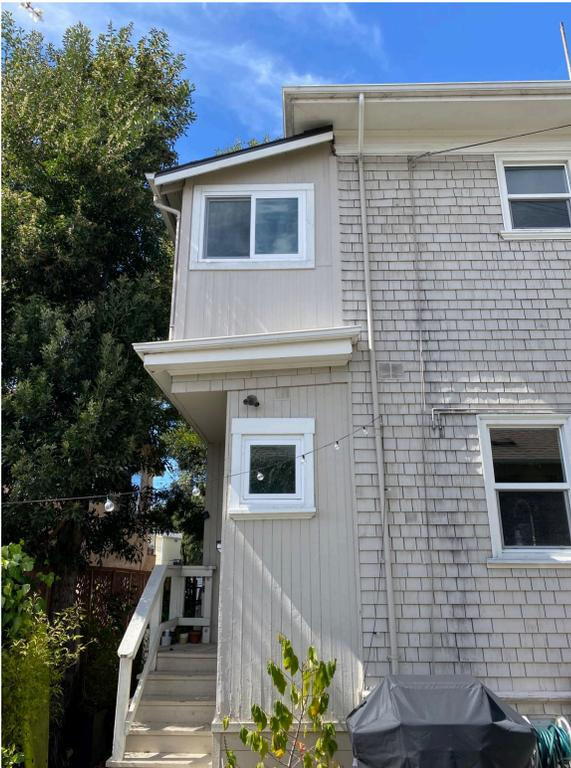
**Image 21** shows the side of the right side of the house where the two rearmost windows need their trims rebuilt to match the other historic trims. All of these window trims need to be sanded, sealed, repainted, and repaired as needed, along with the ones all around the house.
