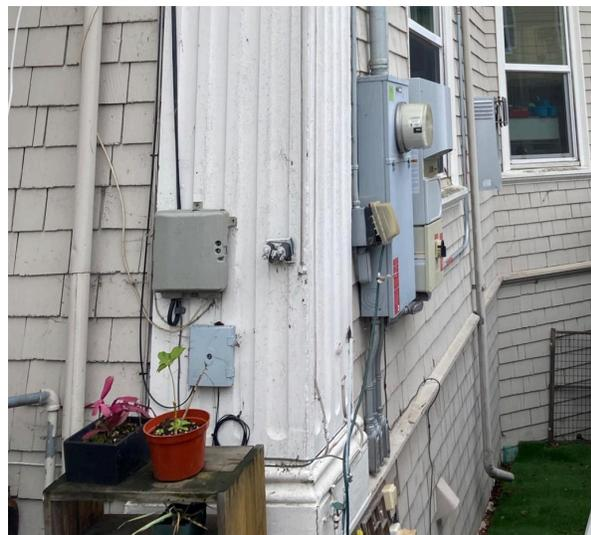
**Images 15 and 16** show each corner wooden fluted pilaster in need of sanding, sealing, and repainting.
