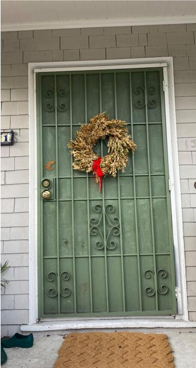
**Image 3** shows the security screen door that does not match the style of the house. Ideally a more historically appropriate security door can be used, or if not, a historic screen door, salvaged if possible.
