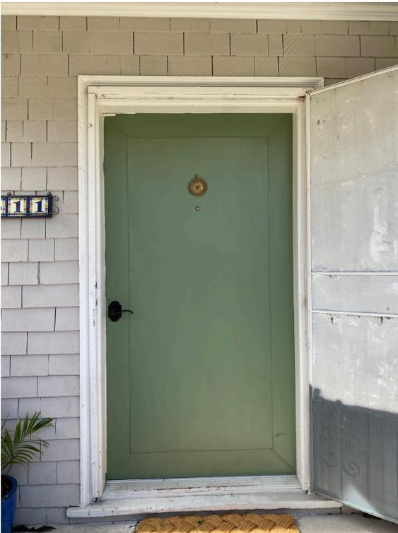
**Image 4** shows the steel front door that does not match the style of the house. The plan will be to replace the existing door with a beautiful, salvaged wood door with partial glass similar to other homes of this time period. See examples below. If a door cannot be salvaged then a new, but historically appropriate door will be used instead. Due to the unusual size of the door (39" x 72") a salvaged door may not be possible.
