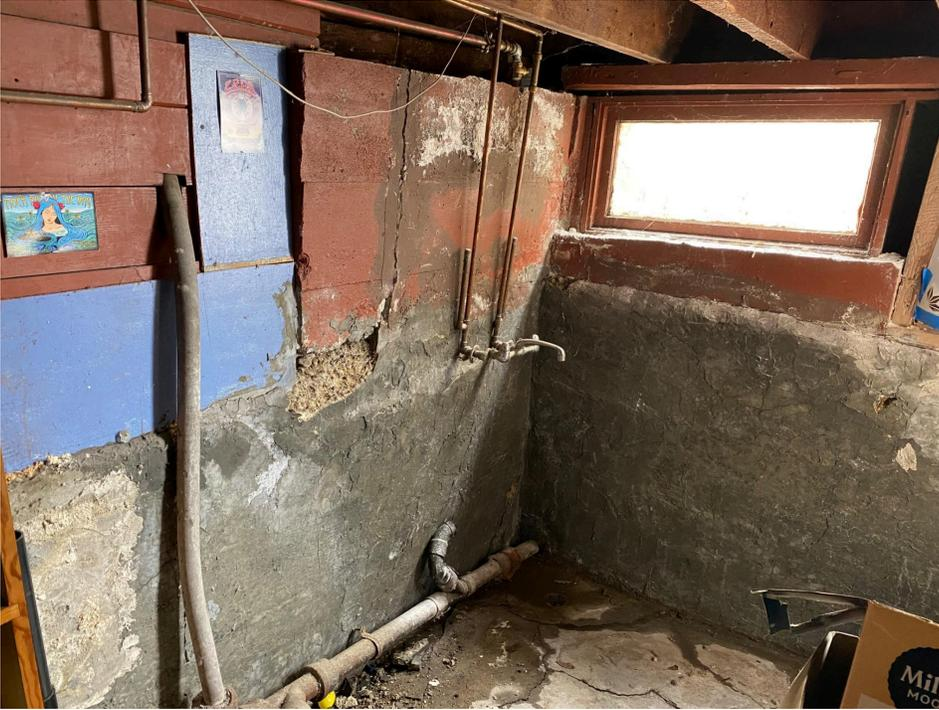
**Image 1** shows foundation cracks that are past the point of repair and require replacement. Second area is difficult to photograph due to location and lack of light, but can be seen in the plans from the civil engineer (attached).
