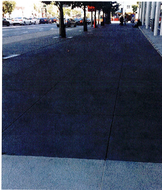
PAVING PRECEDENT - POURED IN PLACE CONCRETE WITH INTEGRAL COLOR
