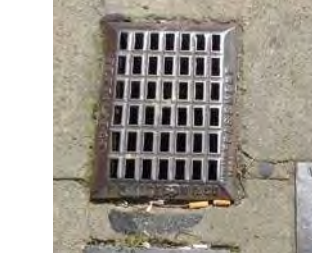
EXISTING METAL VENT
