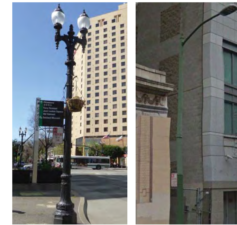
EXISTING BROADWAY STREET LIGHT - TO BE REPAINTED EXISTING 11TH AND 12TH STREET LIGHT - TO BE REPAINTED
