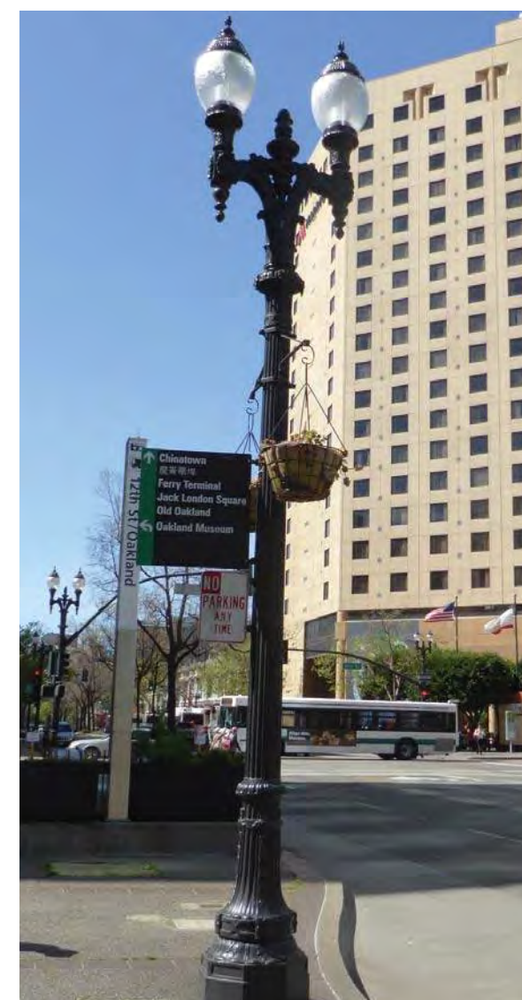
EXISTING BROADWAY STREET LIGHT - TO BE REPAINTED
