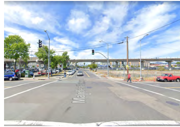
13-Mandela Parkway and 5th st.
