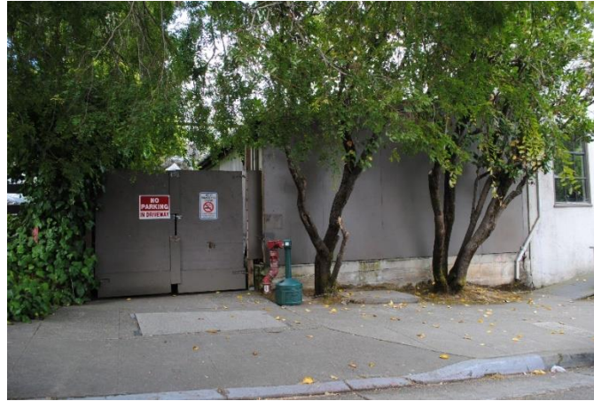
Figure 41. Non-original shed roof addition which abuts the east façade of the Facilities Building, visible at the primary (north) façade, looking south.
