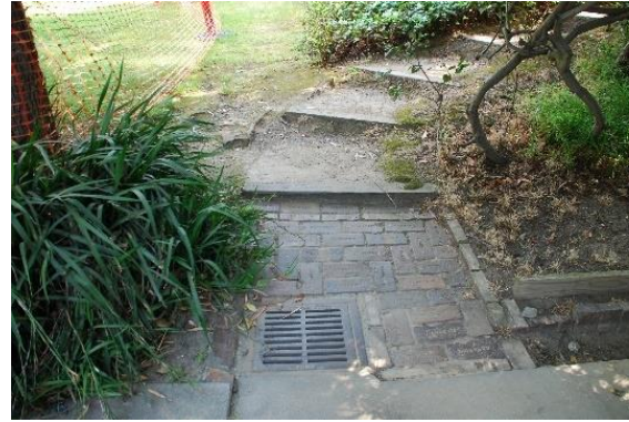
Figure 152. Carnegie bricks used to pave portion of steps near the west end of Founders Hall.
