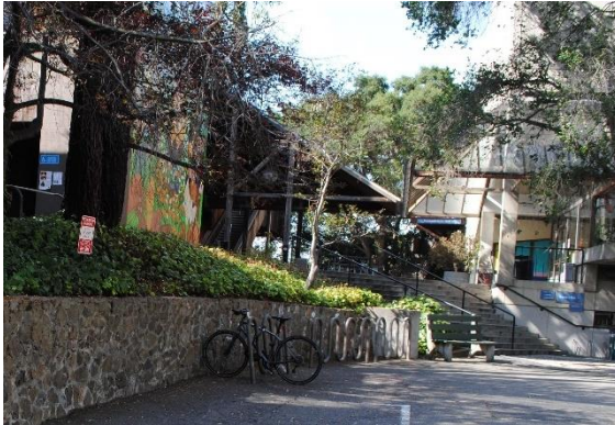
Figure 64. Martinez Hall (left) and Founders Hall (right) accessed by concrete stairs, with rock retaining wall, looking south.
