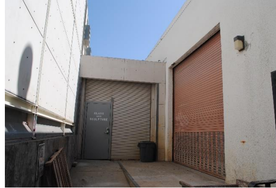
Figure 144. Metal roll-up door accessed via a concrete ramp on the north side of the hyphen between Barclay Simpson Sculpture Studio (left) and the Shaklee Building (right).
