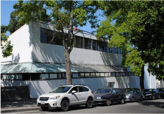
Figure 120. Shaklee Building, north façade, east portion, facing southwest.
