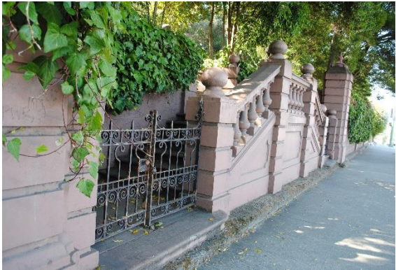
Figure 29. Broadway Wall, stair entrance, facing southeast.
