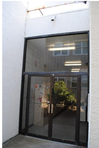
Figure 125. Aluminum storefront window wall with double doors on the south façade of the Shaklee Building, looking north.
