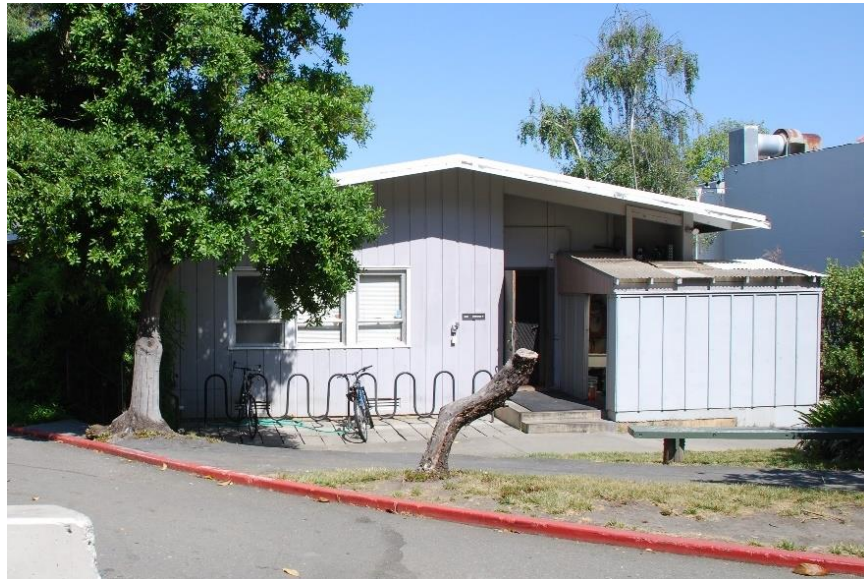
Figure 52. Irwin Student Center, east façade of the east-west ell, facing west.
