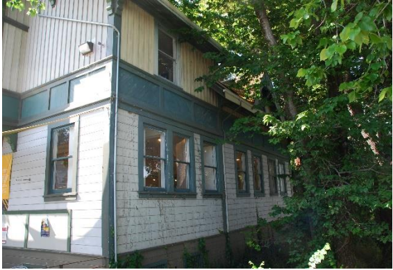
Figure 21. Carriage House, north and west façades, facing southeast.
