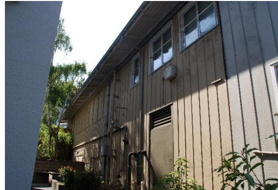
Figure 55. Partial view of the east end of the north façade of Irwin Student Center, looking southeast.
