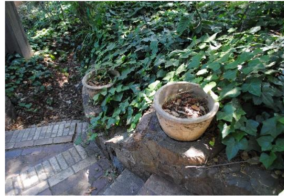
Figure 166. Staircase paved with Carnegie bricks, flanked by masonry retaining walls with ceramic pots.
