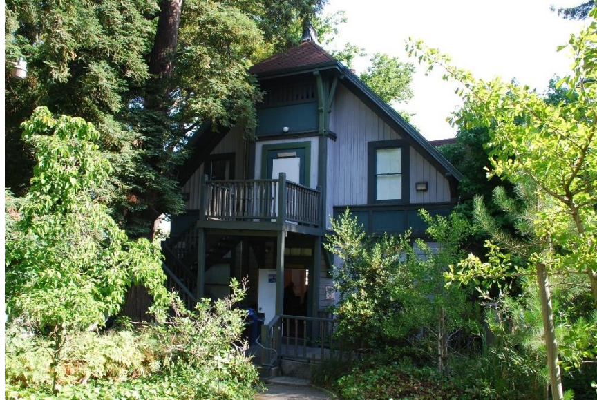
Figure 18. Carriage House, partial view of primary (south) façade and east façade, facing north.
