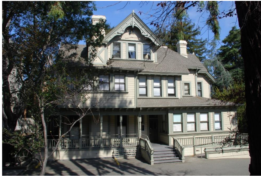
Figure 12. Macky Hall, east (rear) façade, facing west.
