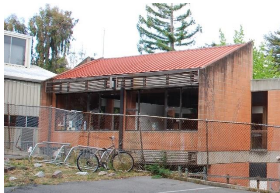
Figure 107. Ceramic Arts Center, portion of east façade with shed roof, looking southeast.
