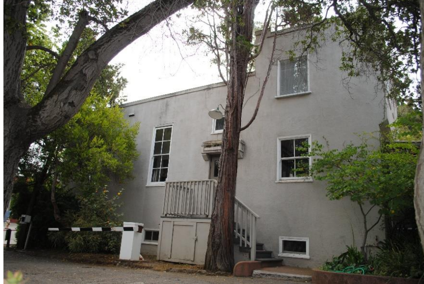
Figure 39. Facilities Building, west façade, facing east.
