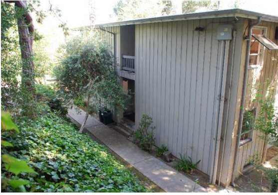
Figure 56. Irwin Student Center, south façade of the north-south wing, looking northwest.
