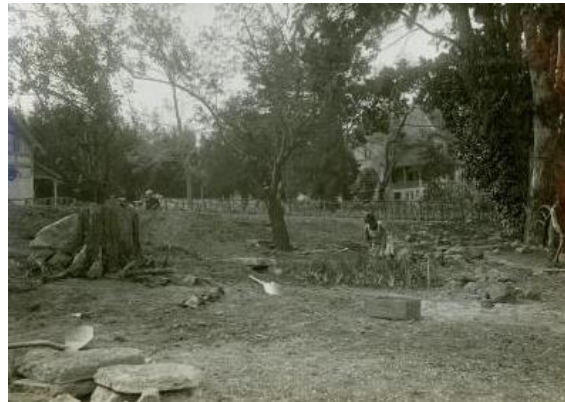
Figure 199. Students clearing land and planting, with partial view of carriage house at left, 1924. Source: CCA Libraries Special Collections.
