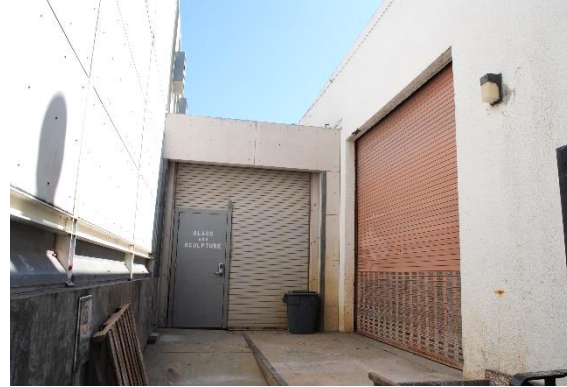
Figure 123. Large metal roll-up door at the south end of the west façade of Shaklee Building (right), looking south. A hyphen addition attaches to Barclay Simpson Sculpture Studio (left).
