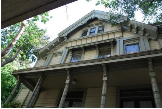
Figure 13. Macky Hall, south façade, partial view, facing north.
