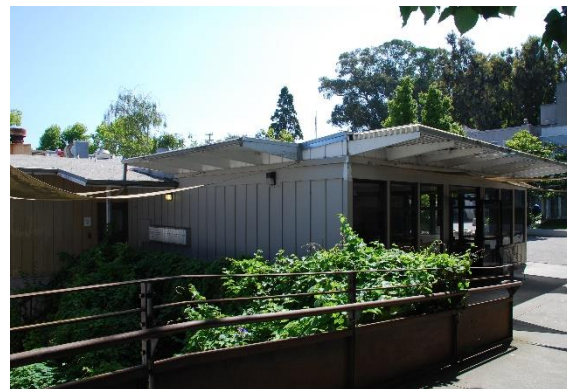
Figure 59. A-2 Cafe, west and south façades, facing northeast.
