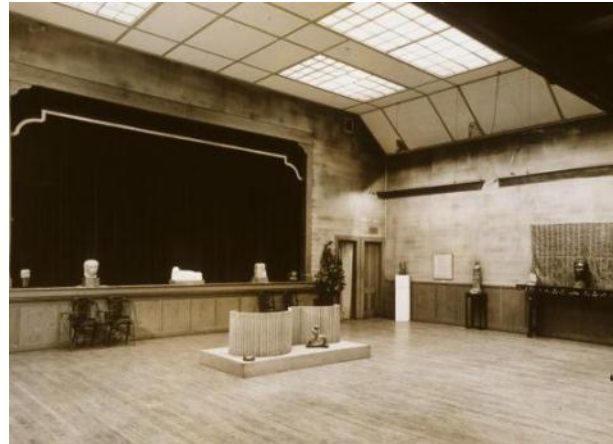
Figure 203. Guild Hall auditorium, no date, estimated 1930. Source: CCA Libraries Special Collections.
