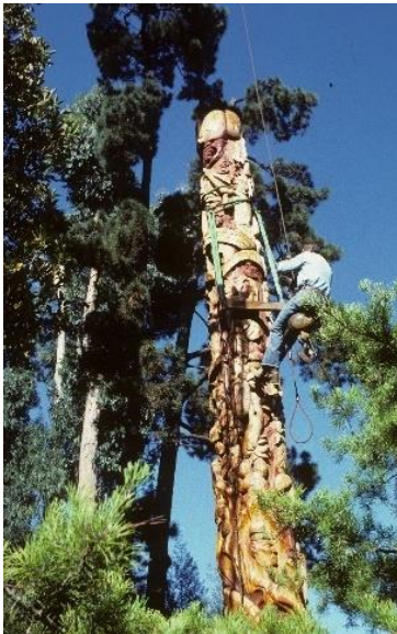
Figure 171. Installation of the Celebration Pole, 1982. Source: CCA Libraries Special Collections.
