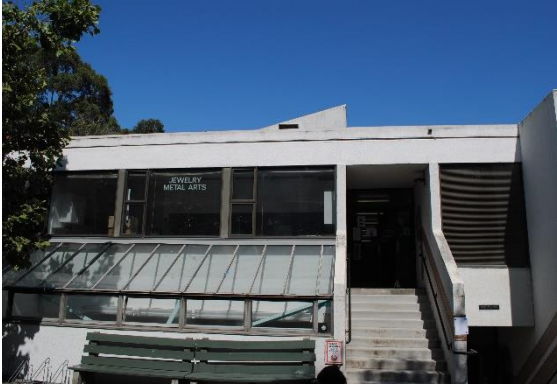
Figure 118. Shaklee Building, east façade, south portion, with primary entrance at right, facing west. Shed roof clerestory volume is partially visible.
