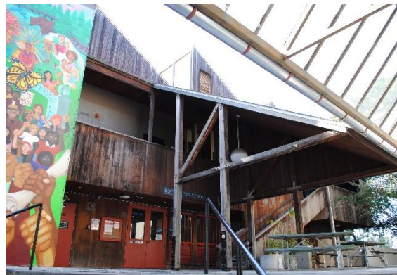
Figure 71. Projecting canopy at primary façade, supported by wood post with one hanging, white globe light fixture, looking southeast.
