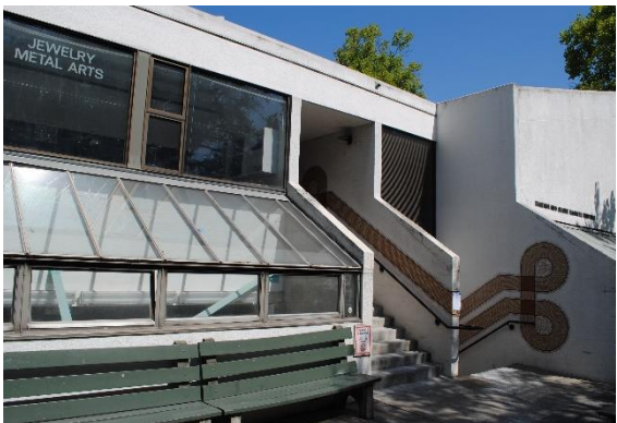
Figure 116. Shaklee Building east façade, center and north portion, facing northwest.
