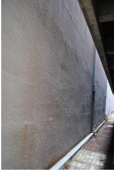
Figure 134. South façade of the Oliver & Ralls Building (left), looking east.
