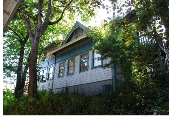
Figure 22. Carriage House, west façade, looking east.
