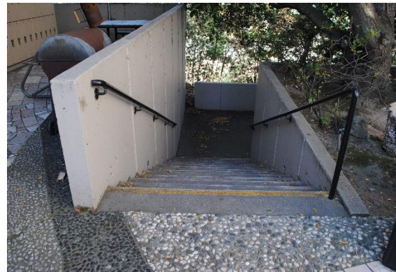
Figure 83. Concrete stairs at the southeast corner of Founders Hall, accessing the south side of the building.
