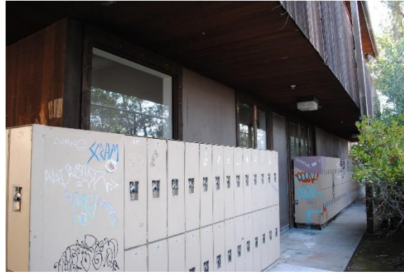
Figure 72. Martinez Hall, south façade, partial view, looking east.
