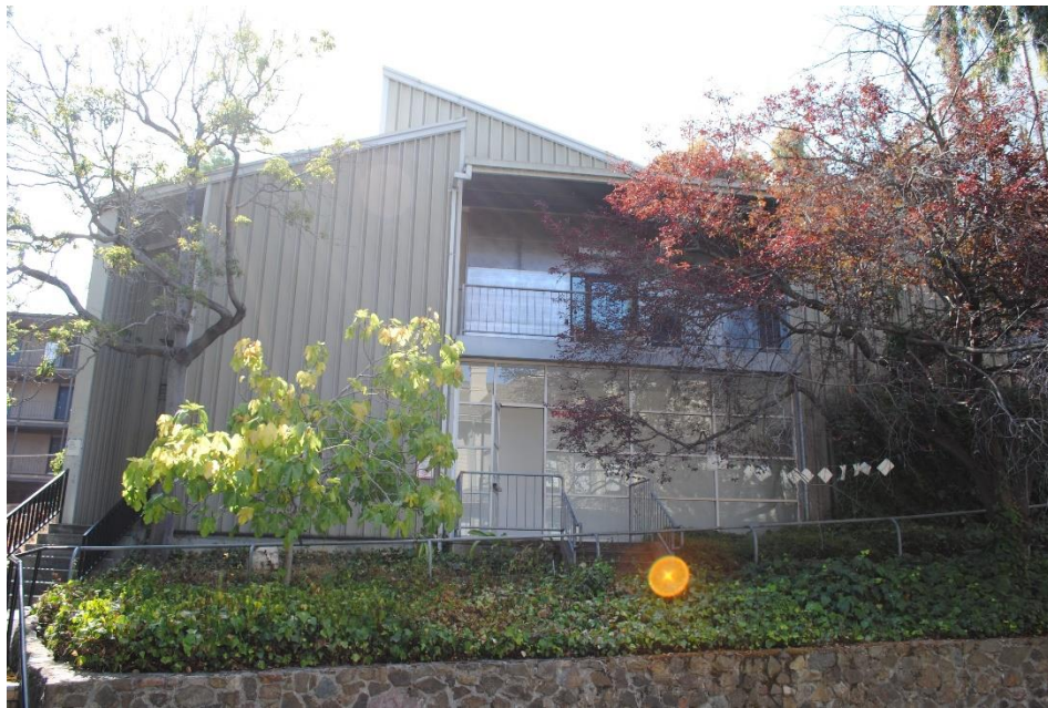
Figure 94. Martinez Hall Annex, primary (west) façade, facing east.
