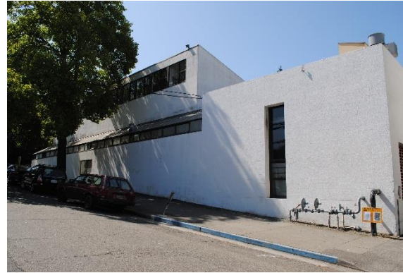
Figure 121. Shaklee Building, north façade, west portion, facing southeast.
