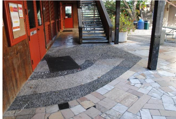
Figure 65. Irregular, polychromatic flagstone and pebble patio between Martinez Hall and Founders Hall, looking south.
