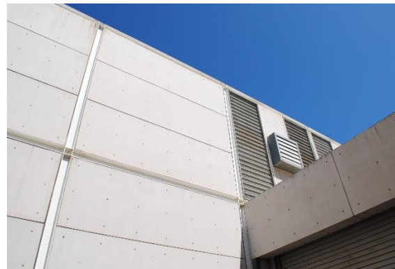
Figure 142. Steel grid structure with fiber-reinforced concrete boards fastened by screws on the east façade, looking west. Metal vents are visible above the central hyphen volume.
