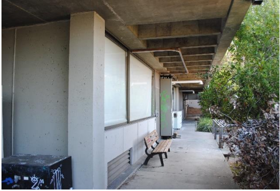
Figure 89. Founders Hall, south façade basement level, facing east.
