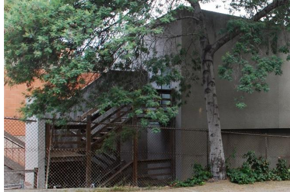
Figure 135. Exterior stair tower at the southeast corner of the Oliver & Ralls Building, accessing doors on the south façade, looking northwest.
