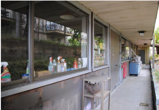
Figure 73. Martinez Hall, east façade, first story, looking north.
