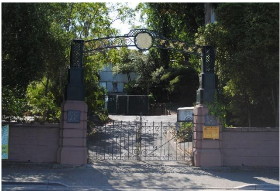
Figure 31. Broadway Wall carriage entrance with plaques and metal arch, looking east.
