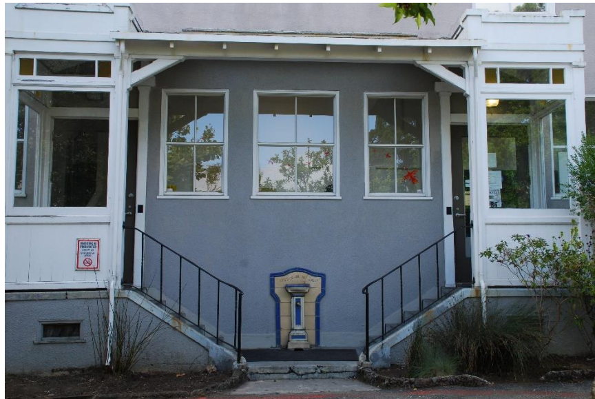
Figure 44. The B Building, west façade detail, primary entrances and tile fountain, facing east.
