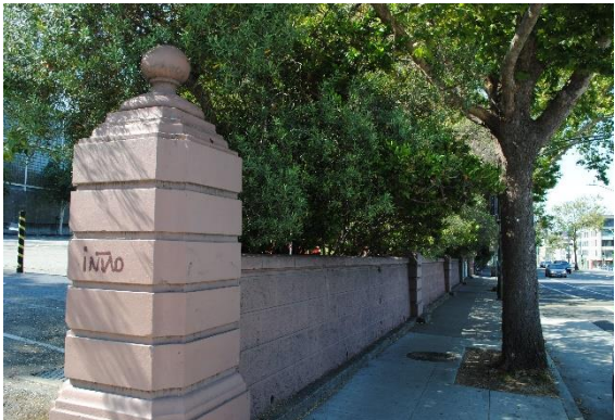
Figure 27. Broadway Wall, northernmost pier, facing southeast.
