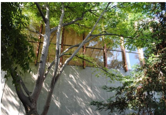
Figure 86. Founders Hall, north façade, second story detail, facing southwest.
