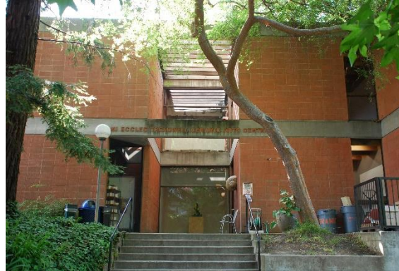
Figure 100. Ceramic Arts Center, recessed entry accessed via concrete steps at the primary (west) façade, facing east.
