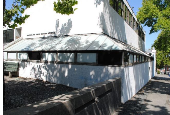
Figure 119. Conservatory windows at the north portion of the primary façade.
