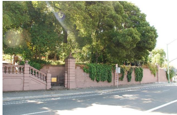
Figure 28. Broadway Wall, southernmost three piers, facing southeast.
