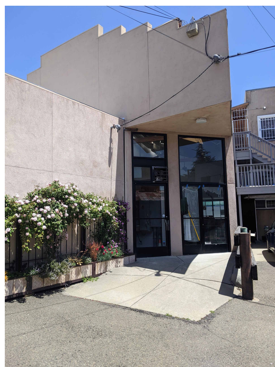
SUBJECT PROPERTY REAR FACADE
