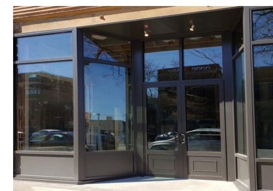
STOREFRONT SYSTEM - CLR. TEMP GL. IN BRONZE ANODIZED ALUM. FRAME
