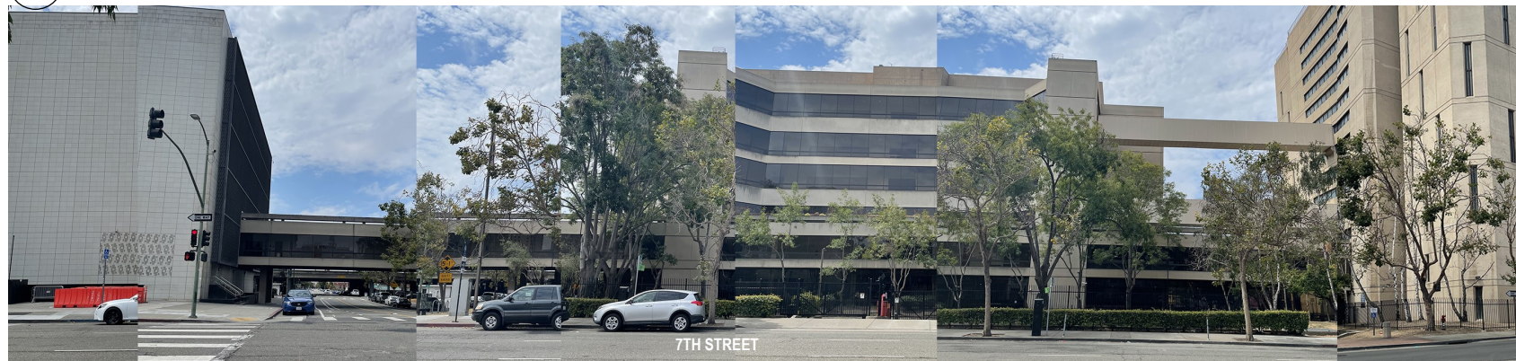
4 BUILDINGS ACROSS THE STREET ON WASHINGTON STREET (FACING SOUTH)
