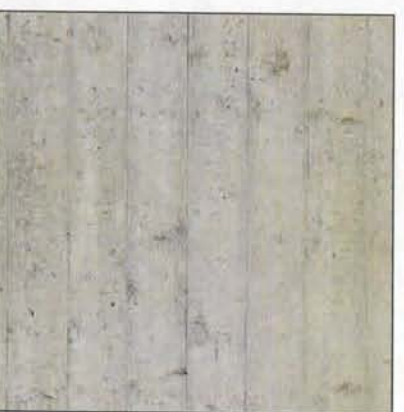
BOARD FORM CONCRETE
