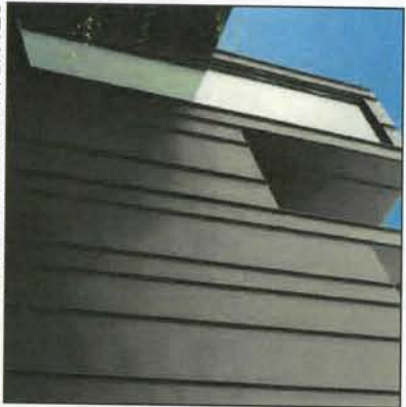
STANDING SEAM SIDING/ CORRUGATED METAL SIDING
