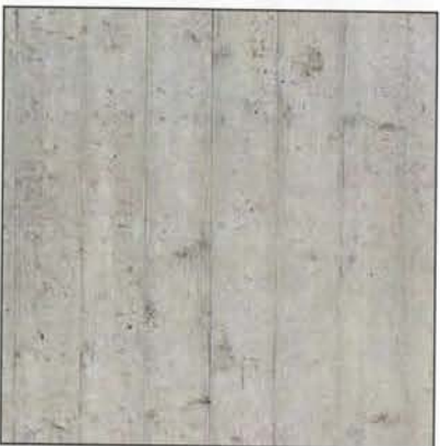
BOARD FORM CONCRETE
