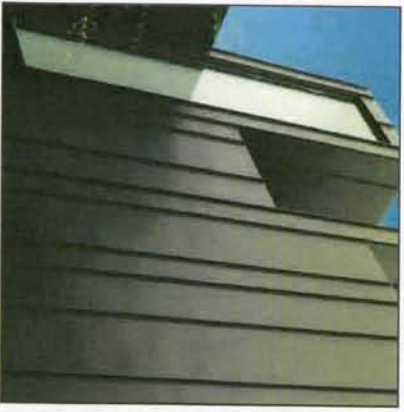
STANDING SEAM SIDING/ CORRUGATED METAL SIDING
