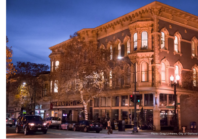
Photo 20- Streetscape in Old Oakland
