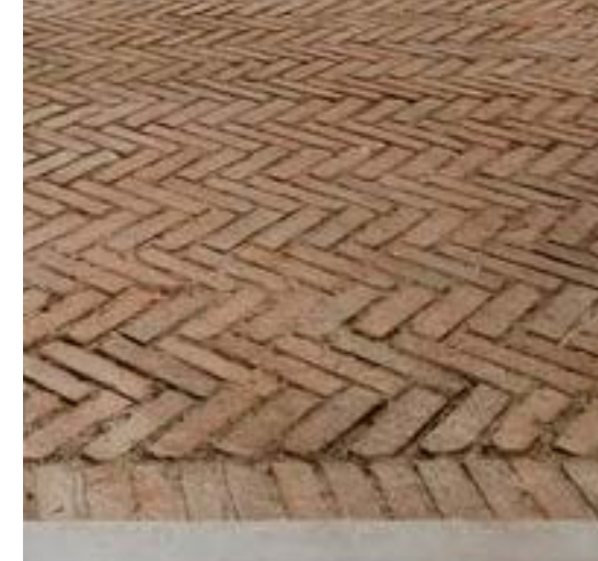
4. Site Salvaged Brick Paving
