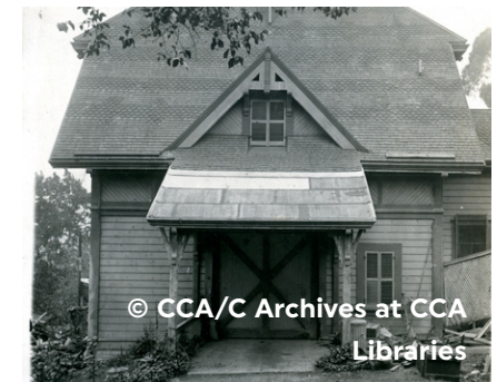
Figure 2.7: Carriage House original opening on east facade
