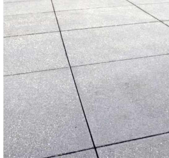
3. CIP Concrete Paving - Finish 3 Pedestrian
