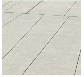
1. CIP Concrete Paving - Finish 1 Manufacturer: Davis Colors Color: Sandstone 5237 Finish: Top-Cast Sawcut control joints
