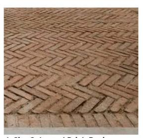
4. Site Salvaged Brick Paving Existing bricks to stockpile and protect onsite Approximate Size: 4-1/2" X 9" XD 2-1/2"
