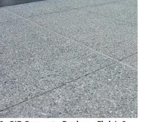
2. CIP Concrete Paving - Finish 2 Manufacturer: Davis Colors Color: Sandstone 5237 Finish: Heavy Top-Cast Sawcut control joints
