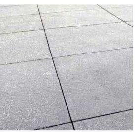
3. CIP Concrete Paving - Finish 3 **Pedestrian**
