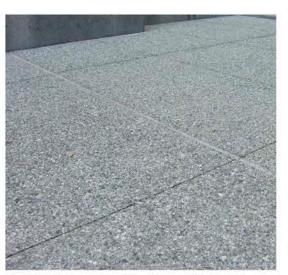
2. CIP Concrete Paving - Finish 2 Pedestrian and Vehicular
