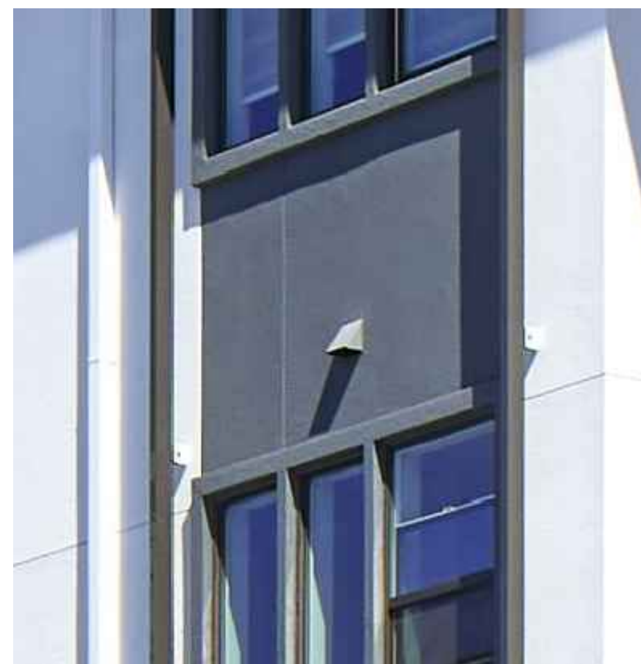
TYP. VENT DETAIL (PAINT TO MATCH ADJACENT COLOR) (LOCATIONS TBD DURING CD PHASE)
