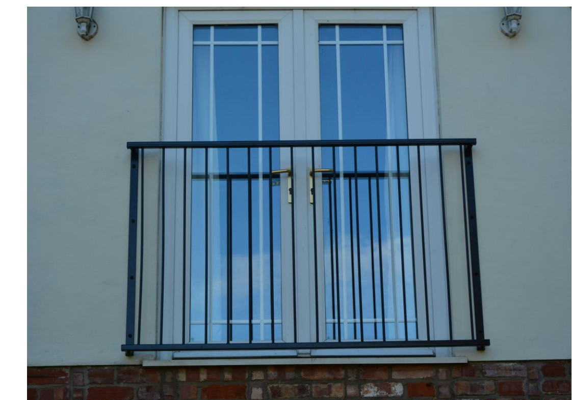
METAL JULIET BALCONY RAILING
