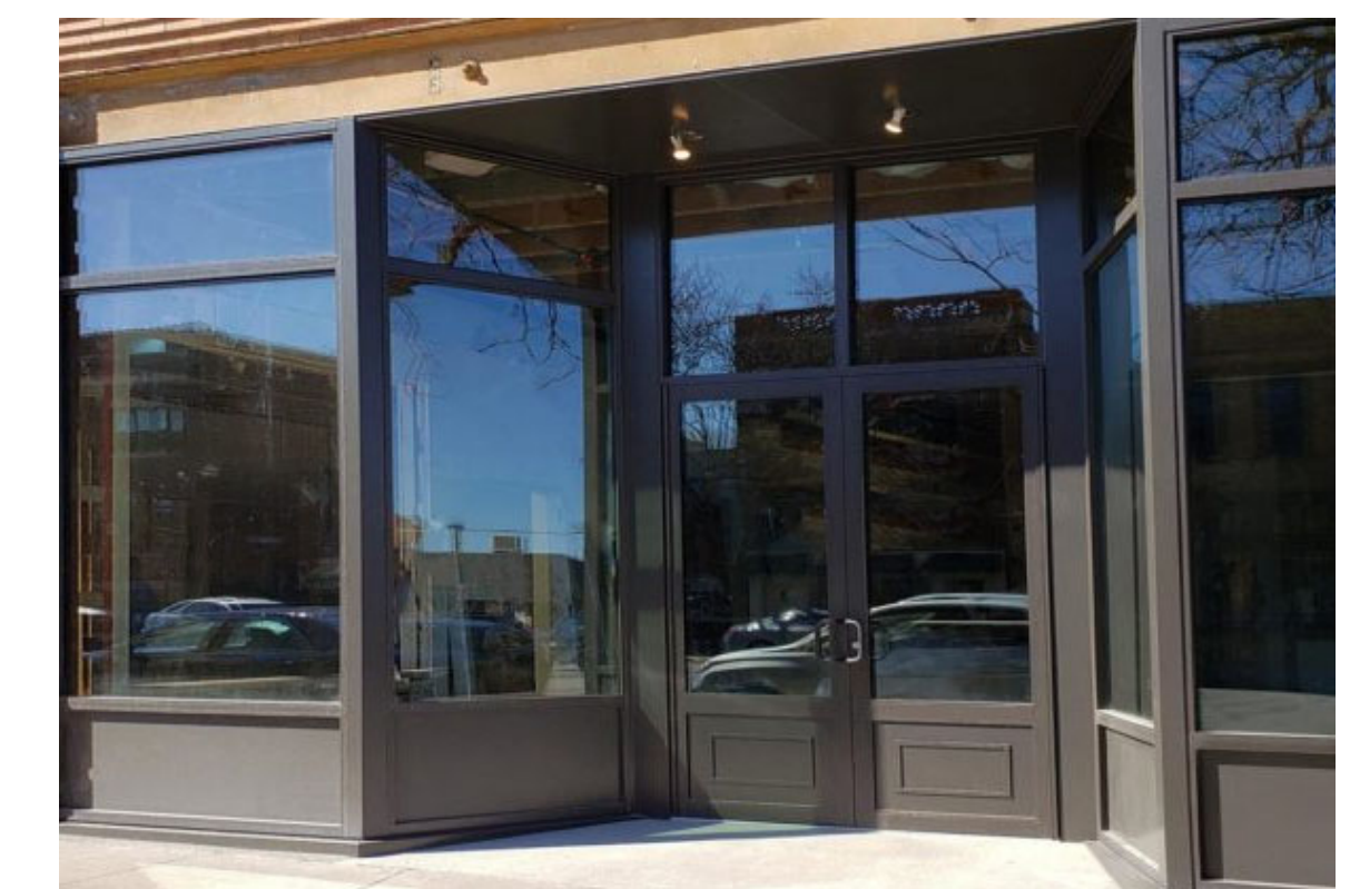
STOREFRONT SYSTEM - CLR. TEMP GL. IN BRONZE ANODIZED ALUM. FRAME
