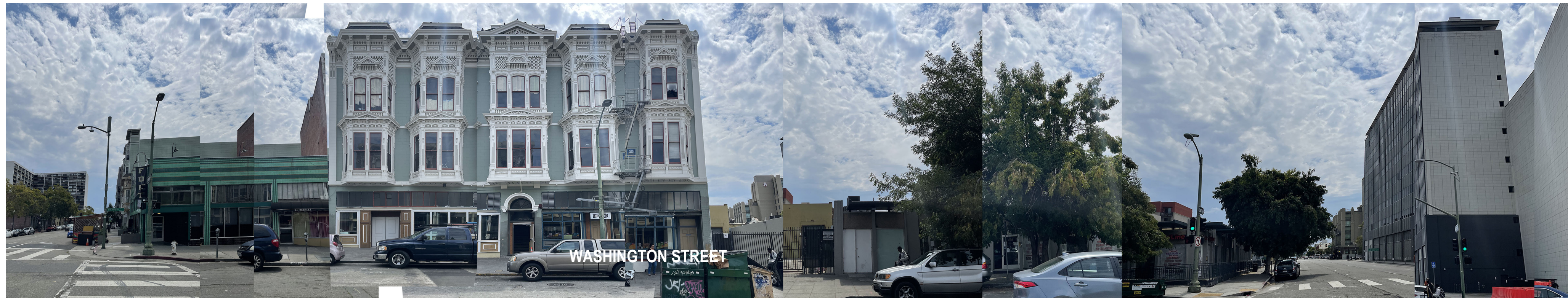
2 BUILDINGS ACROSS THE STREET ON WASHINGTON STREET (FACING EAST)
