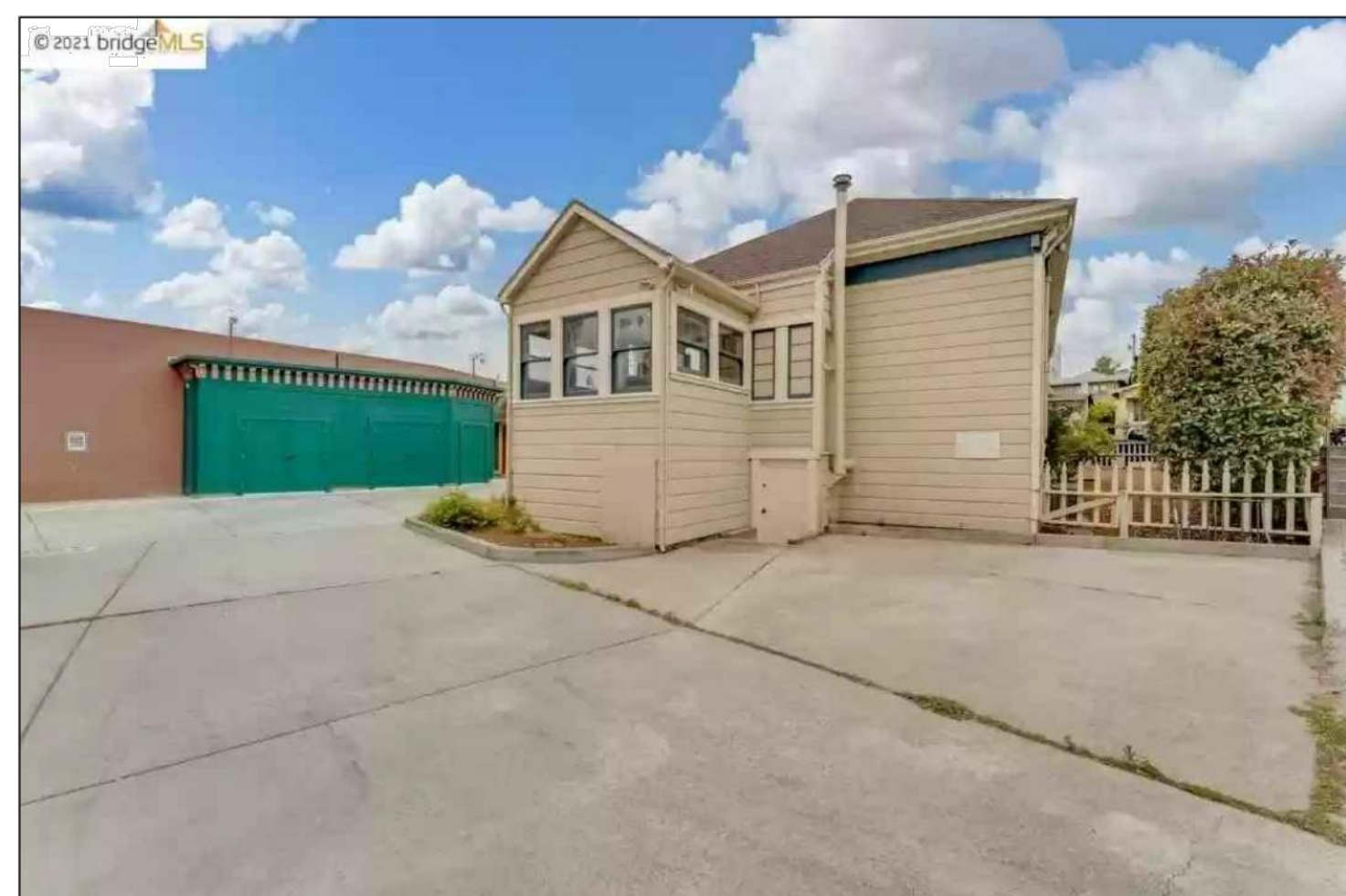
SOUTH EAST CORNER
