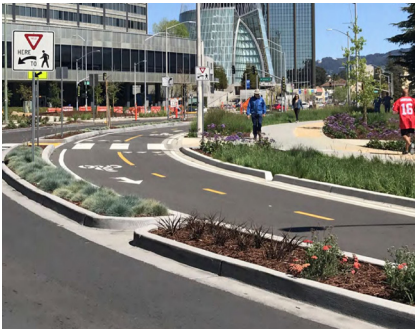
Harrison Street Bioswales (Source: Oakland GSI Plan)
