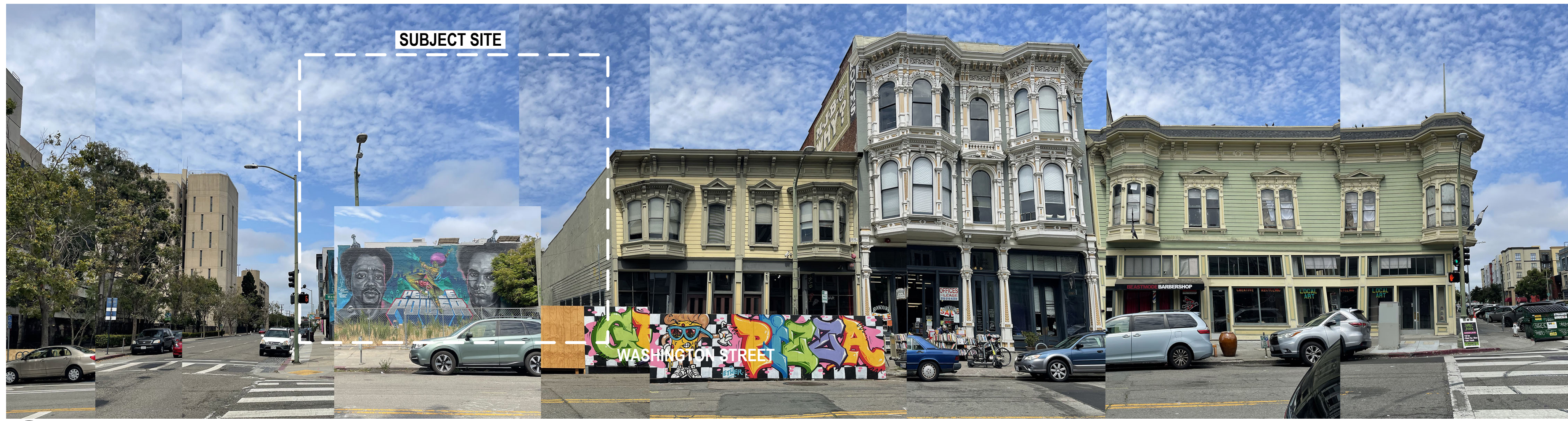
1 SUBJECT SITE AND ADJACENT BUILDINGS ON WASHINGTON STREET (LOOKING WEST)
