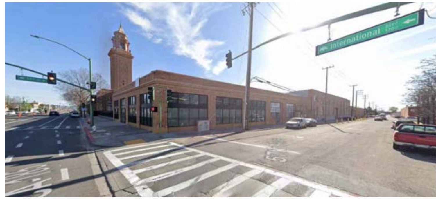
5701 INTERNATIONAL BLVD., BUILDING A
