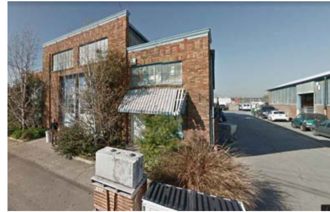
1135 57TH AVE. (NORTH)
