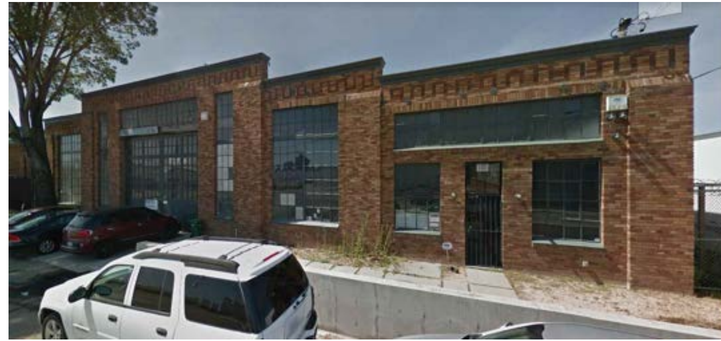
1137 57TH AVE., CONCRETEWORKS (NORTH)
